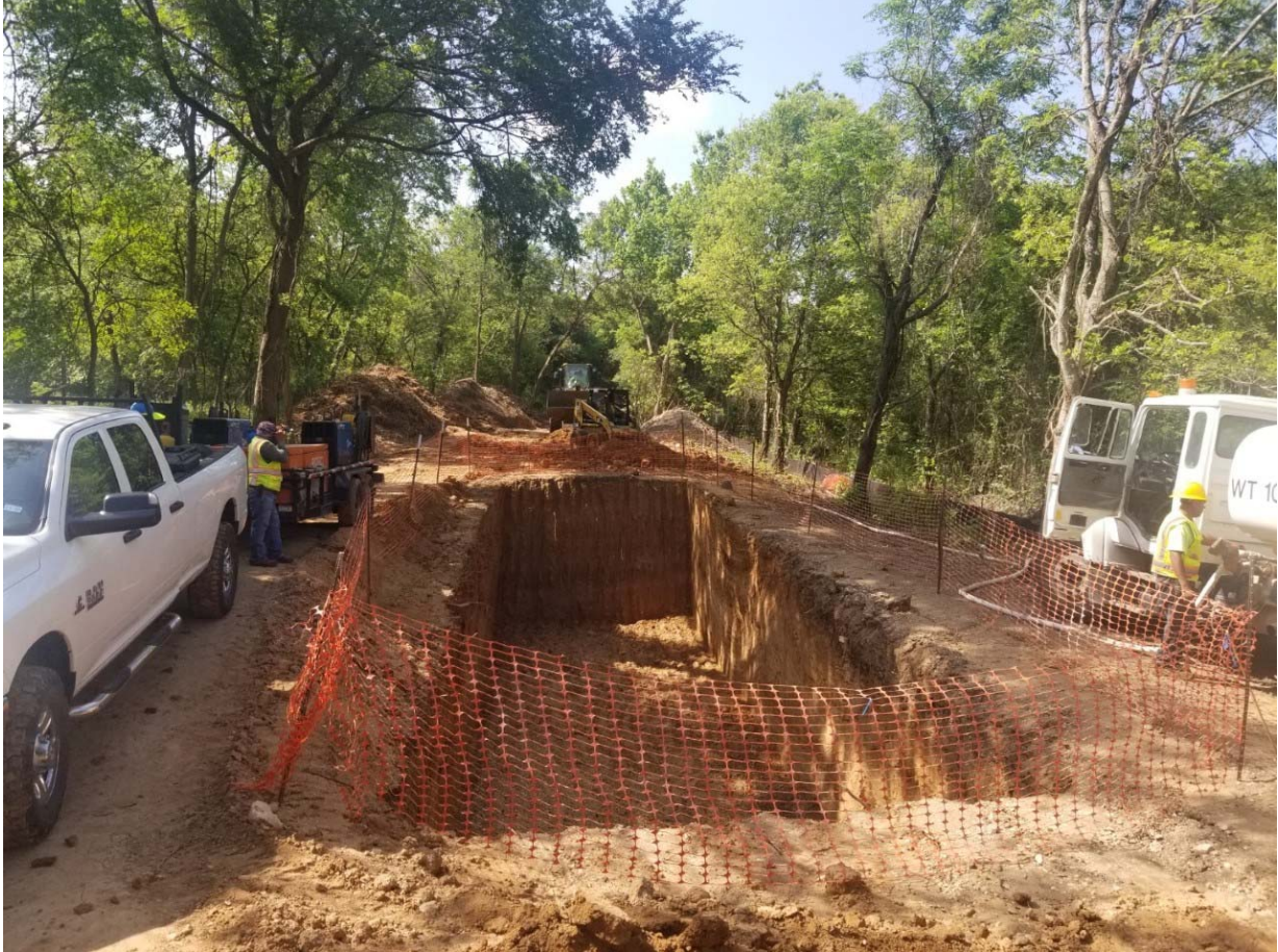
Bore Pit Prep – Southside of Onion Creek crossing.
