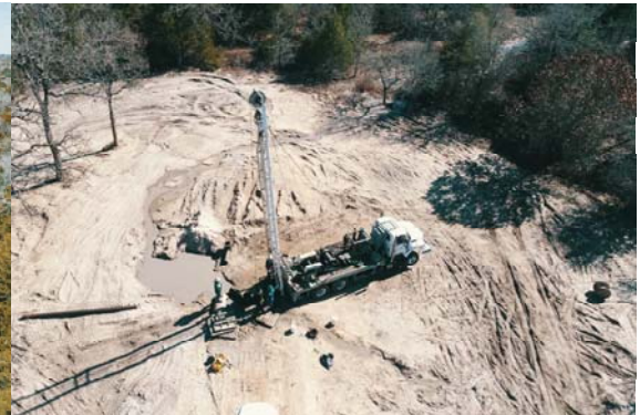
Well No. 9 Bailing to Cleanup Water
