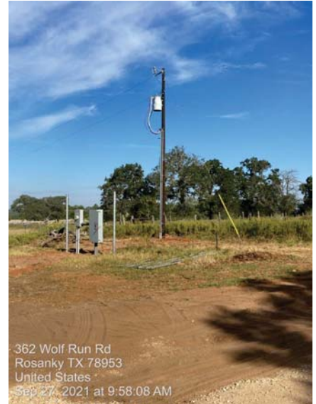
Electrical service for job trailers
