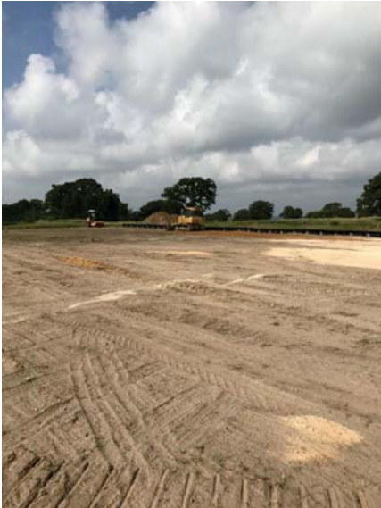
Placing base at laydown yard
