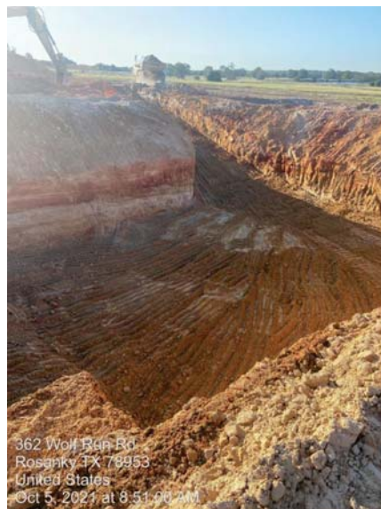
Plate settler basin subgrade
