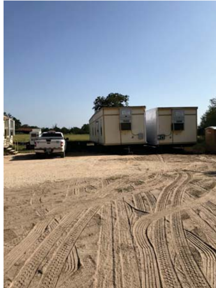
Job trailers delivered
