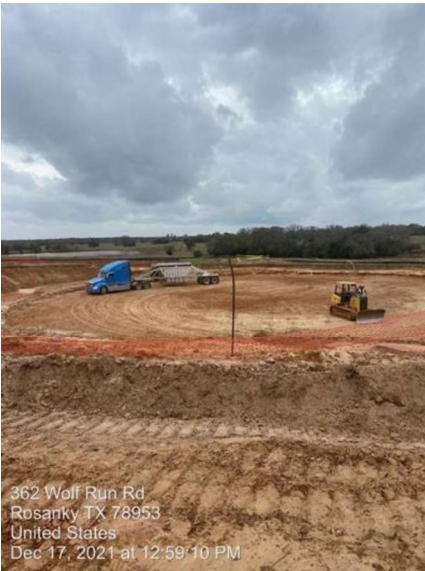
WTP/RWI – Clearwell backfill
