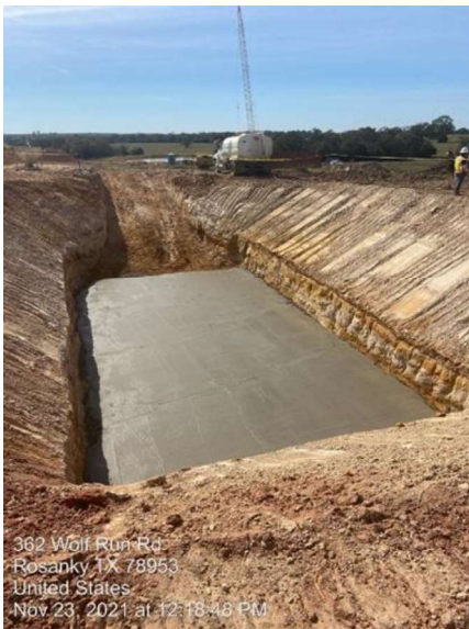
WTP/RWI – Rapid Mix Basin mud slab
