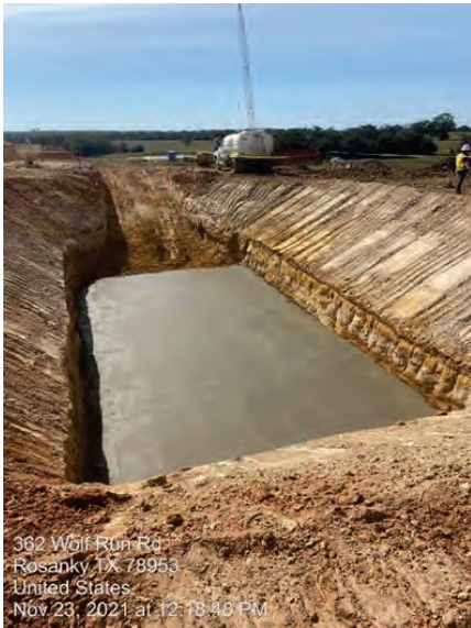
WTP/RWI – Rapid Mix Basin mud slab
