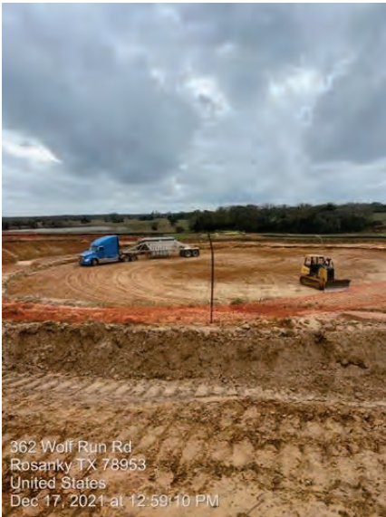
WTP/RWI – Clearwell backfill
