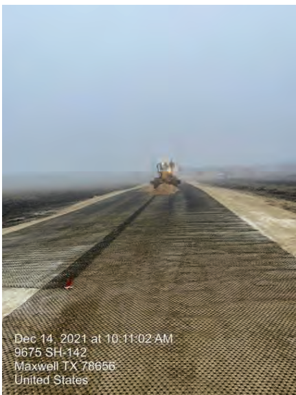
BPS - Access Road construction
