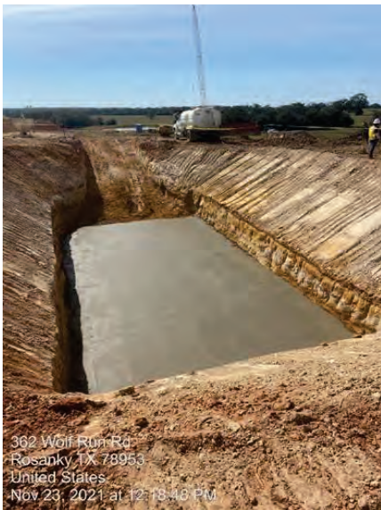
WTP/RWI – Rapid Mix Basin mud slab
