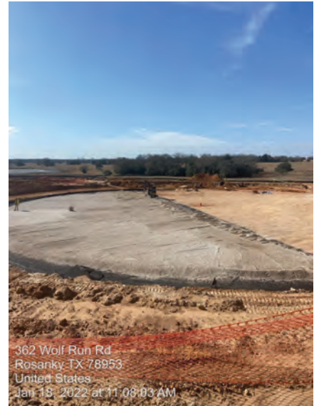
WTP/RWI – Clearwell Leveling Base
