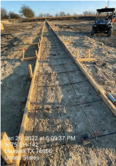
BPS – Detention Pond Trickle Channel
