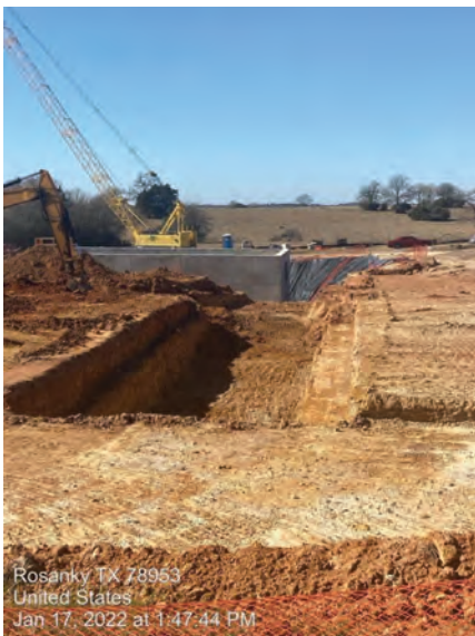
WTP/RWI – Filter Complex Excavation
