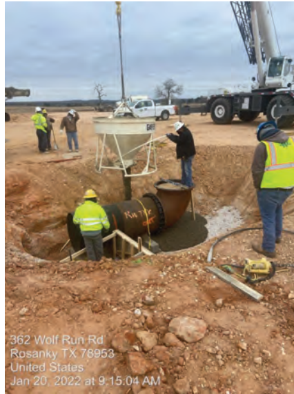
WTP/RWI – Tank Piping Encasement
