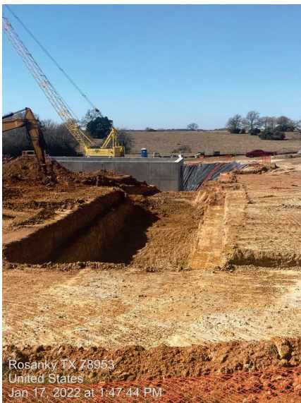
WTP/RWI – Filter Complex Excavation
