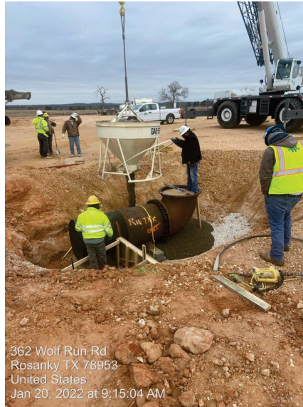
WTP/RWI – Tank Piping Encasement
