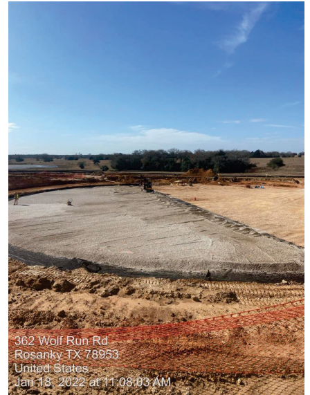
WTP/RWI – Clearwell Leveling Base
