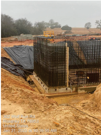
WTP/RWI – Recycle Pump Station
