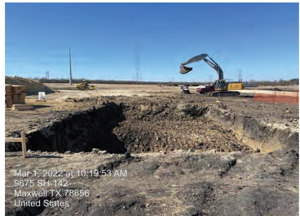
BPS – Electrical Building Foundation Excavation
