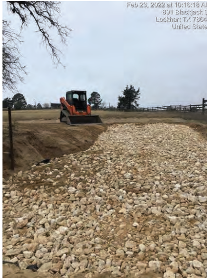
Seg A – Construction Entrance
