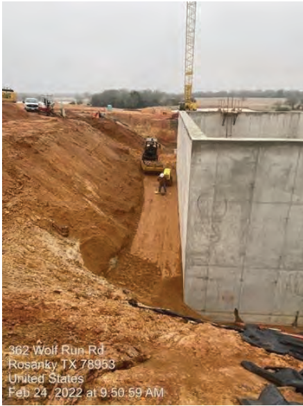
WTP/RWI – Flow EQ Basin Backfill
