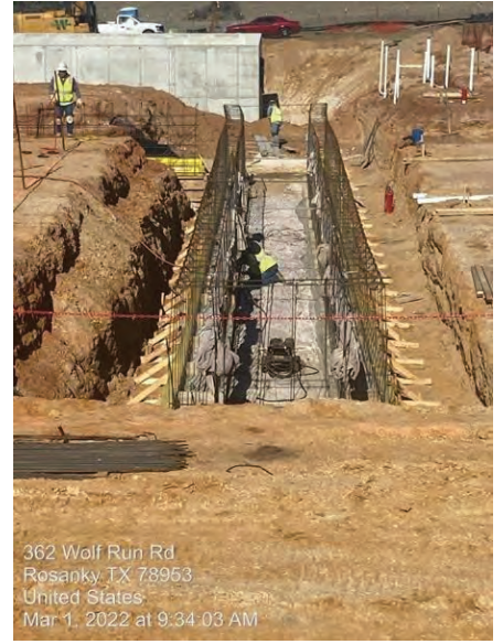
WTP/RWI – Filter Complex BWW piping trench
