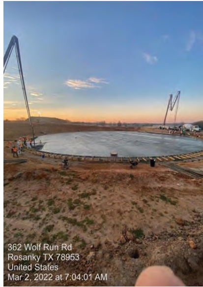
WTP/RWI – Clearwell Foundation Slab
