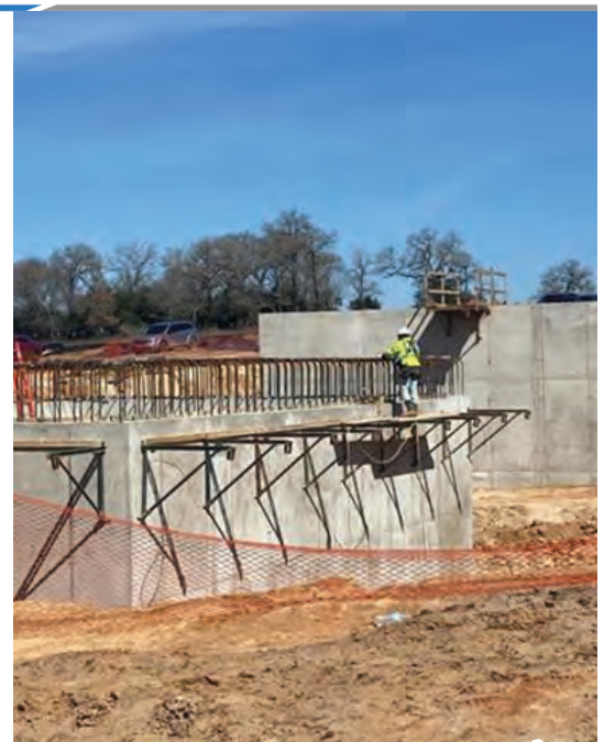
Recycle Pump Station roof deck forming
