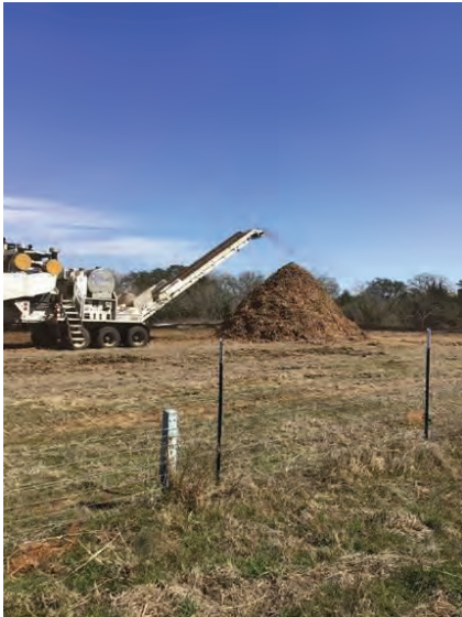
Seg A – Clearing and Mulching ROW
