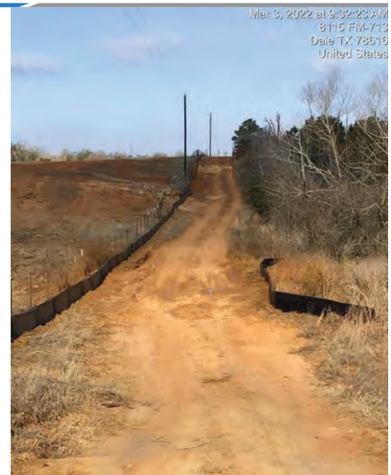
Seg A – Silt Fence Installation
