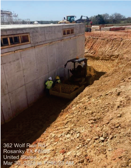
WTP/RWI – Recycle Pump Station Backfill
