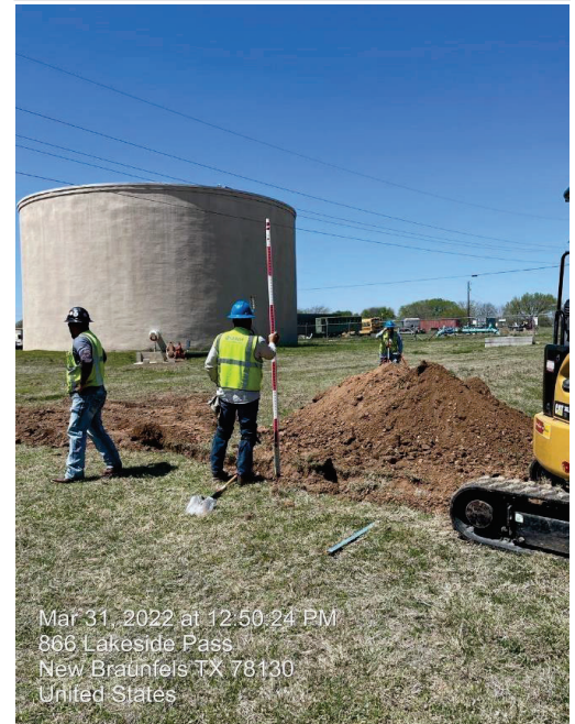
CRWA #4 Delivery Point potholing
