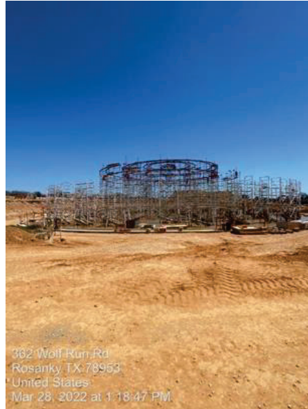
WTP/RWI – Clearwell Roof Shoring
