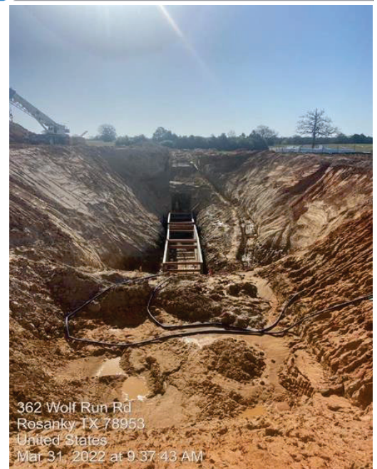
High Service Pump Station Excavation/Shoring
