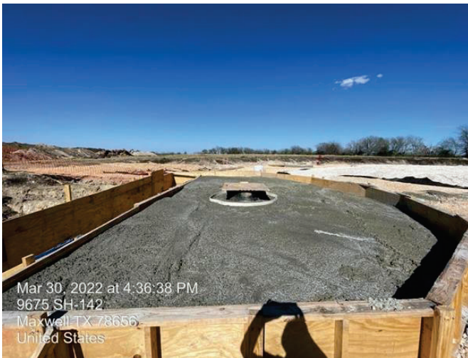
BPS – GST 36" DIP outlet concrete encasement
