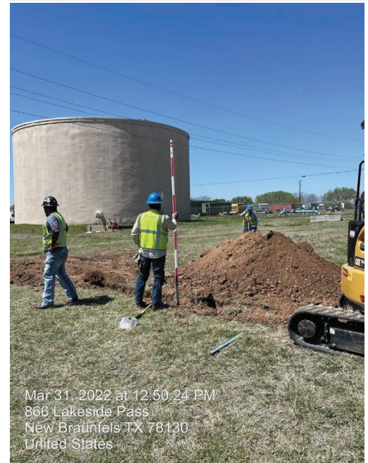
CRWA #4 Delivery Point potholing
