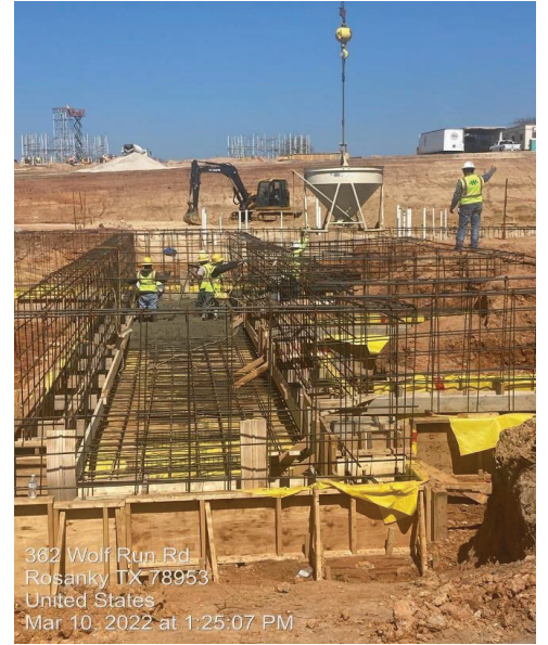
WTP/RWI – Filter Complex BWW piping trench
