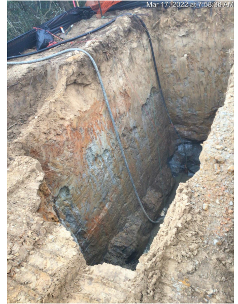
Seg A – Bore Pit at Sandy Creek 11
