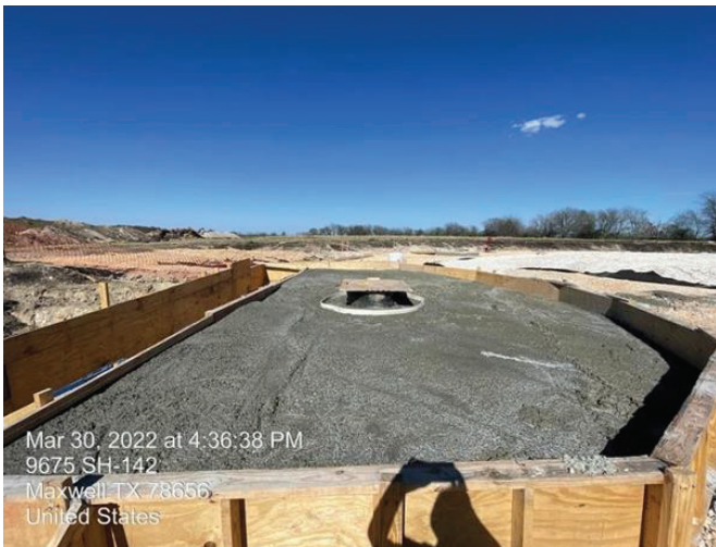
BPS – GST 36" DIP outlet concrete encasement
