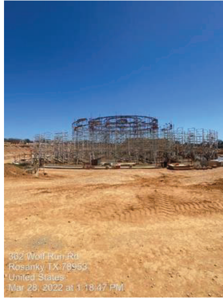
WTP/RWI – Clearwell Roof Shoring
