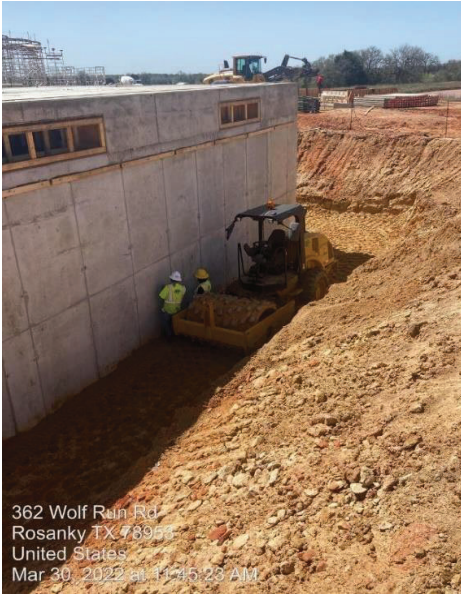
WTP/RWI – Recycle Pump Station Backfill
