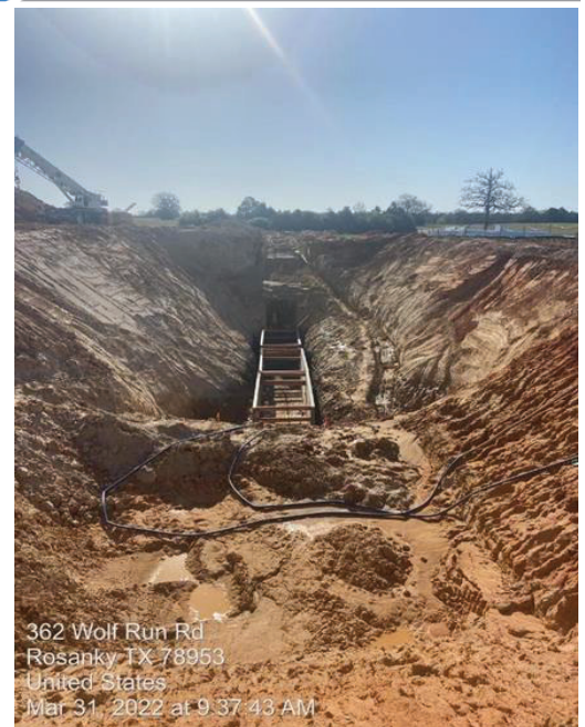
High Service Pump Station Excavation/Shoring
