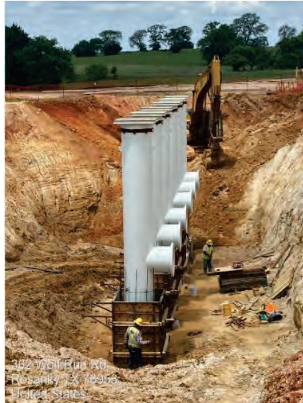
WTP– HSPS Pump Can Installation
