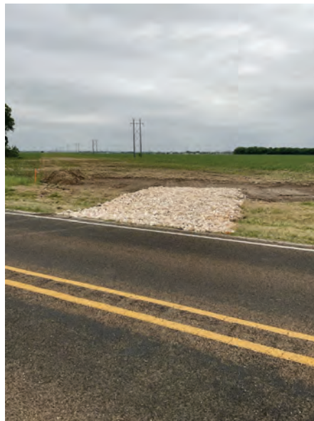
Seg B – Construction Entrance Installation
