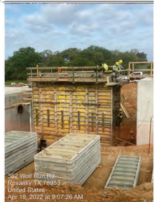
Basin Wall Forms East Side
