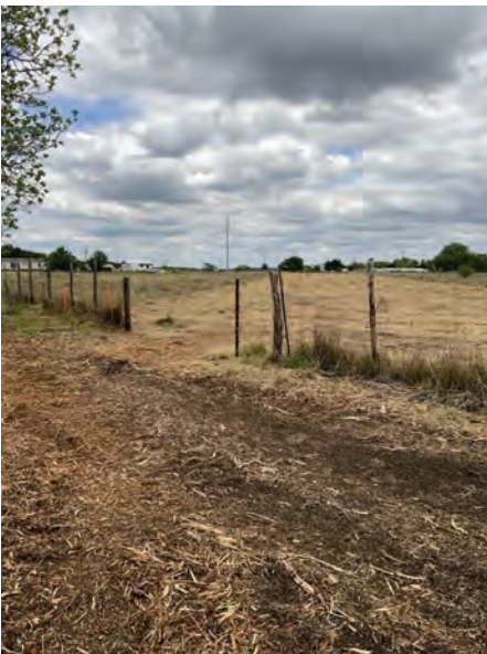
Seg B – Fence Gap Installation
