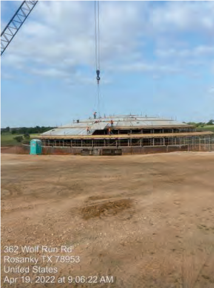
WTP – Placing Clearwell Roof Panels
