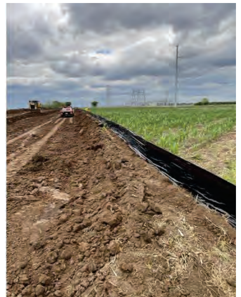
Seg B –Topsoil Removal
