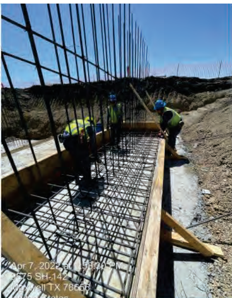
BPS – Steel Reinforcement for Pump Station
