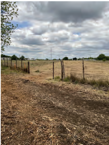
Seg B – Fence Gap Installation
