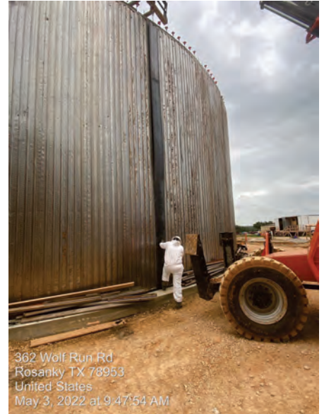
WTP – Raw Water Tank Wall Panel Joint Installation
