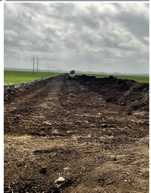
Seg B – Topsoil Stripping
