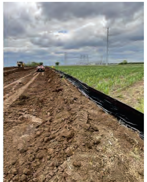
Seg B –Topsoil Removal
