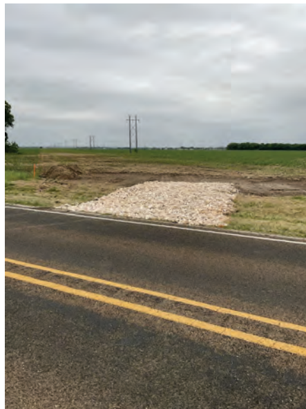
Seg B – Construction Entrance Installation
