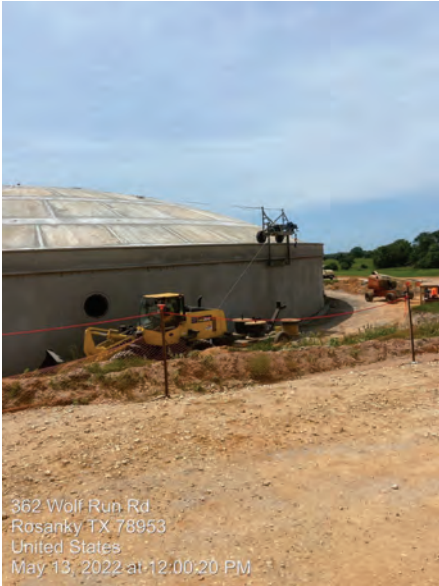
WTP – Cable install on top dome ring at Clearwell
