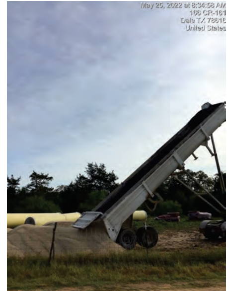
Seg A – Embedment material delivery to site
