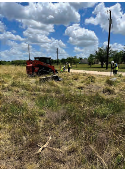
Seg B – Fence gap installation
