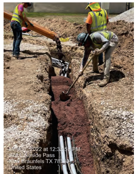
BPS – Concrete placement for electrical duct bank at CRWA #4
