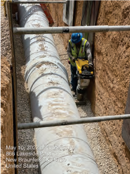
BPS – Embedment compaction for 36” DI at CRWA #4
