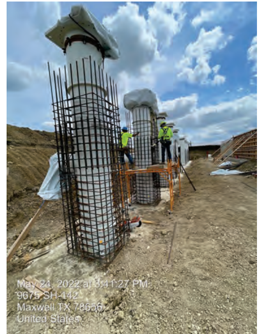
Reinforced steel for pump cans
