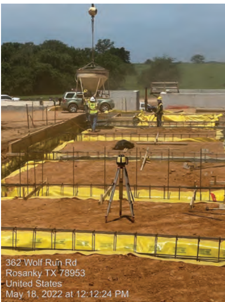
WTP – Placing concrete at grade beams at filter complex
