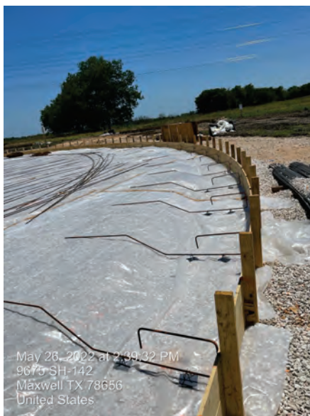
BPS – Reinforcement steel for GST
