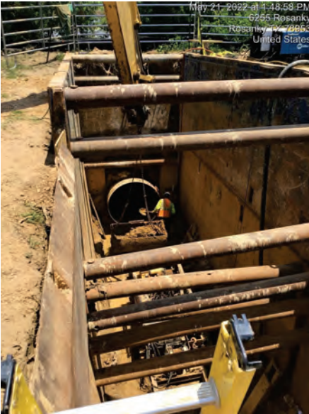
Seg A – Boring operations at Bore #2 (Wetlands Crossing)
