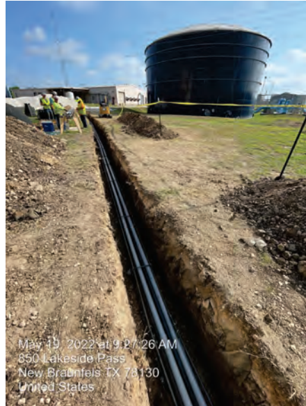
BPS – Electrical duct bank installation at CRWA #4
