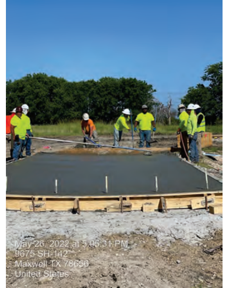
BPS – Wall section concrete placement for GST
