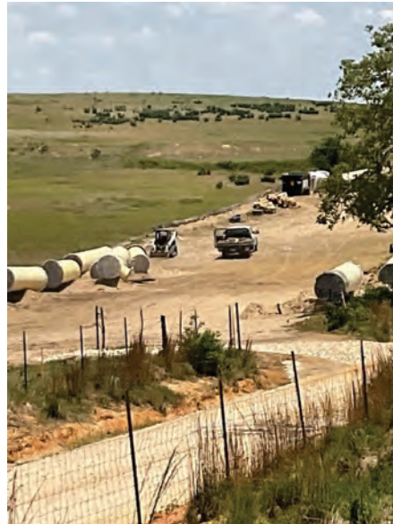
Seg A – Cleared ROW and pipe staging
