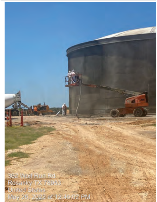
Placing shotcrete at Raw Water Storage Tank
