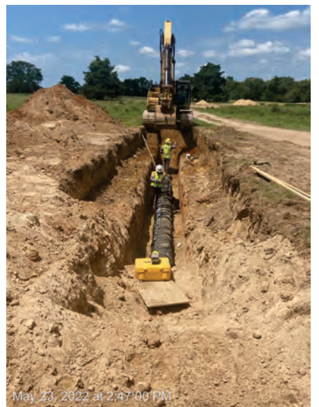
WTP – Raw Water Pipeline WL-A
