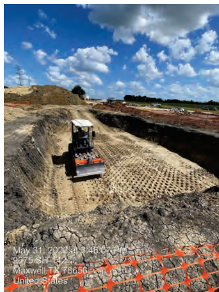
BPS – Generator pad subgrade preparation
