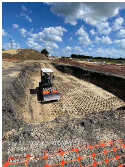
BPS – Generator pad subgrade preparation
