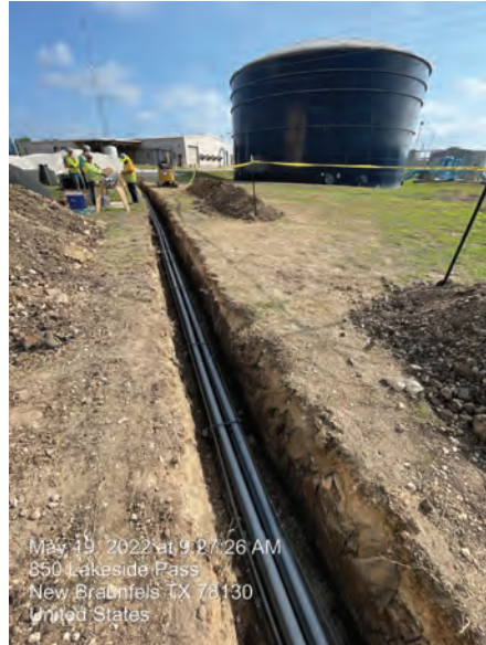
BPS – Electrical duct bank installation at CRWA #4
