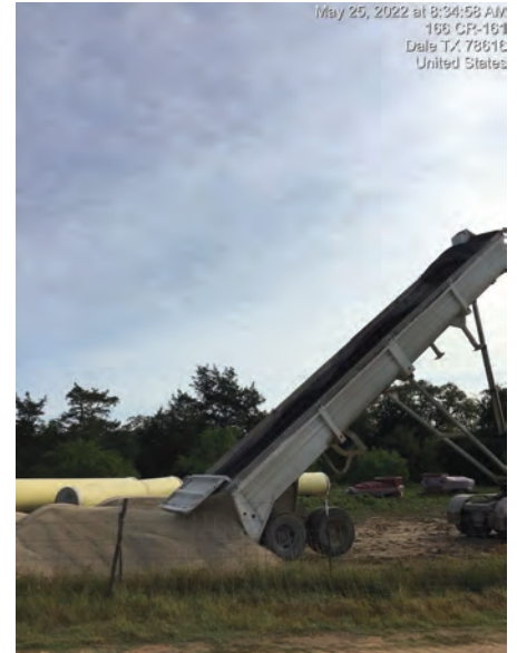
Seg A – Embedment material delivery to site
