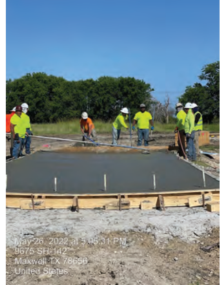
BPS – Wall section concrete placement for GST
