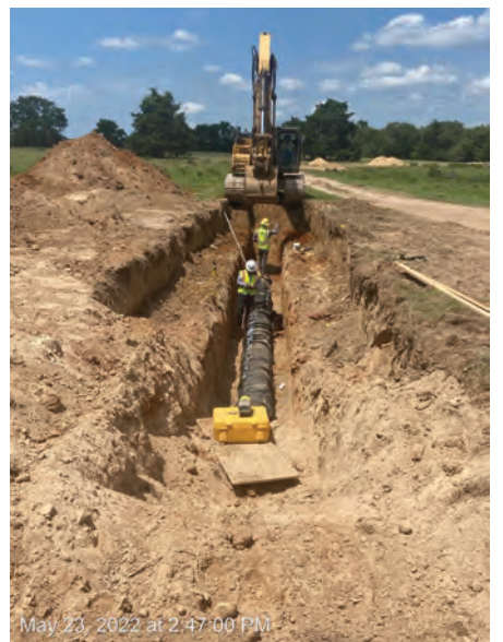
WTP – Raw Water Pipeline WL-A
