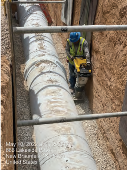
BPS – Embedment compaction for 36” DI at CRWA #4
