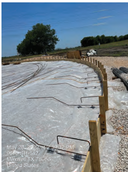
BPS – Reinforcement steel for GST
