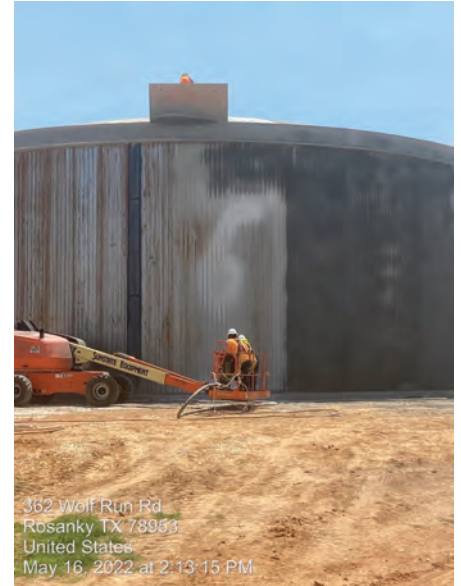
WTP – Placing shotcrete at Raw Water Storage Tank
