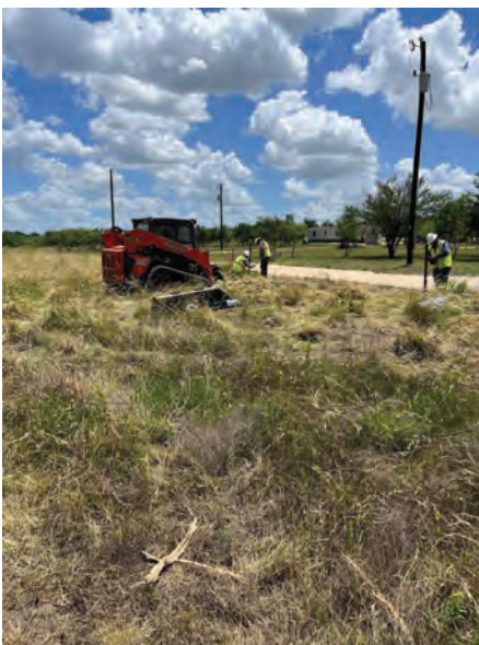
Seg B – Fence gap installation
