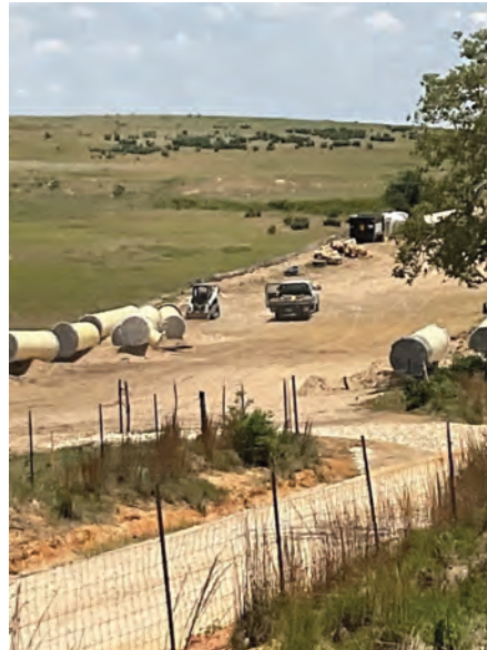
Seg A – Cleared ROW and pipe staging
