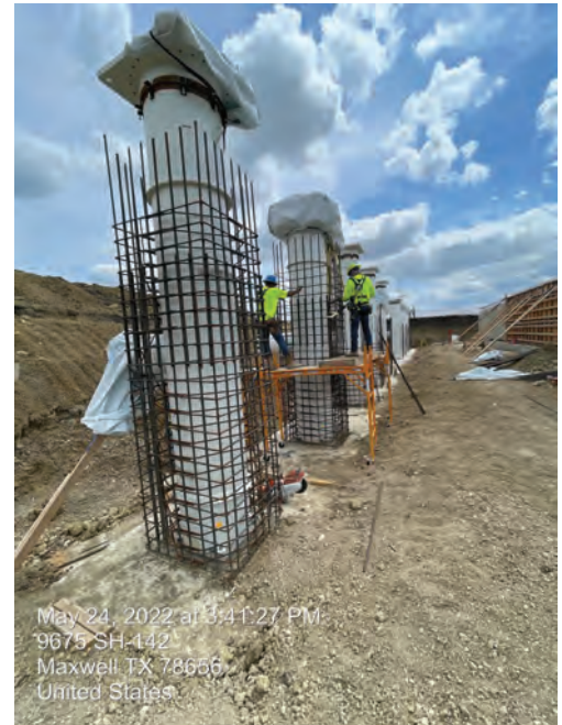
Reinforced steel for pump cans
