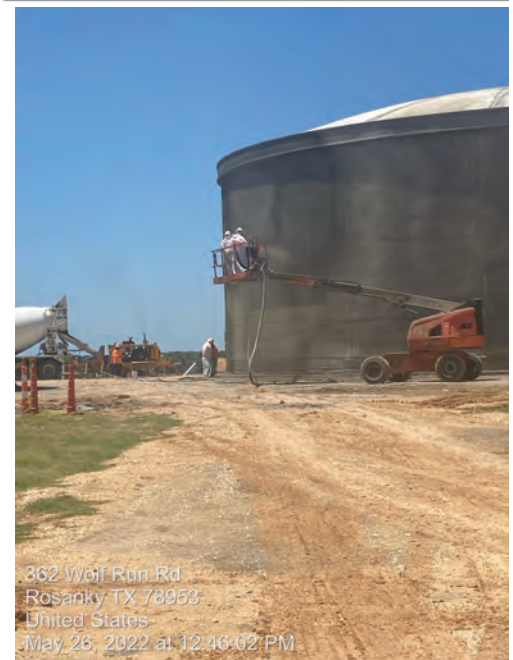
Placing shotcrete at Raw Water Storage Tank
