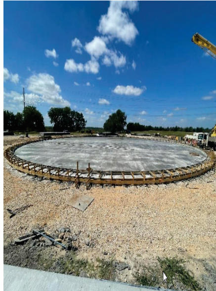
BPS – GST Foundation Slab
