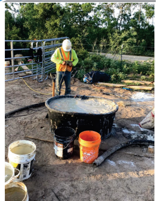
Seg A – Mixing Gel at Bore No. 2
