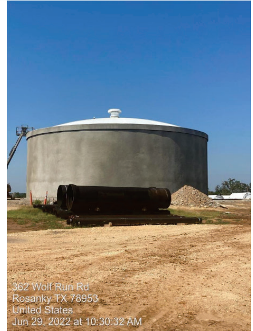
Raw Water Tank Dome and Vent
