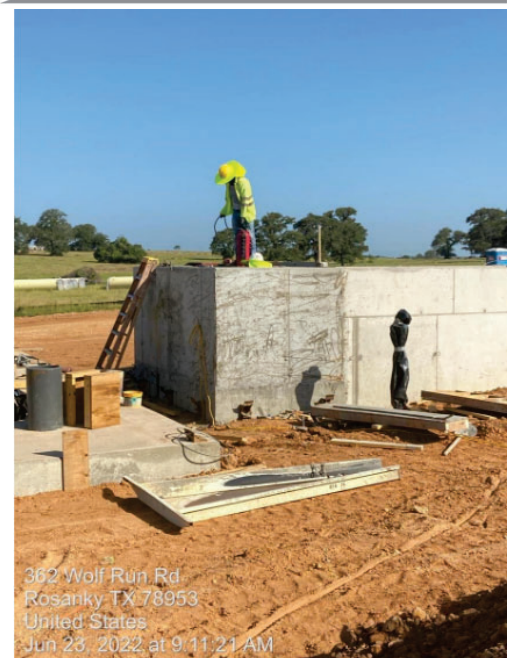
Plate Settler Basin Outlet Box
