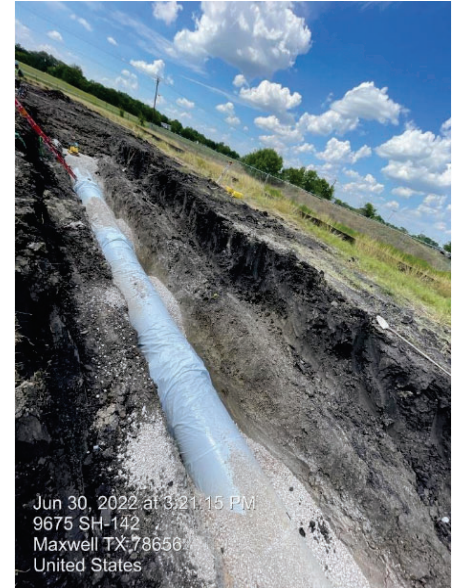
BPS – Installation of 36" DIP Seg B at STA 4+50
