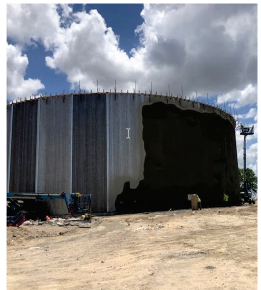
GST Wall Panel Erection
