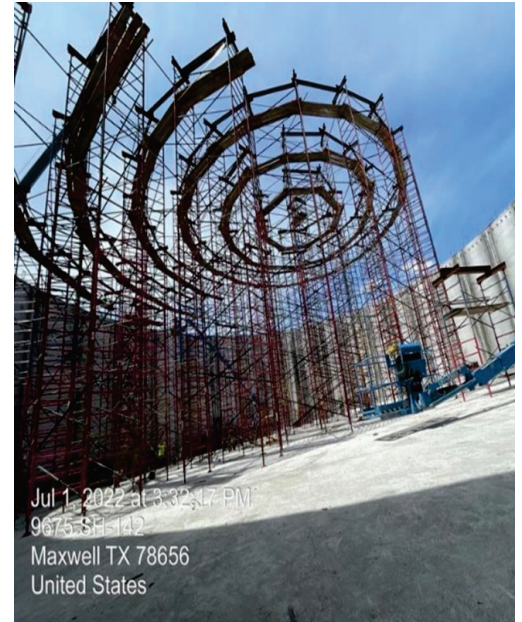
GST Roof Dome Shoring Erection
