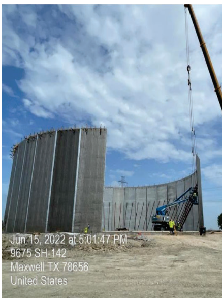
BPS – GST Wall Panel Erection
