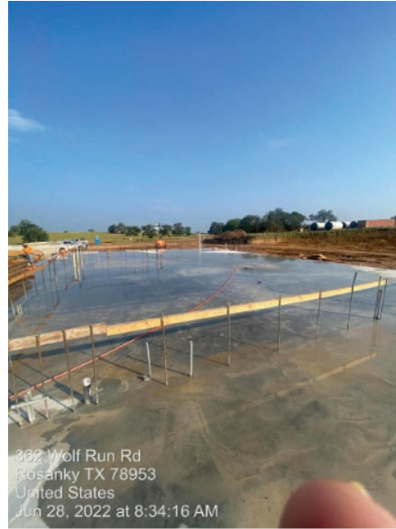
WTP– Maintenance Room Slab of Filter Complex
