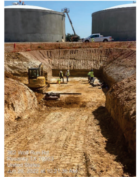
WTP – Drain Line Installation at Rapid Mix Basin
