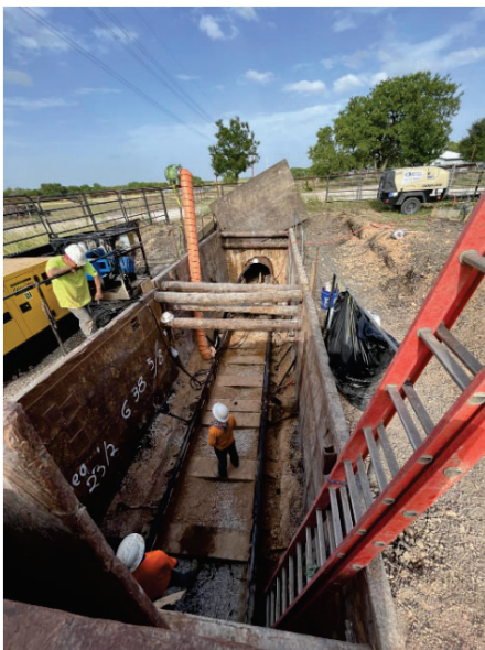
Seg B2 – BORECO Tunnel at CR 173
