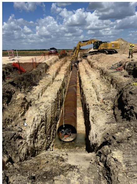
Seg B – Casing Placement at FM 110
