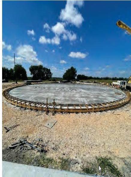
BPS – GST Foundation Slab
