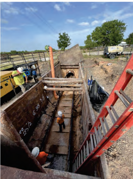
Seg B2 – BORECO Tunnel at CR 173
