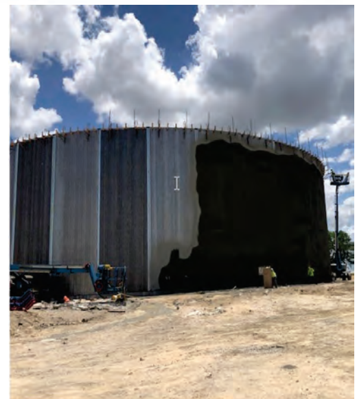
GST Wall Panel Erection
