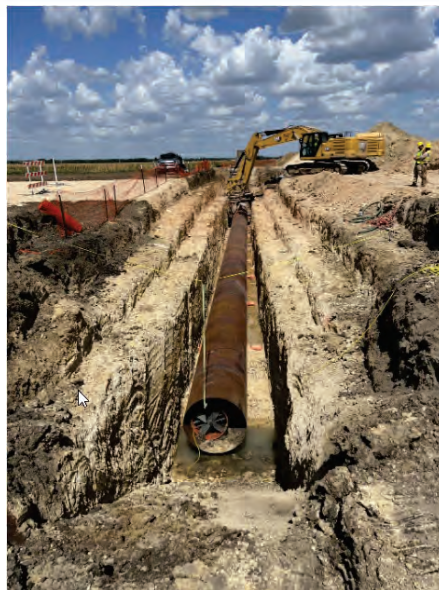
Seg B – Casing Placement at FM 110
