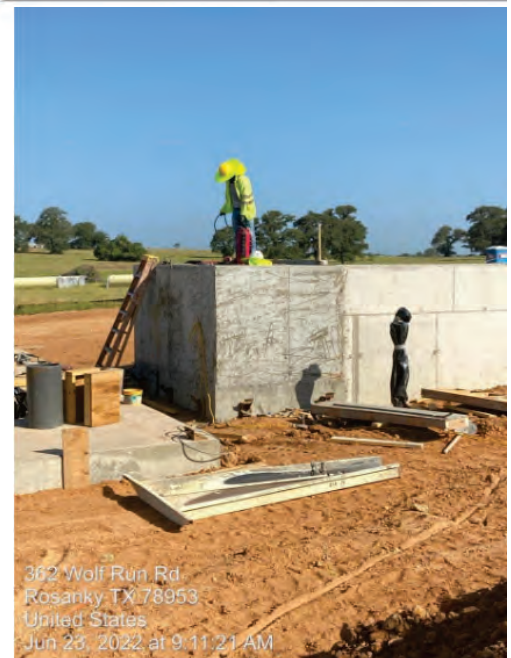
Plate Settler Basin Outlet Box
