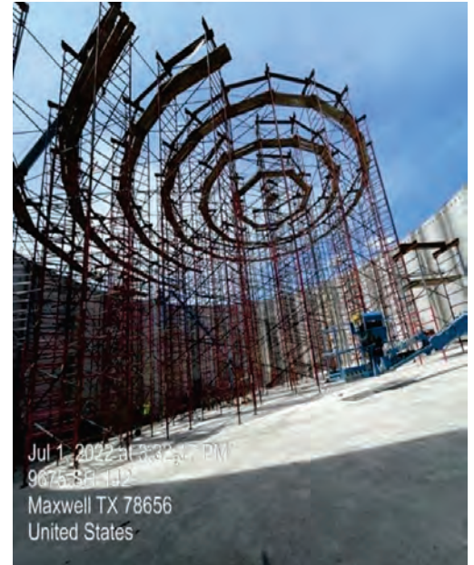
GST Roof Dome Shoring Erection
