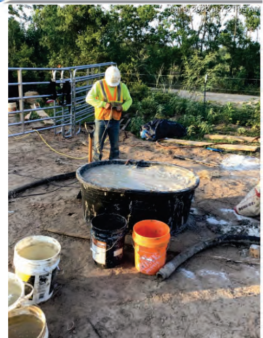
Seg A – Mixing Gel at Bore No. 2
