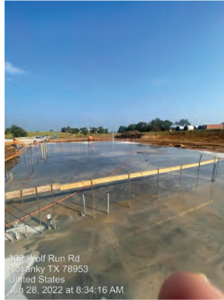
WTP– Maintenance Room Slab of Filter Complex
