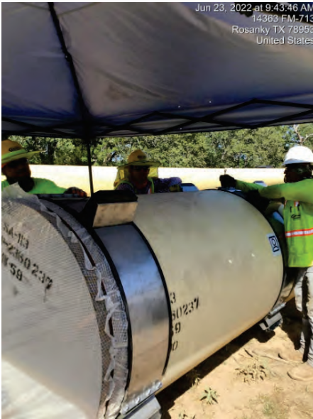
Seg A – Placing Case Spacers on Bore No. 1
