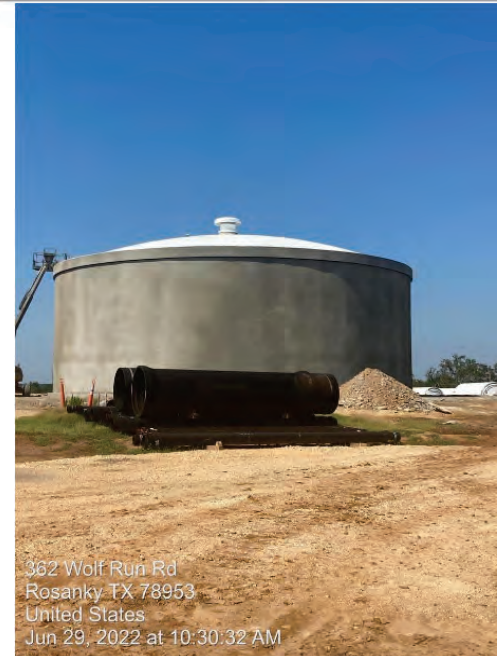
Raw Water Tank Dome and Vent
