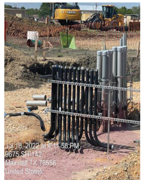
BPS – Electrical Building Electrical Conduit Rough-in
