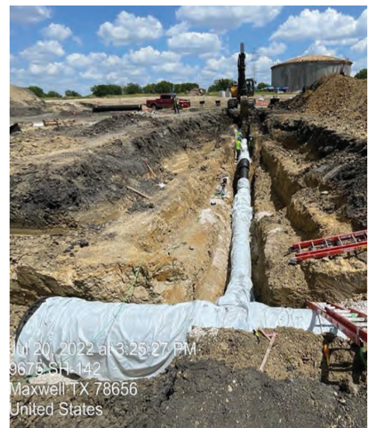
BPS – Pump Station Backfill
