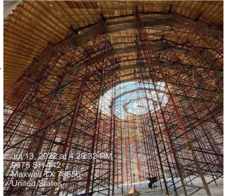
GST Shoring for dome placement
