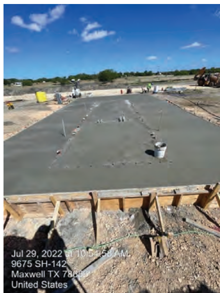
BPS – Generator Concrete Placement
