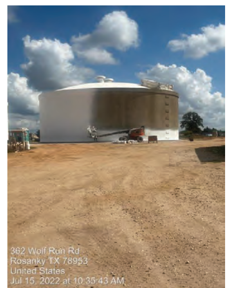
WTP – Raw Water Tanks Exterior Coating
