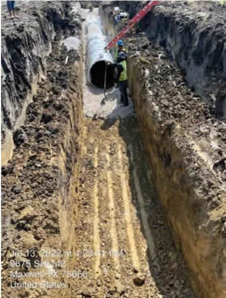
Segment B 36" DIP at STA 11+60
