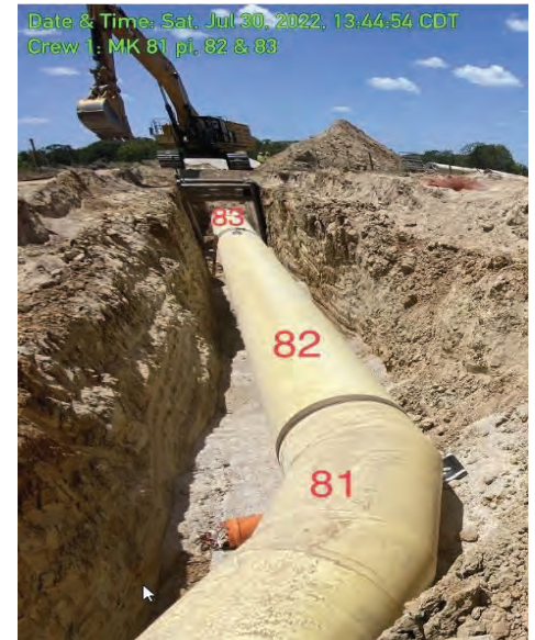
Seg A – Road Crossing Pipe Install
