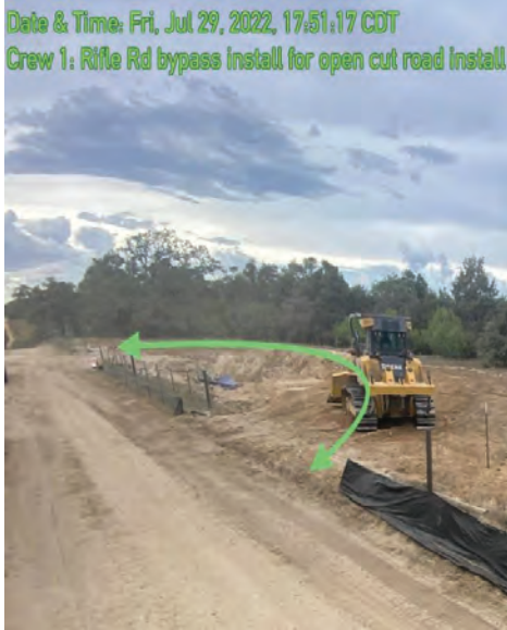
Seg A – Rifle Rd Bypass Install
