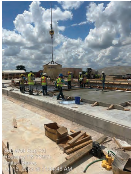
WTP– Filter Unit Housekeeping Pad of Filter Complex
