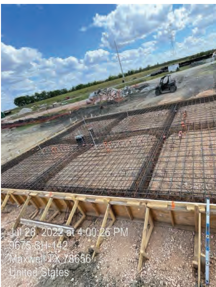
BPS – Generator Pad Prior to Concrete Placement
