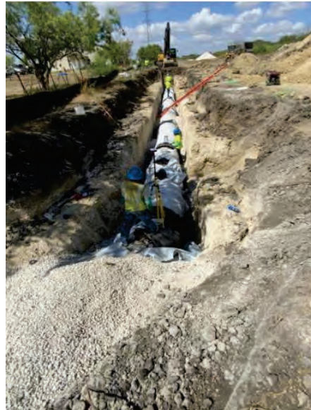
BPS – Segment B1 42" DIP at STA 11+67
