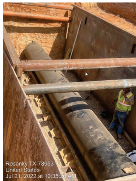
WTP – Raw Waterline WL-C Bore and Casting at STA 23+50
