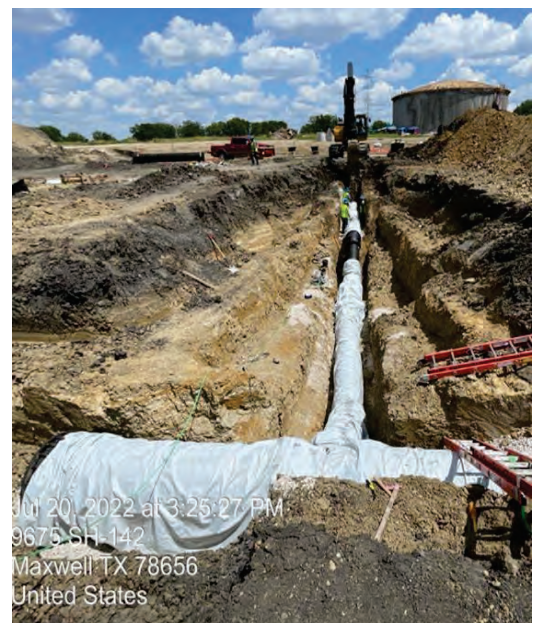
BPS – Pump Station Backfill
