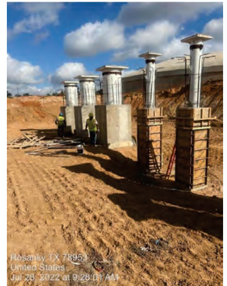
WTP– HSPS Plant Water Pump Can Encasement Formwork
