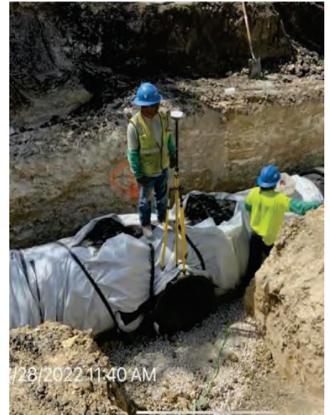
BPS – Segment B1 42" DIP at STA 12+71
