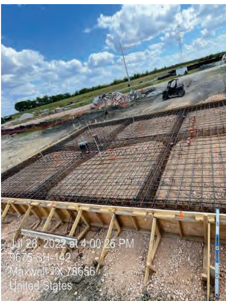
BPS – Generator Pad Prior to Concrete Placement
