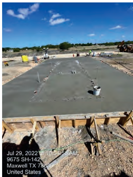
BPS – Generator Concrete Placement
