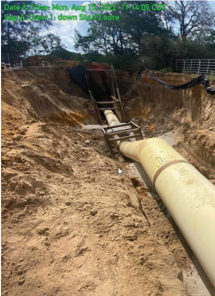
Seg A – Bore #3 Bore Excavation
