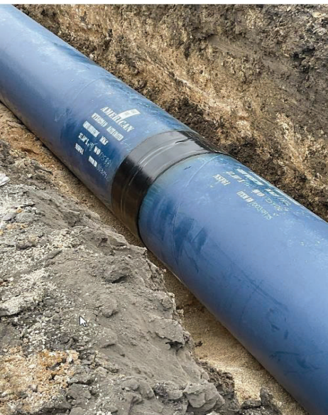
Seg B – 36-Inch Shrink Sleeve Placement
