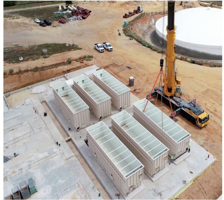
Filter Installation
