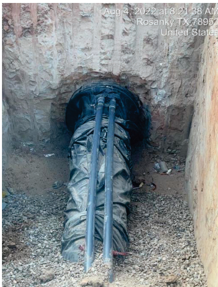
WTP – Casing & Fiber Conduits on Raw Waterline WL-A at STA-23+80
