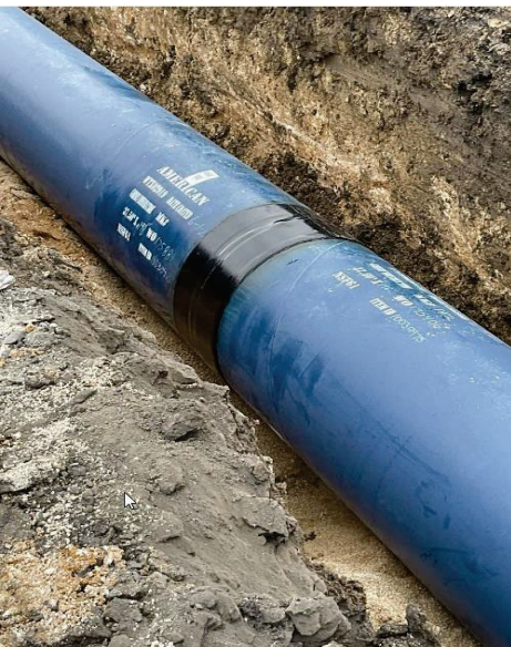
Seg B – 36-Inch Shrink Sleeve Placement
