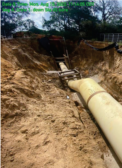
Seg A – Bore #3 Bore Excavation
