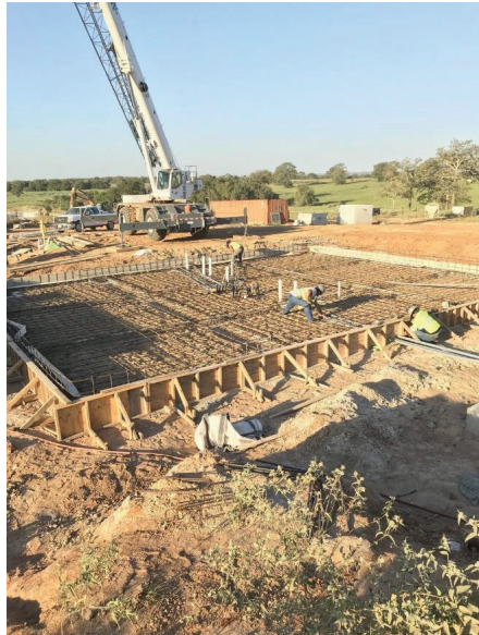
WTP – Lime System Foundation
