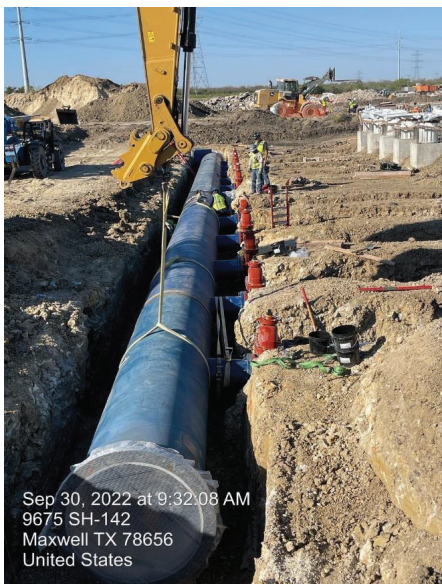
BPS – Pump Station Suction Header
