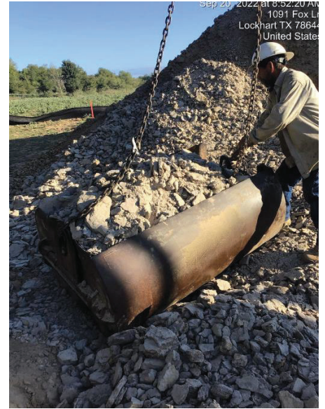
Seg A – Bore#9 Material Removal
