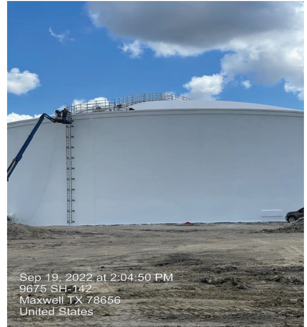
BPS – GST Ladder and Handrail Installation
