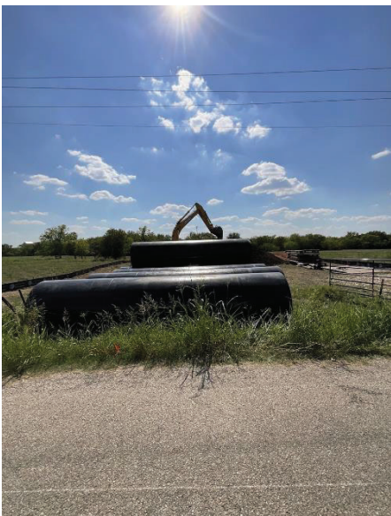
Seg B – Staging 60” casing at Tunnel #11
