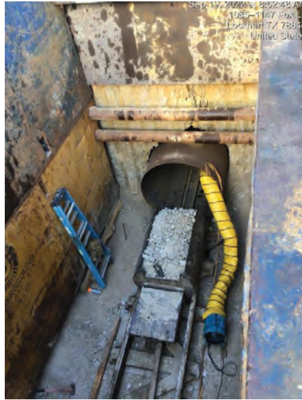
Seg A – Bore #9 Completed 80" of Hand Digging
