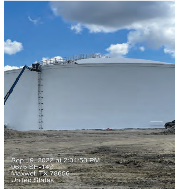
BPS – GST Ladder and Handrail Installation
