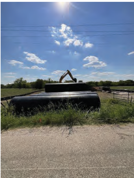
Seg B – Staging 60” casing at Tunnel #11
