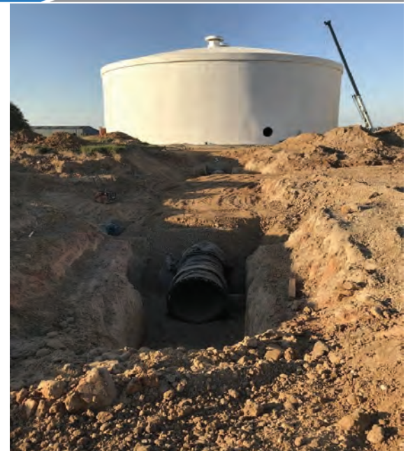
WTP - 36" GW Line to Raw Water Tanks
