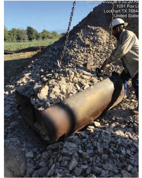
Seg A – Bore#9 Material Removal
