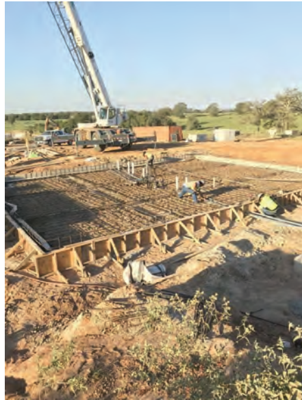
WTP – Lime System Foundation
