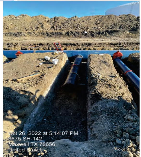
BPS – Seg B Discharge Pipe Installation from Suction Header
