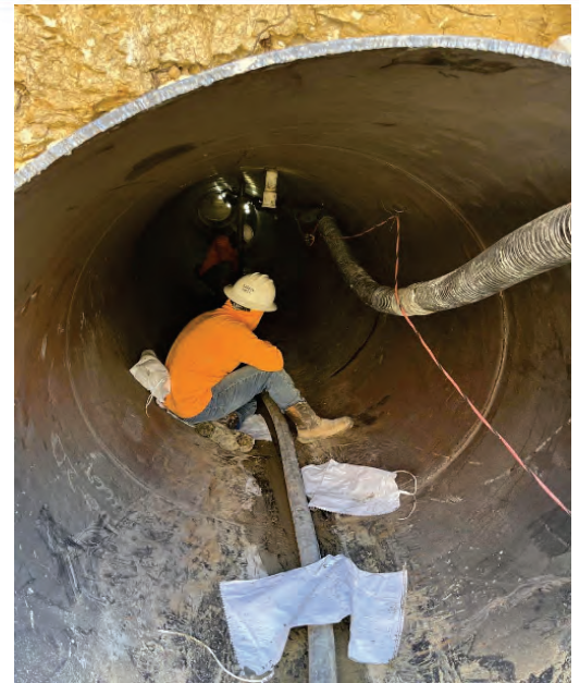
Seg B – Bore #9 - BORECO Placing Contact Grout
