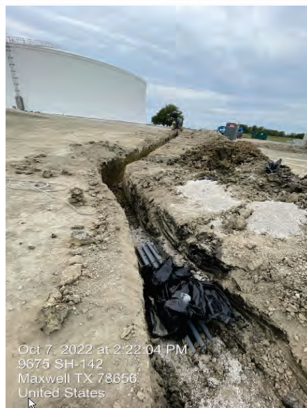
BPS – Electrical Ductbank work from Electrical building to GST
