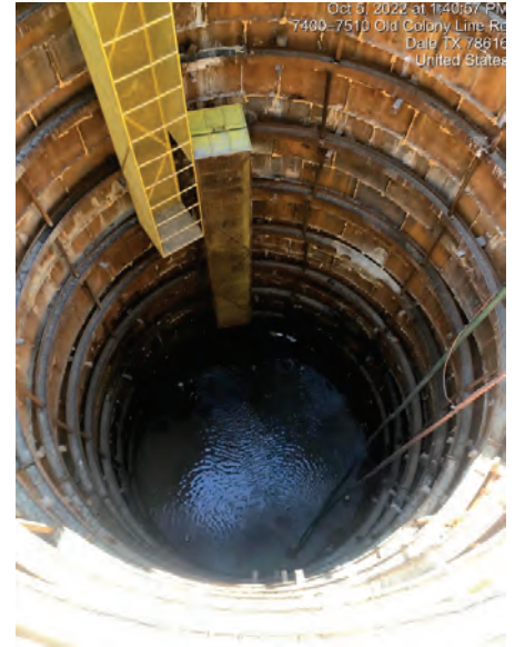
Seg A – Plum Creek Receiving Pit Pump Out 11
