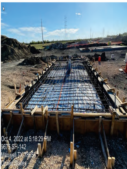
BPS – Electrical Building Slab Formwork and Reinforced Steel
