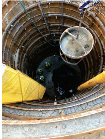
Seg A – Plum Creek Placing Concrete Floor
