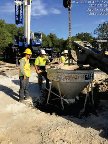
Seg A – Plum Creek Loading Concrete into Hopper
