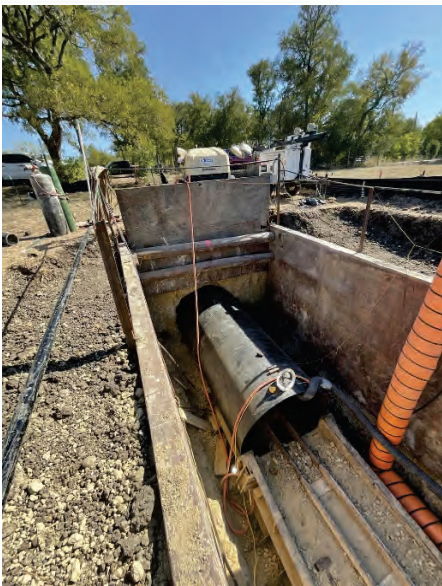
Seg B – Bore #9A – BORECO Placing 60” Casing
