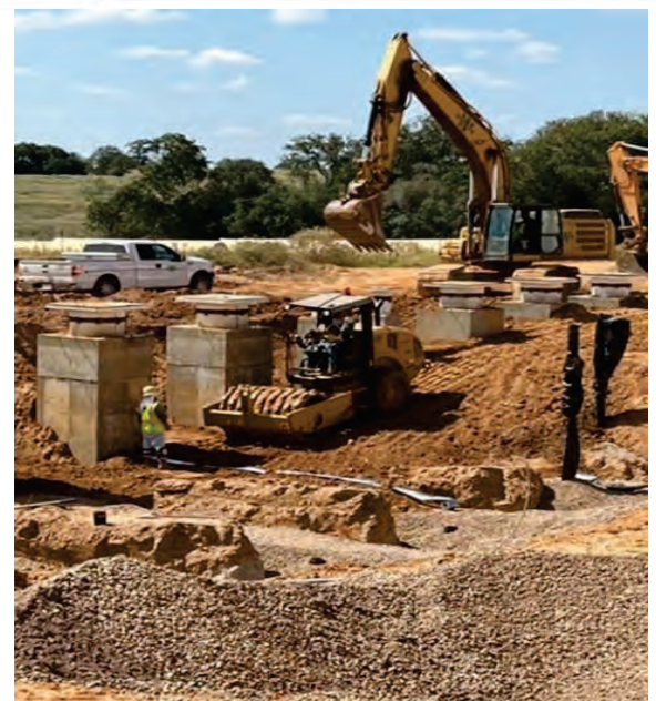
WTP - HSPS backfill PW Lines to Pumps
