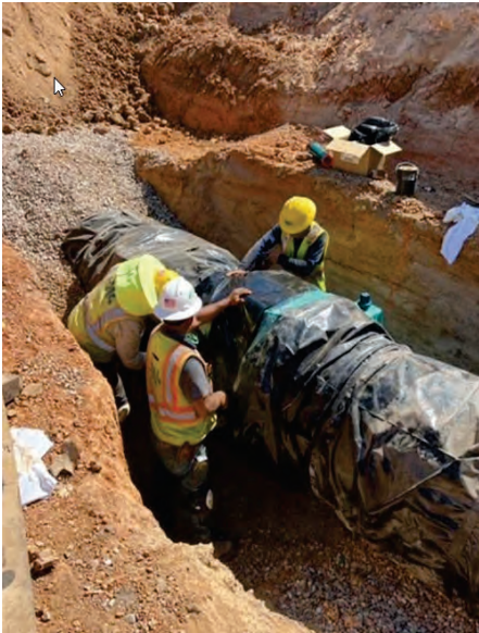
WTP – Wrap fittings on 36" Ground Water Piping to GBRA RW Tank
