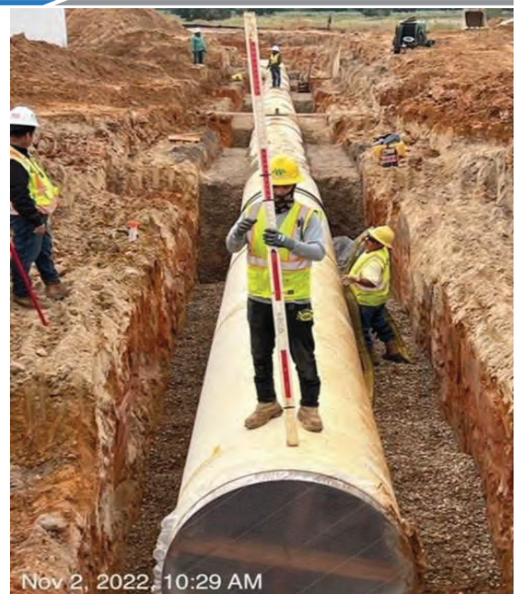
WTP – 48" Potable Water Line A Setting Pipe HSPS-81
