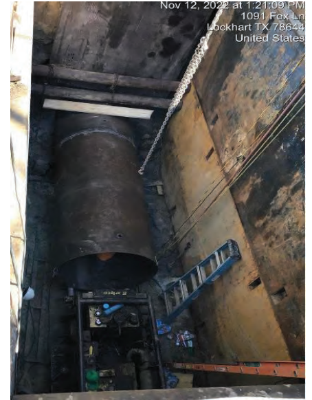
Seg A – Daniel Creek Place and Weld Encasement Pipe 11
