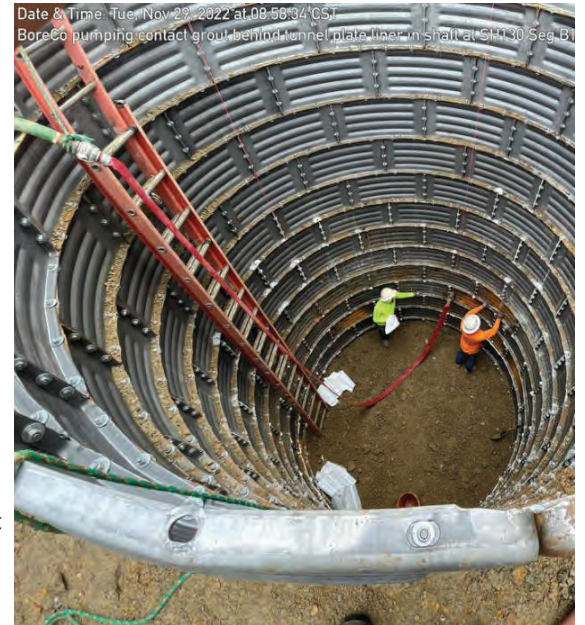
SH130 – BoreCO Pumping Grout behind Tunnel Plate Liner
