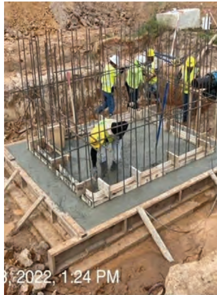
WTP – Fire Line Meter Vault Floor Concrete Placement
