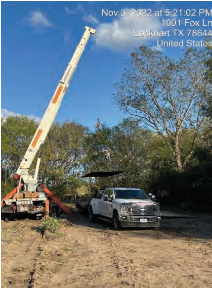
Seg A – Daniel Creek Equipment Mobilization
