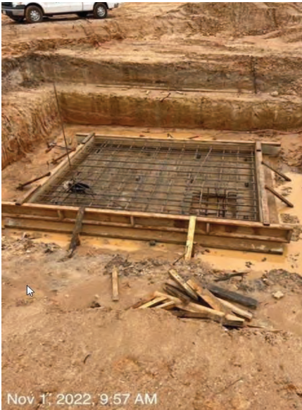
WTP – Fire Line Meter Vault Setting Rebar for Floor
