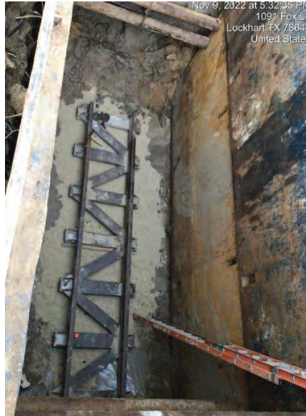
Seg A – Daniel Creek Bore setup on West Side
