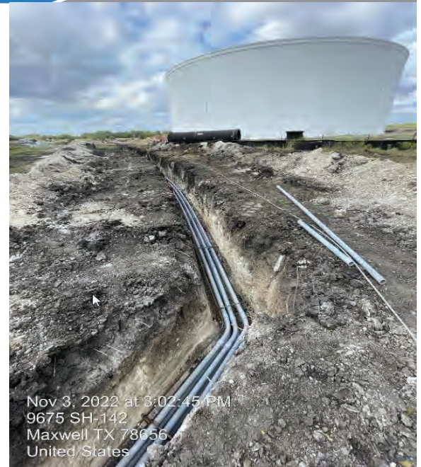
BPS – D Ductbank Installation
