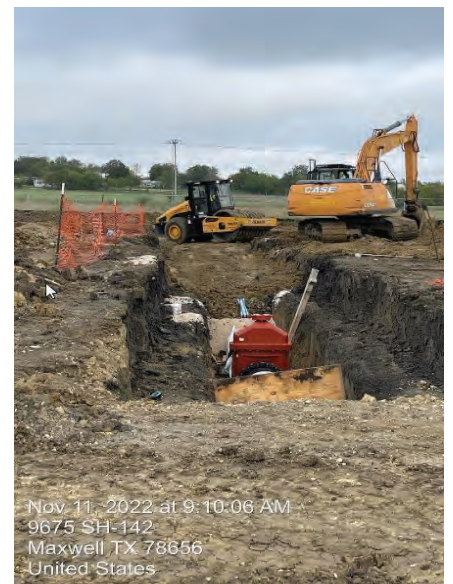
BPS – Backfilling towards STA 12+86
