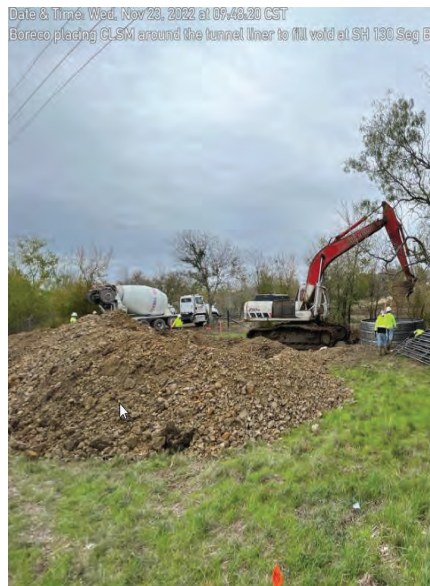
Seg B – SH130 BoreCo Placing CLSM around Tunnel Liner
