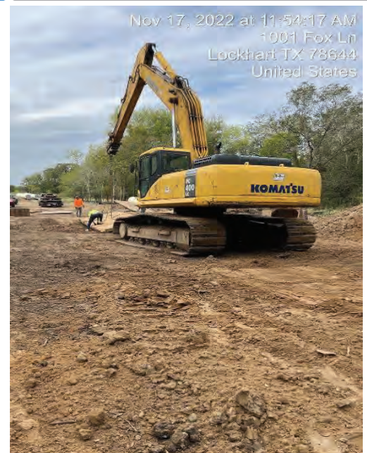
Seg A – Daniel Creek subcontractor Casing Placement
