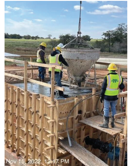
WTP – Backfill 36" Ground Water Piping to GBRA RW Tank
