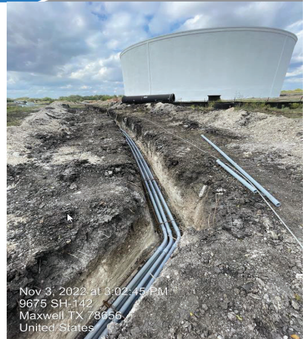
BPS – D Ductbank Installation
