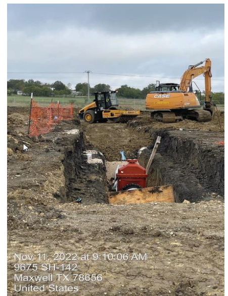
BPS – Backfilling towards STA 12+86
