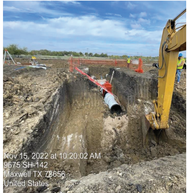
BPS – Flow Meter Vault Excavation for Segment D
