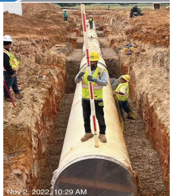
Nov 2, 2022, 10:29 AM WTP – 48" Potable Water Line A Setting Pipe HSPS-81
