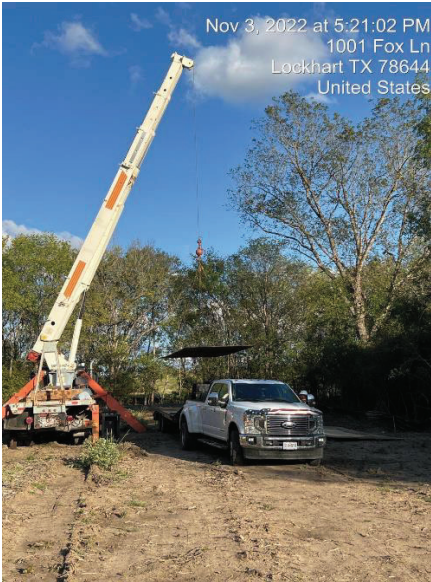
Seg A – Daniel Creek Equipment Mobilization
