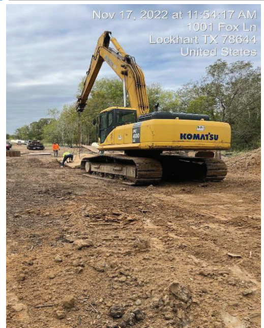
Seg A – Daniel Creek subcontractor Casing Placement
