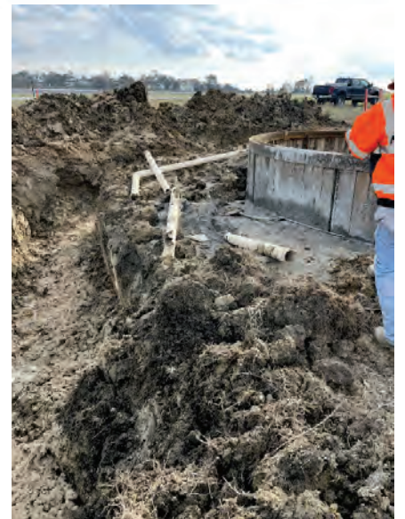
Seg B – SH130 – BORECO Excavated 4" Water Line at Entry Pit
