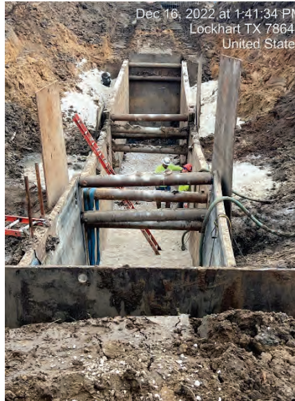
Seg A – STA 671+00 - Casing Placement Preparation
