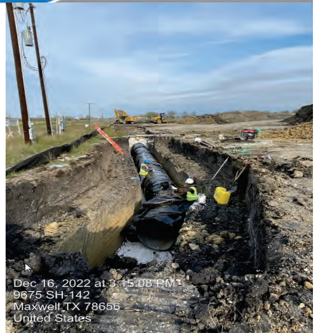
BPS – Segment C Piper Rework STA 1+05
