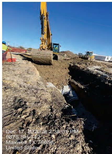
BPS – Segment B Pipe Rework
