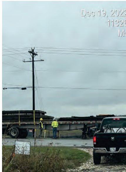
Seg D – Equipment Mobilization
