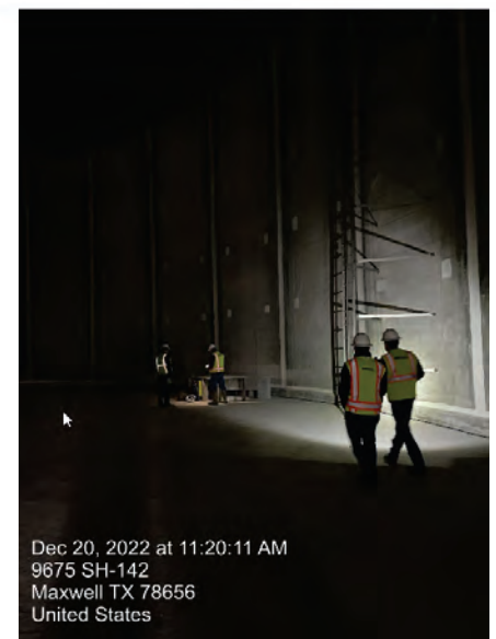
BPS – Ground Storage Tank Inspection
