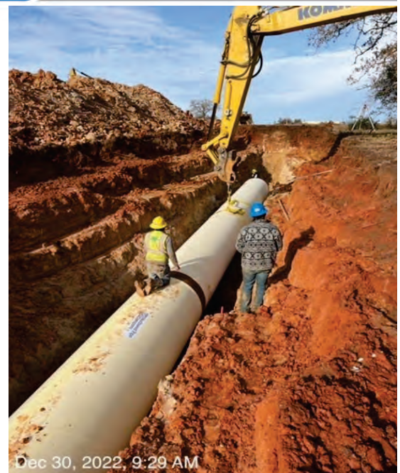
WTP – 48" Potable Water Line Setting Pipe-57
