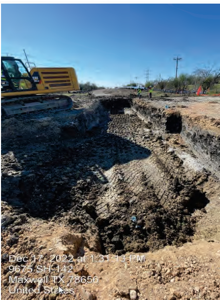
BPS – Segment B Pipe Rework Looking Towards 0+00
