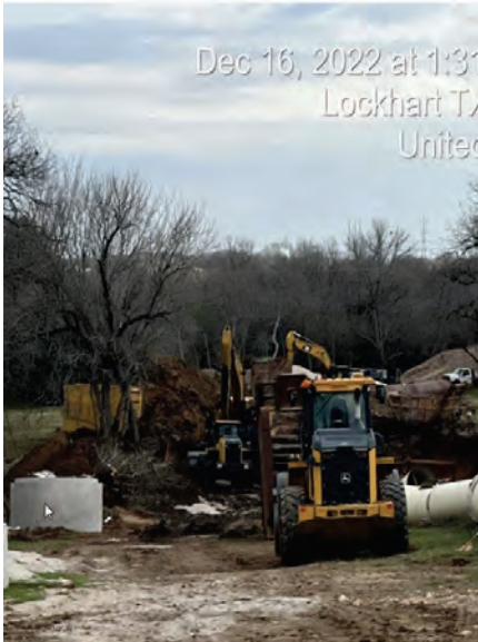
Seg A – STA 671+00 - Casing Placement Preparation
