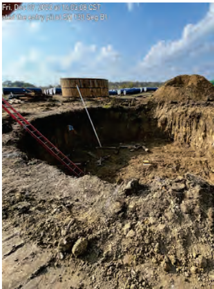
Seg B – SH130 – BORECO Excavating Entry Pit
