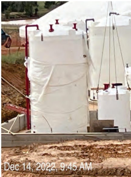
WTP – Filter Complex Setting Sodium Permanganate Tank
