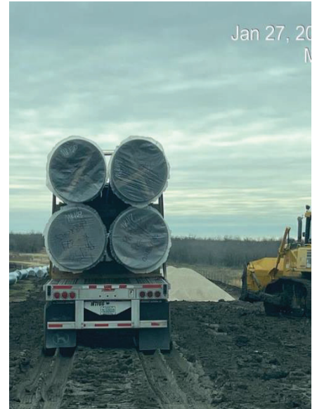
Seg D – Northwest Pipe Deliveries
