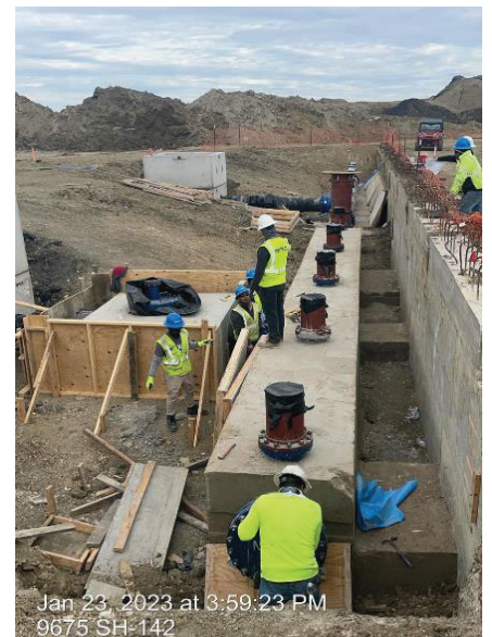
BPS – Stripping Forms for Seg D Discharge Header Flowable Fill Encasement
