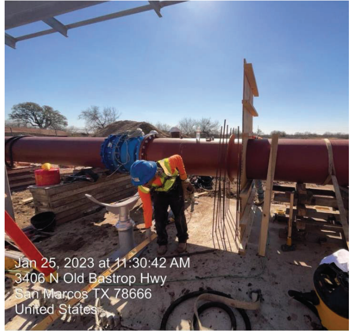
BPS – Rebar Installation for Thrust Block at San Marcos
