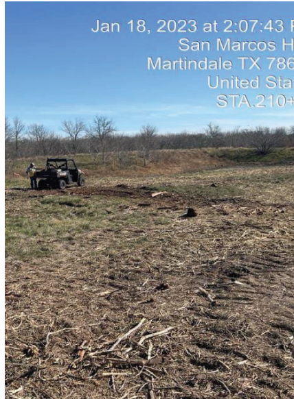
Seg D – Surveying for easement along HWY 80
