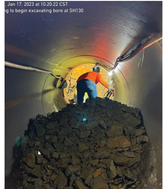
SH130 – BORECO Began Hand Tunneling
