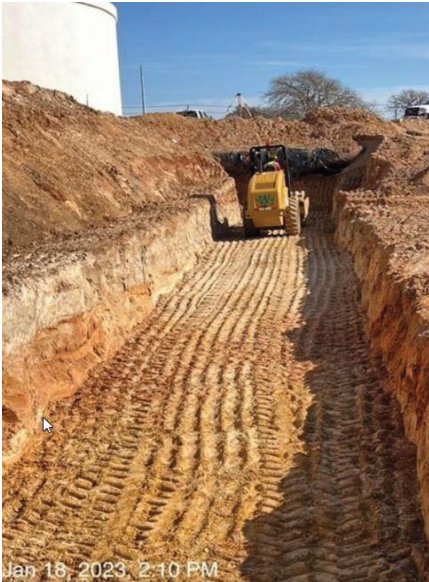
WTP – Compacting Retaining Wall Subgrade
