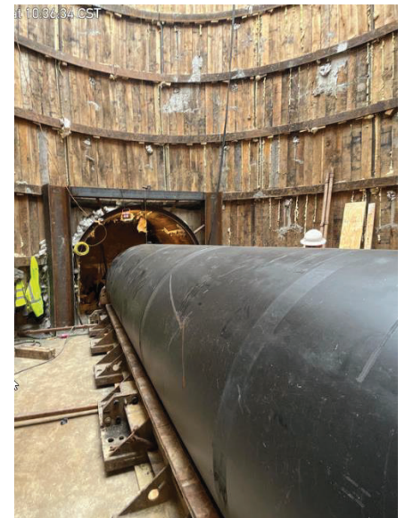
Seg B – SH130 BORECO Aligning Casing
