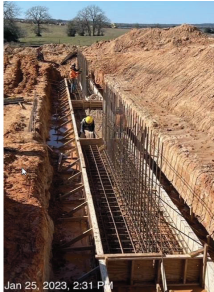
WTP – Retainer Wall Rebar
