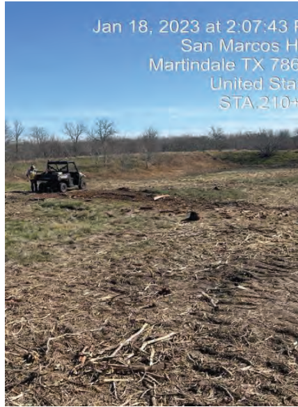
Seg D – Surveying for easement along HWY 80
