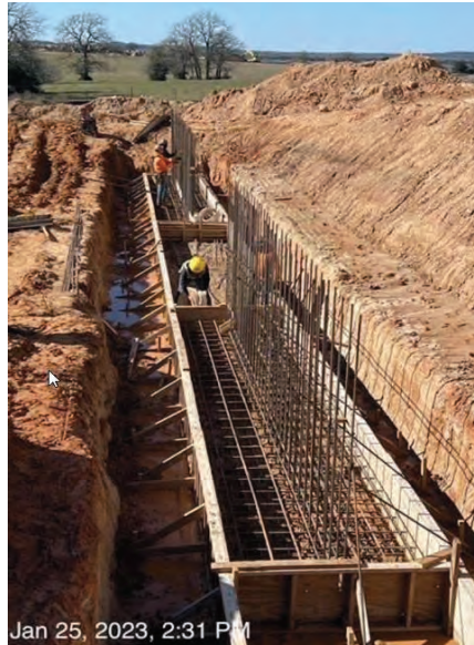
WTP – Retainer Wall Rebar
