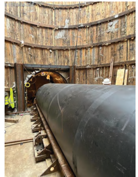
Seg B – SH130 BORECO Aligning Casing
