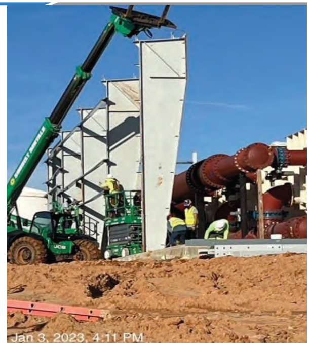
WTP – Filter Complex Grid Line 9 Settings Structural Steel
