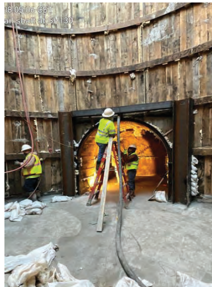
Seg B – SH130 BORECO Placing Contact Grout in Tail Shaft
