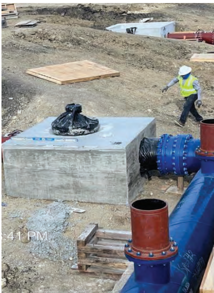
BPS – Seg D Formwork Removal for Concrete Encasement
