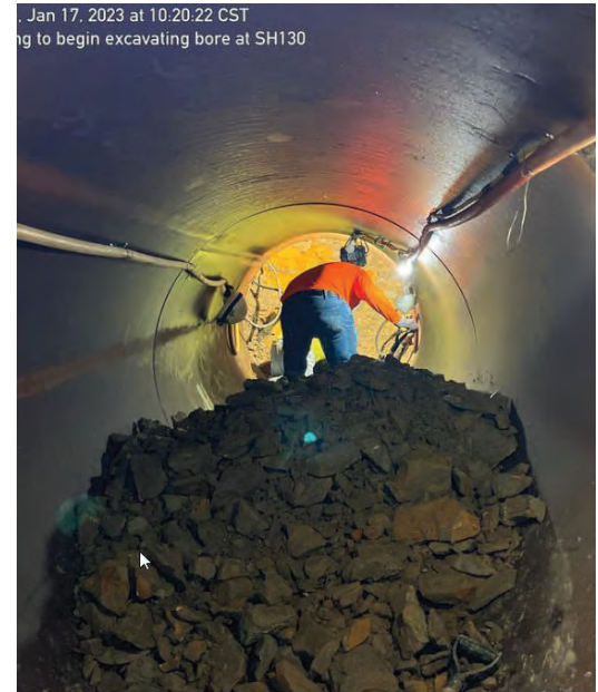
SH130 – BORECO Began Hand Tunneling
