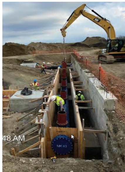
BPS – Seg D Formwork for Flowable Fill Discharge Header
