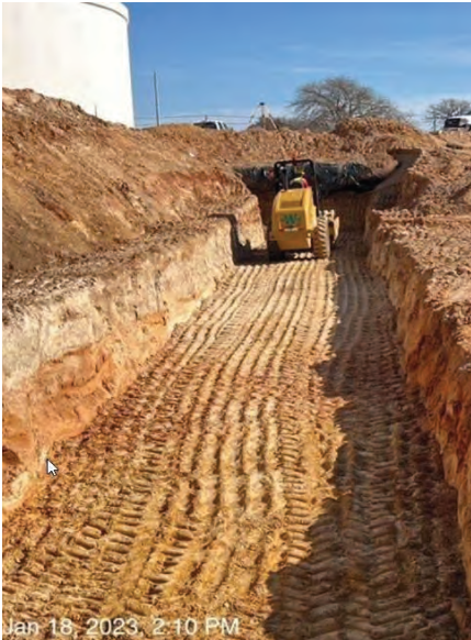
WTP – Compacting Retaining Wall Subgrade
