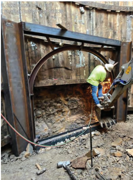
Seg B – SH130 BORECO Assembling Frame for Tail Shaft
