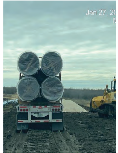
Seg D – Northwest Pipe Deliveries
