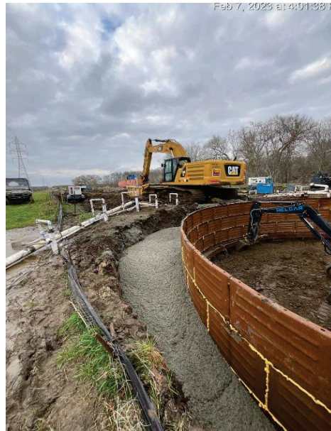
Seg A – Melcar Places Concrete around Liner Plates
