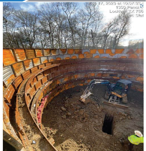
Seg A – RCP-Excavation of Bore Pit
