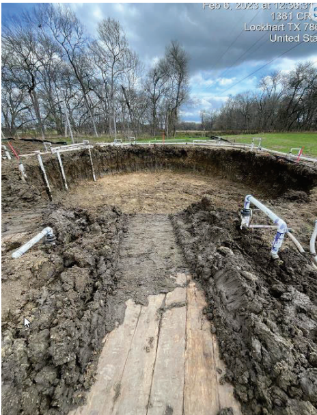
Seg A – Melcar Excavation for Liner Plates
