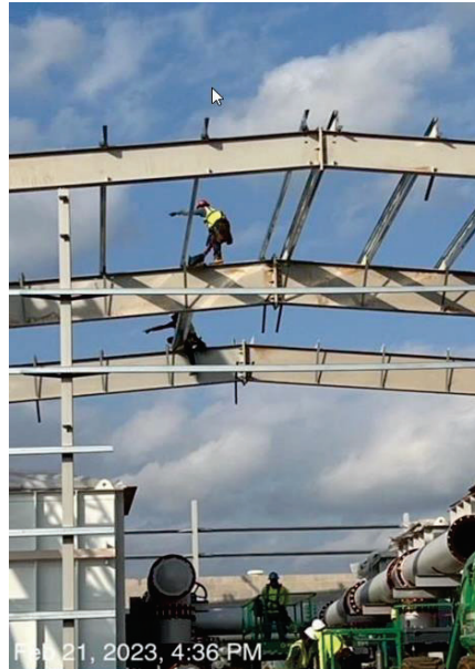
WTP – Filter Complex Setting Roof Purlins
