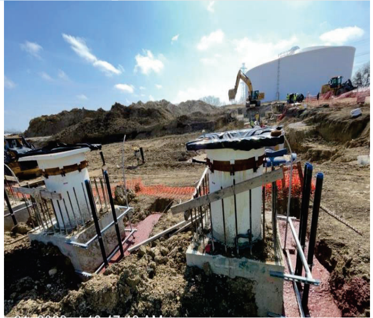
BPS – Concrete Placement for Electrical Ductbanks for Pump Station
