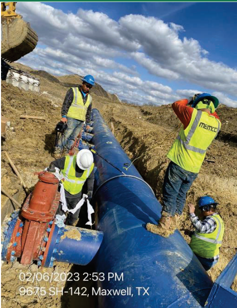
BPS – Holiday Testing Suction Header
