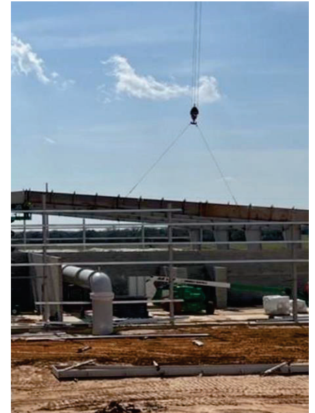
WTP – Filter Complex Setting Roof Beams
