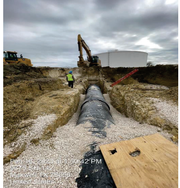
BPS – Suction Line Pipe Installation Near STA 60+00
