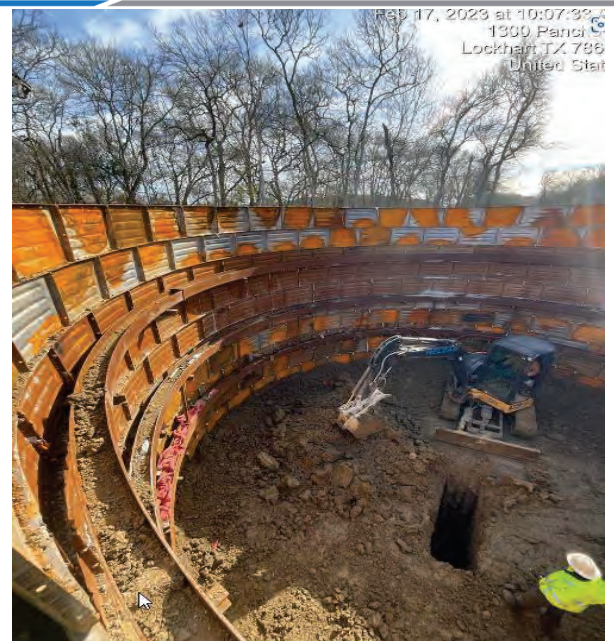
Seg A – RCP-Excavation of Bore Pit
