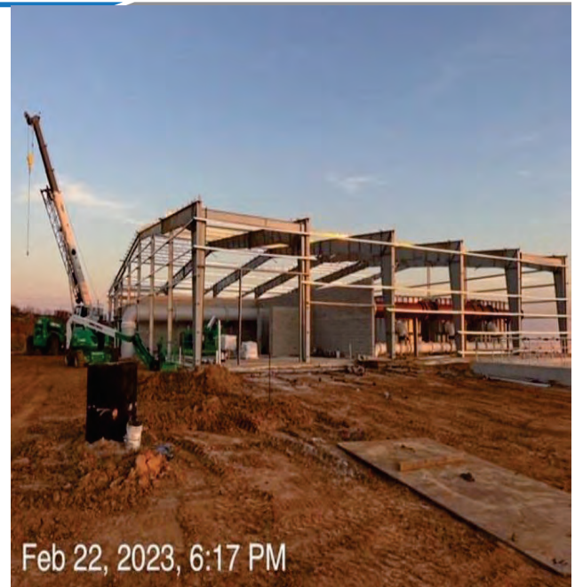
WTP – Filter Complex, Roof Beams Installed
