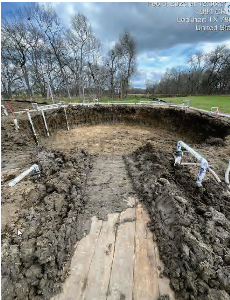
Seg A – Melcar Excavation for Liner Plates
