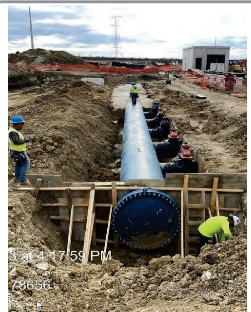
BPS – Formwork Installation for Flowable Fill for Suction Header
