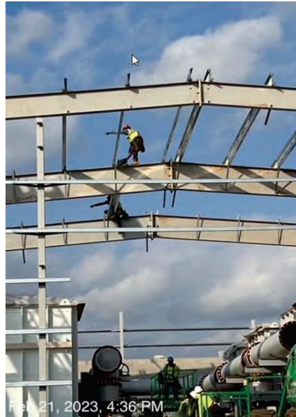
WTP – Filter Complex Setting Roof Purlins
