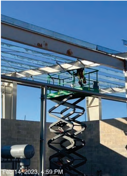
WTP – Filter Complex Re-drill Holes on Roof Purlins
