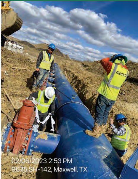
BPS – Holiday Testing Suction Header
