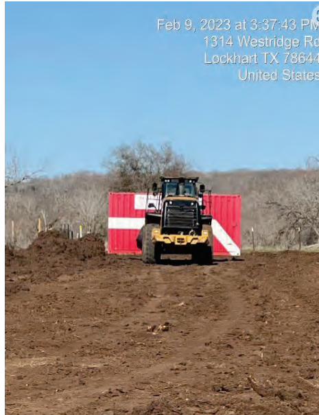
Seg D – Equipment Mobilization
