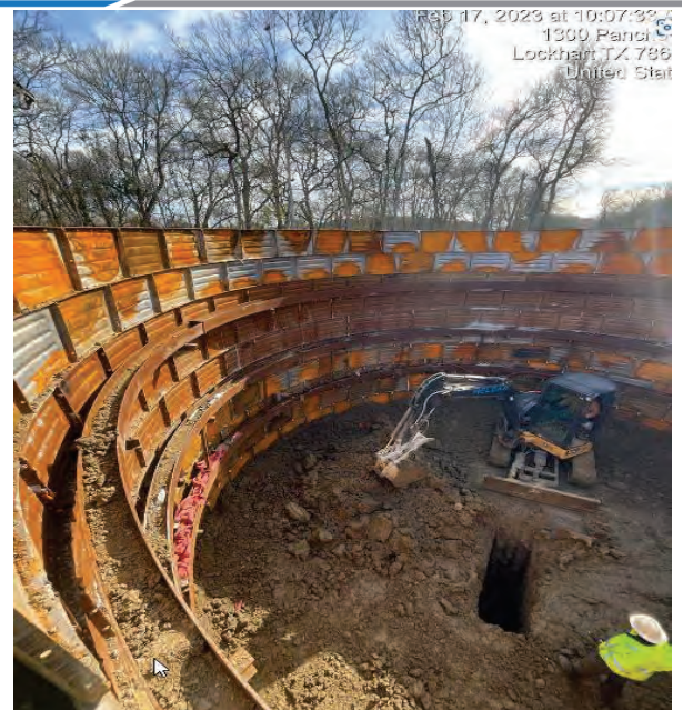
Seg A – RCP-Excavation of Bore Pit
