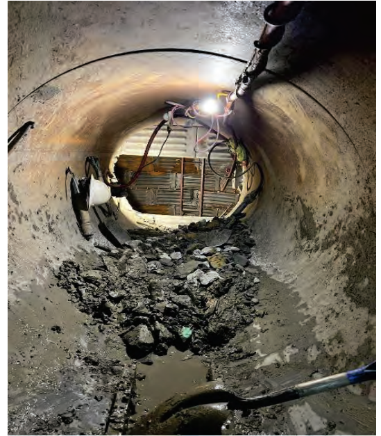
SH130 – BORECO Completed Bore Seg B2
