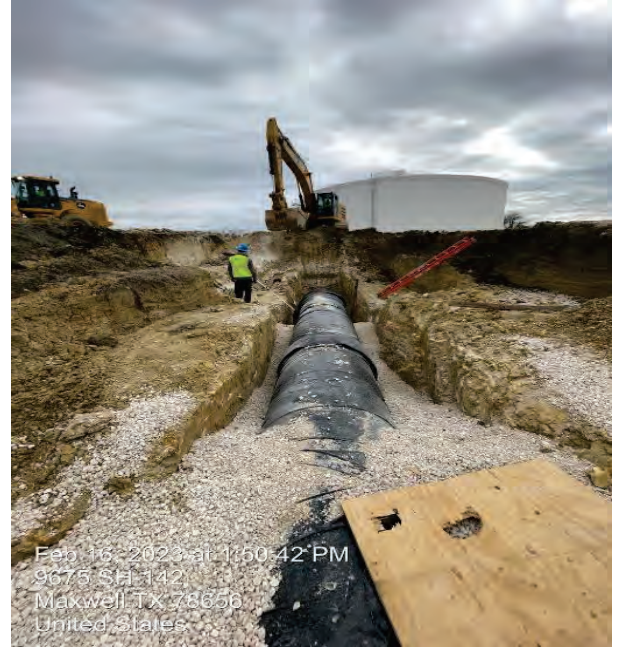
BPS – Suction Line Pipe Installation Near STA 60+00
