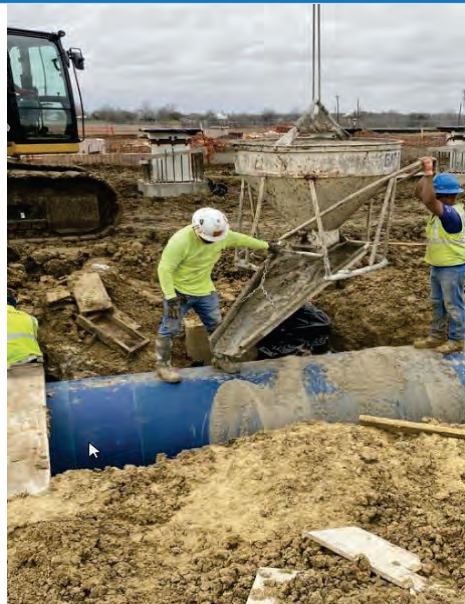
BPS – Flowable Fill Placement for Western Side of Suction Header
