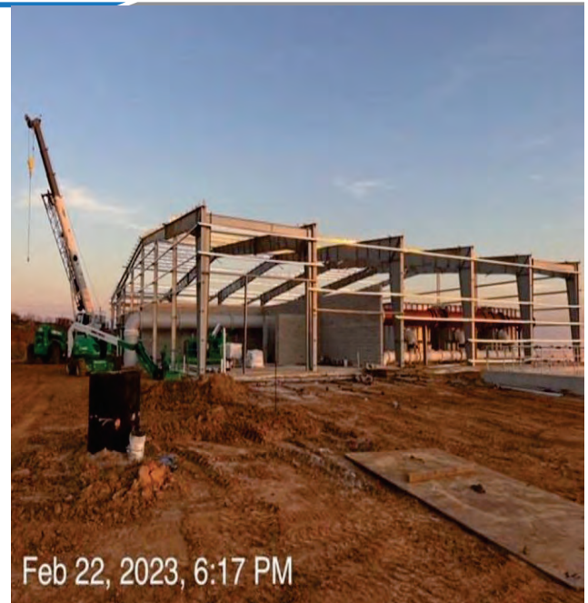
WTP – Filter Complex, Roof Beams Installed
