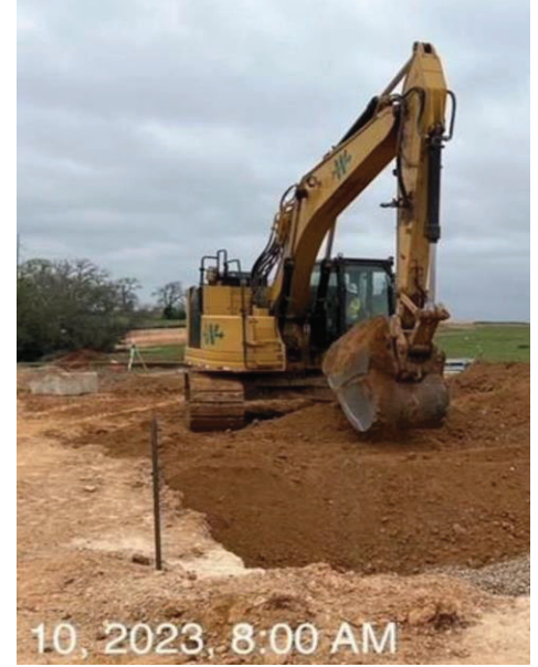
WTP – Culvert Backfill
