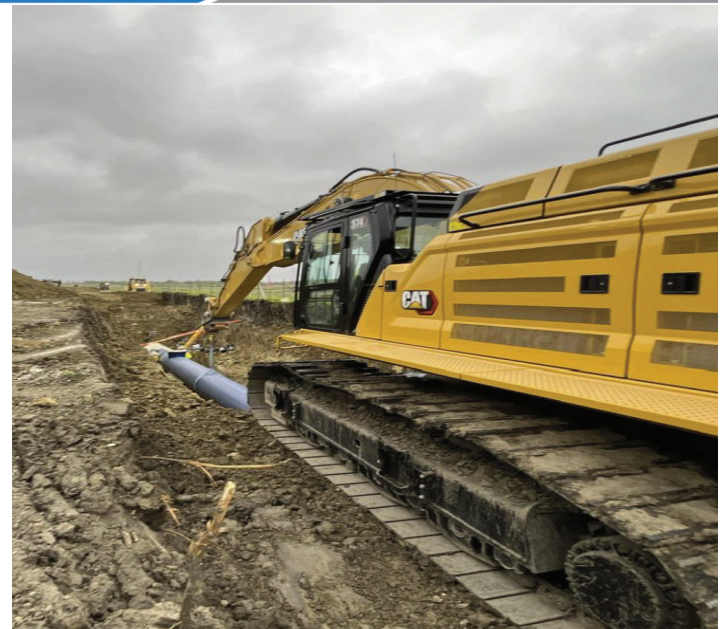
Seg D – Pipe Placement
