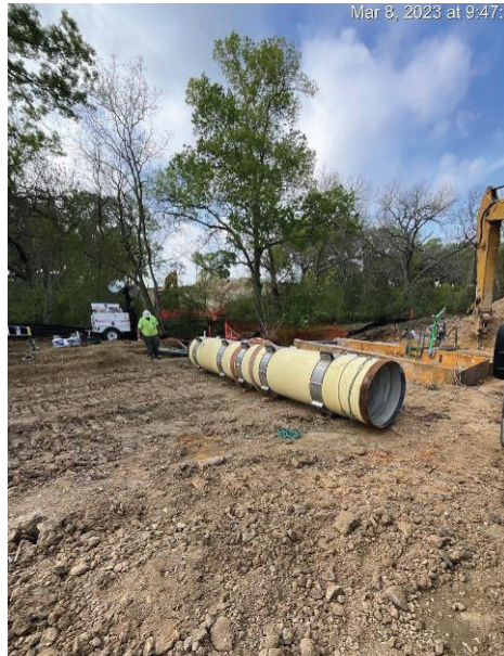
Seg A – Pipe Preparation for Placement in Encasement at Pecan Branch
