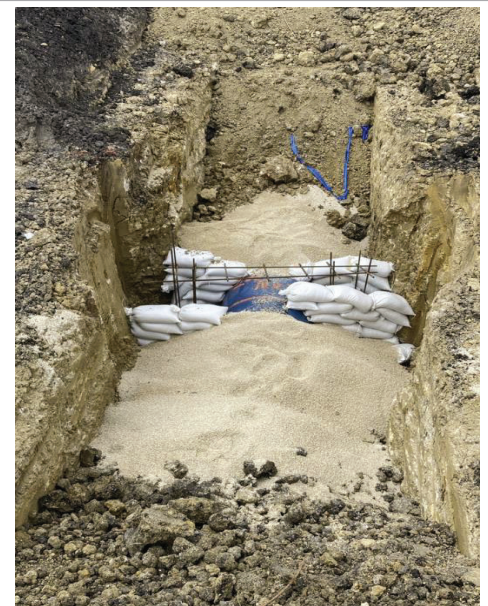
Seg B – Prepping for Concrete
