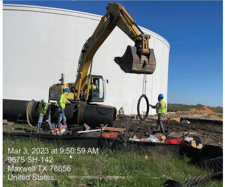
BPS – Seg B1 Pipe Installation for Tee near STA 0+69
