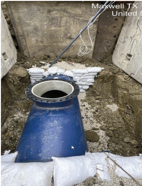
Seg D – Drain Valve Preparation
