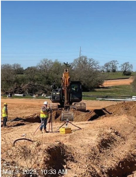
WTP – Culvert C-2 Lay Out and Start Excavation
