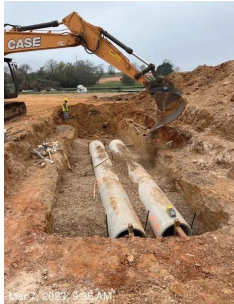
WTP – Installing C-2 Culverts Northwest of Filter Complex
