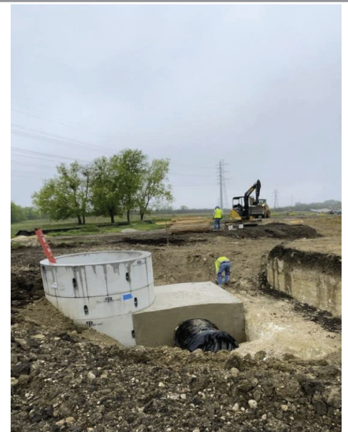
BPS – Seg B1 Formwork removal at STA 0+69
