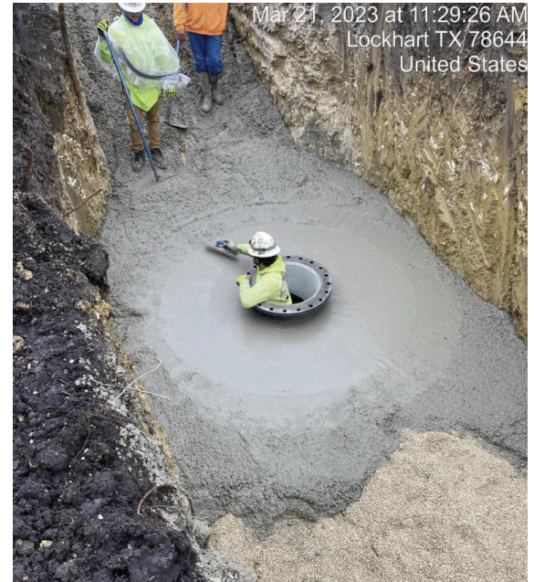
STA 495+68 – Adding Concrete Around Manhole 15
