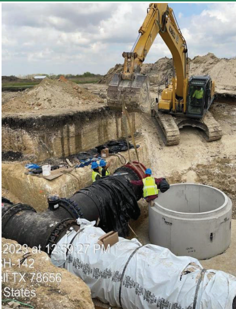
BPS – 42" Butterfly Valve Installation for Seg B1 near STA 0+69
