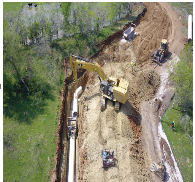
Seg A – Installing MK1064 at STA 458+90
