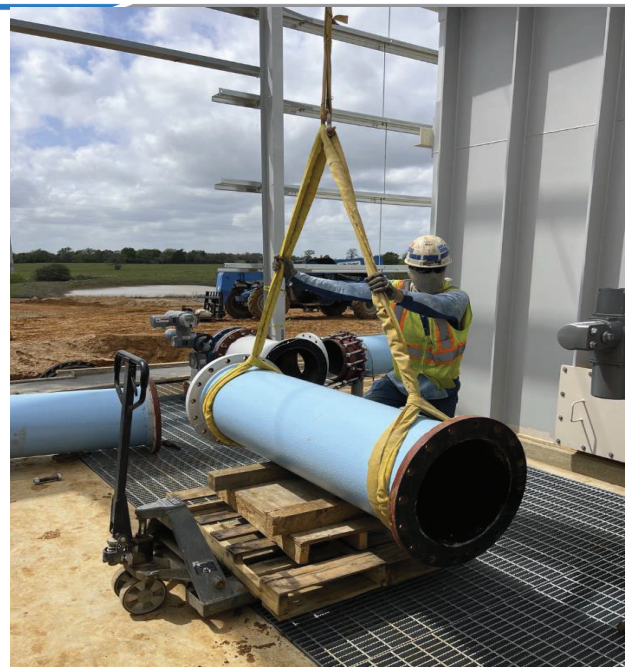
WTP – Filter Complex Installing FE Pipes
