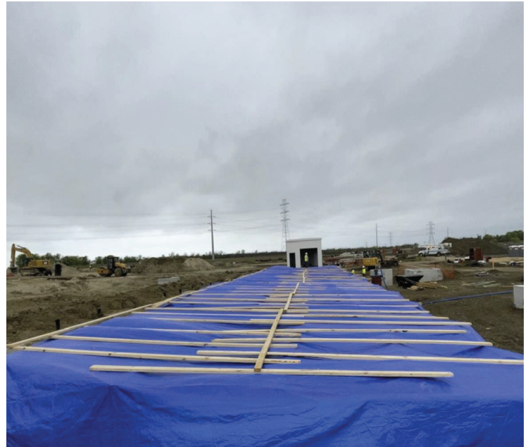
BPS – Rain Protection over Carton Form Work
