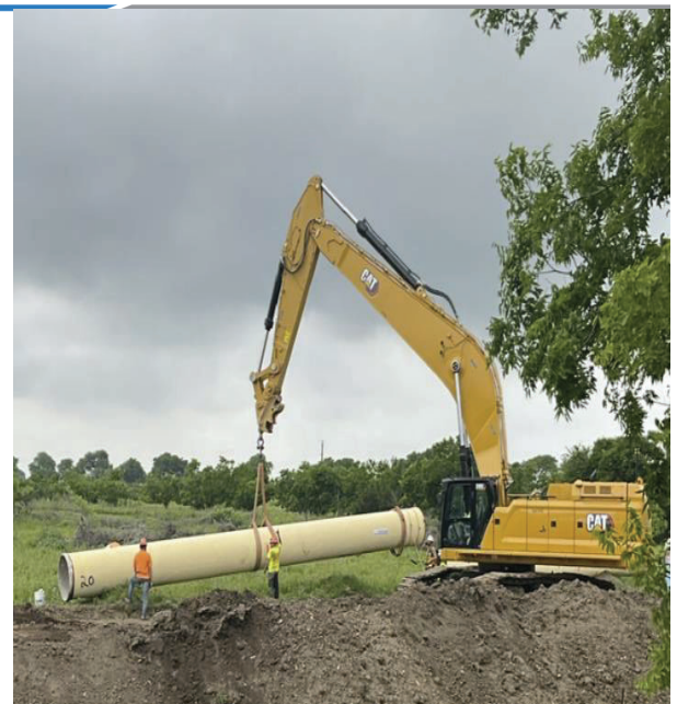
Seg A – Installing Pipe Piece 2520
