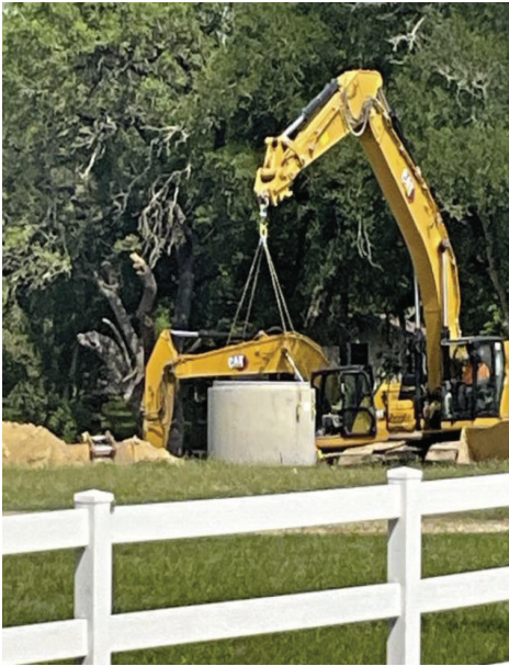
Seg A – Garney Crew Receiving Precast Manhole Section
