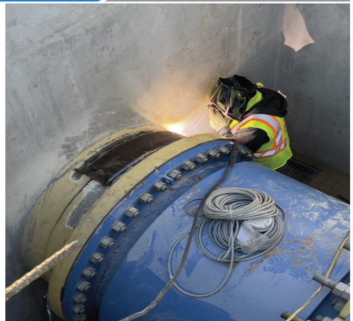
WTP – PWL Welding Butt Strap on Pipe, inside of Meter Vault.
