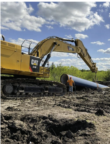
Seg B – Preparing Pipe for Placement
