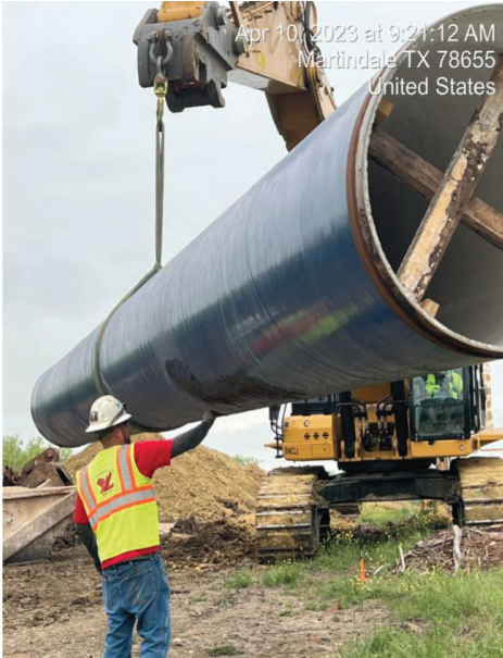
Seg D – Pipe Preparation
