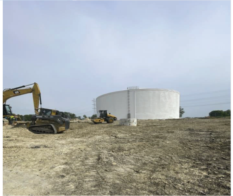
BPS – Native Backfilling Efforts for Suction Line
