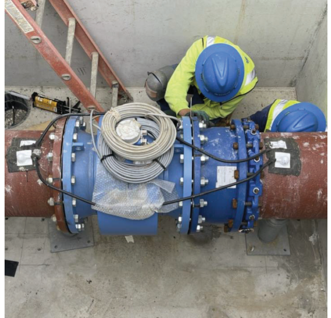
BPS – Anchoring Pipe Supports for Seg D Meter Vault Pipe
