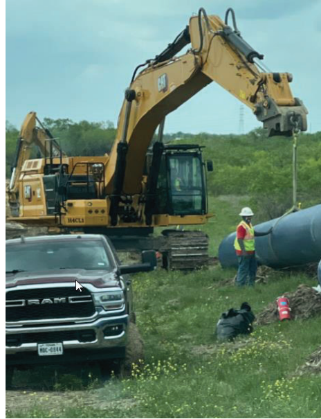
Seg D – Pipe Placement
