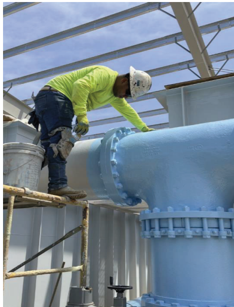
WTP – Filter Complex Painting Pipes
