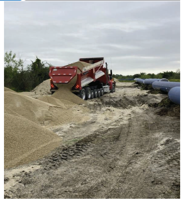
Segment A – Unloading Embedment Material
