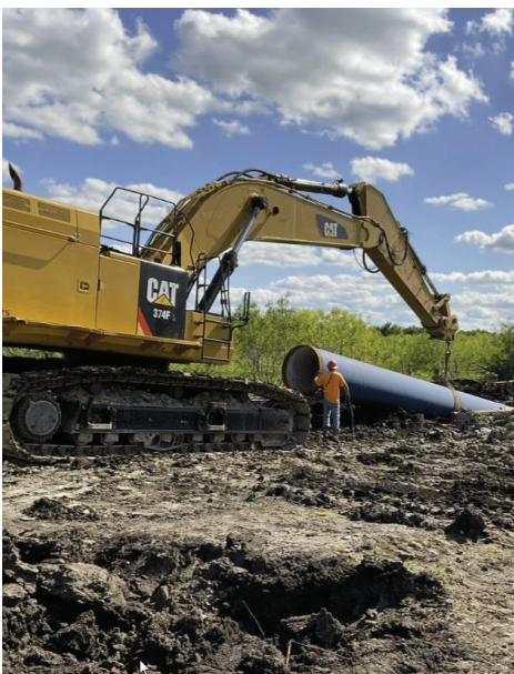
Seg B – Preparing Pipe for Placement
