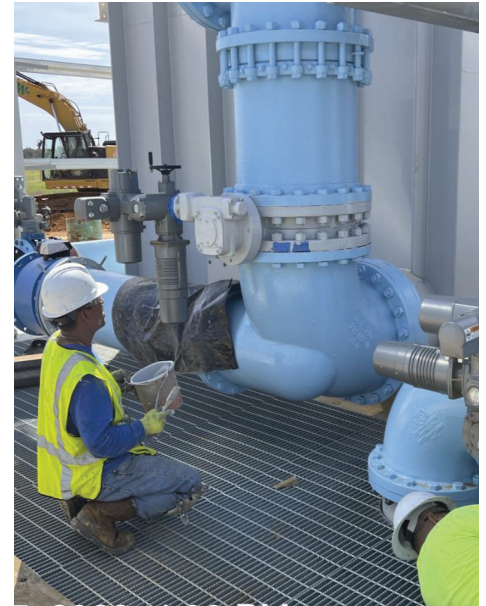
WTP – Filter Complex Painting FE Pipes 5
