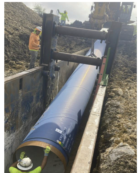
Seg B – Installing Pipe MK#2216
