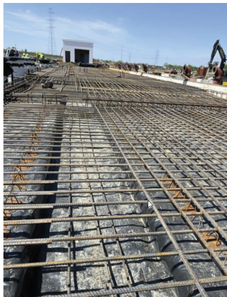
BPS – Reinforced Steel for Pump Station Slab
