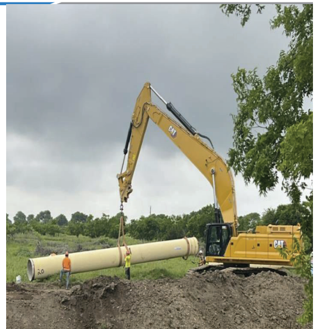
Seg A – Installing Pipe Piece 2520
