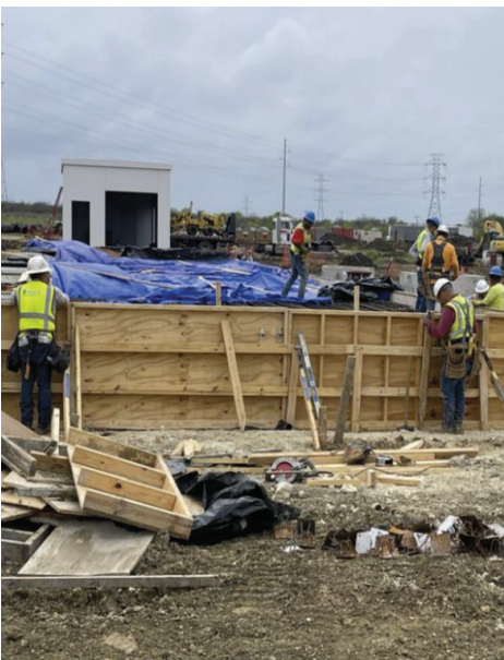
BPS – Formwork at Eastern End of Pump Station Slab
