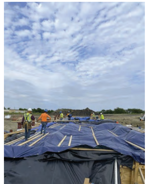
BPS – Pump Station Slab Protection from Forecasted Rain
