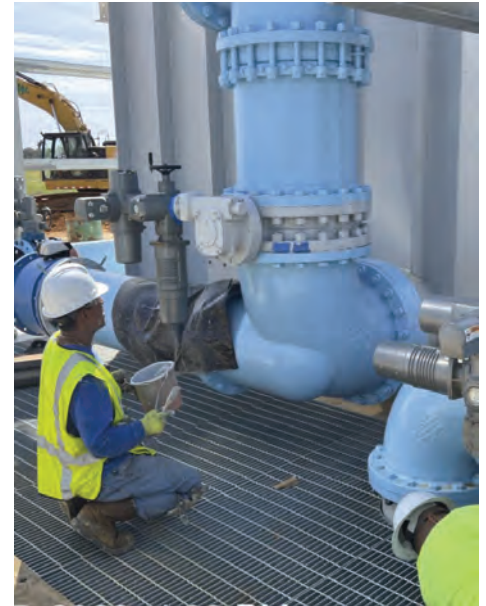
WTP – Filter Complex Painting FE Pipes 5
