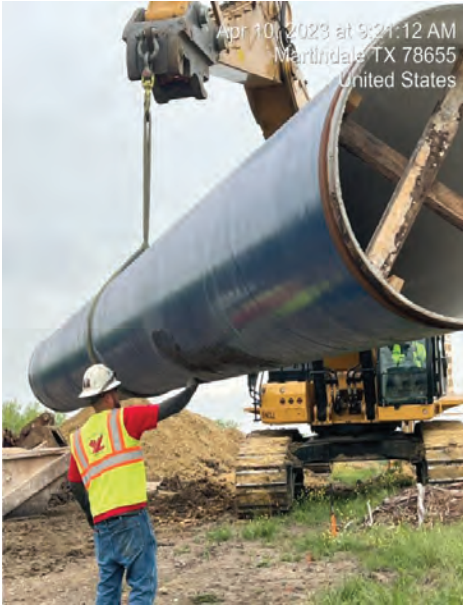
Seg D – Pipe Preparation
