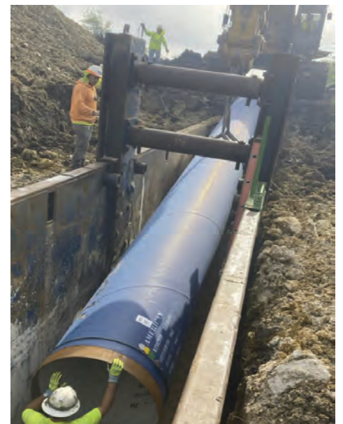
Seg B – Installing Pipe MK#2216
