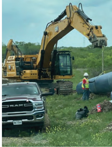
Seg D – Pipe Placement
