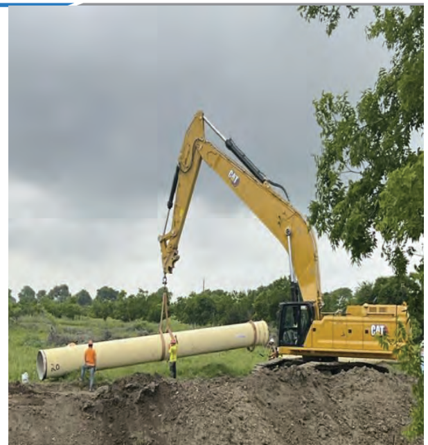
Seg A – Installing Pipe Piece 2520
