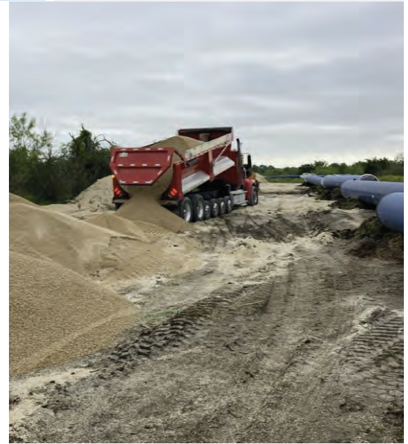
Segment A – Unloading Embedment Material
