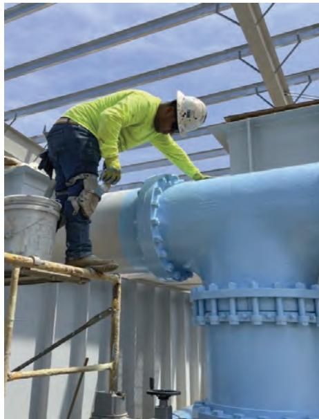
WTP – Filter Complex Painting Pipes
