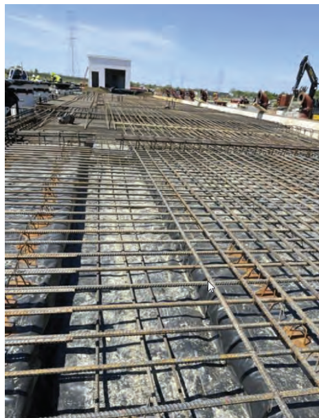
BPS – Reinforced Steel for Pump Station Slab
