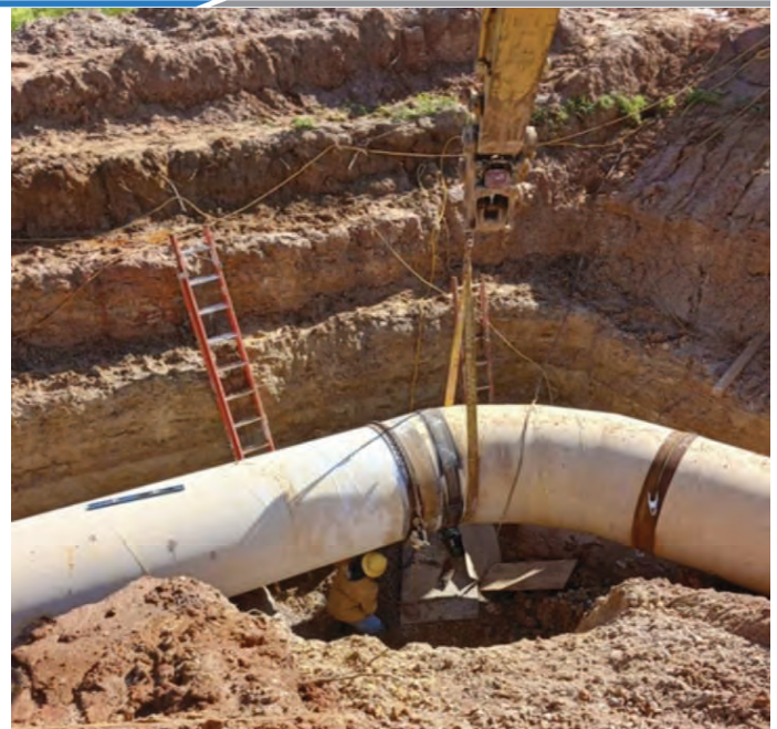
WTP – 48" Potable Water Line Welding Last Pipe
