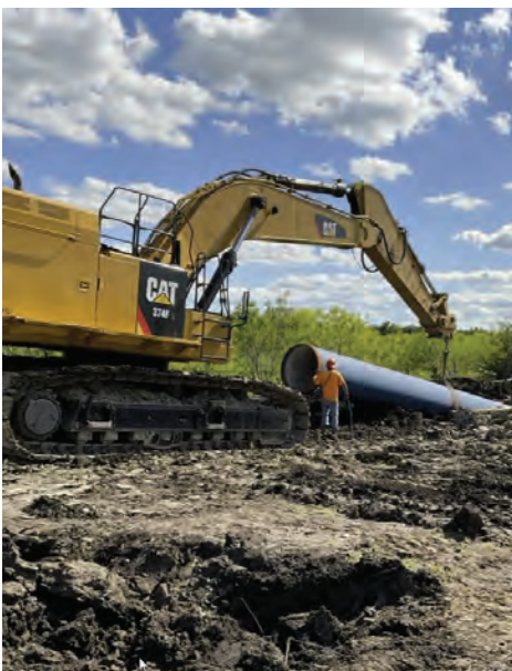
Seg B – Preparing Pipe for Placement
