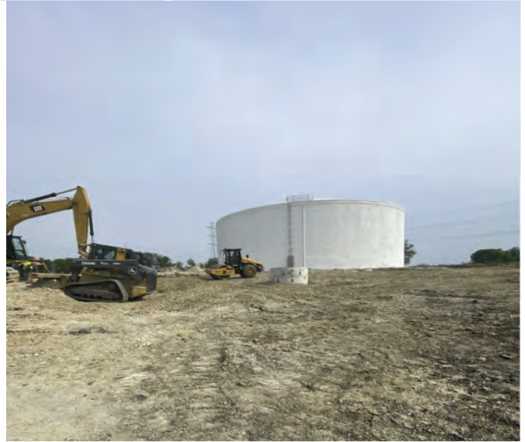
BPS – Native Backfilling Efforts for Suction Line
