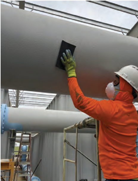
WTP – Filter Complex Sanding & Cleaning Pipes for Paint
