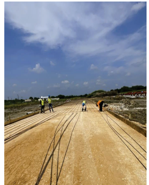
BPS – Road Paving Steel Reinforcement
