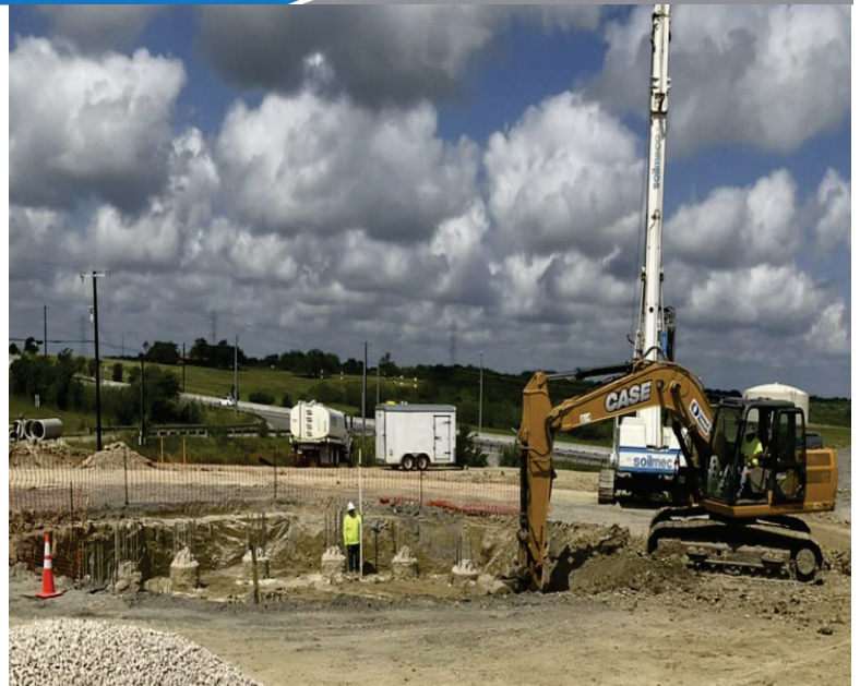
EST - Excavating Piers for Cap Placement
