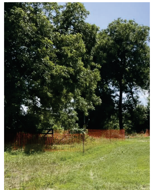
Seg E – Installed Tree Protection
