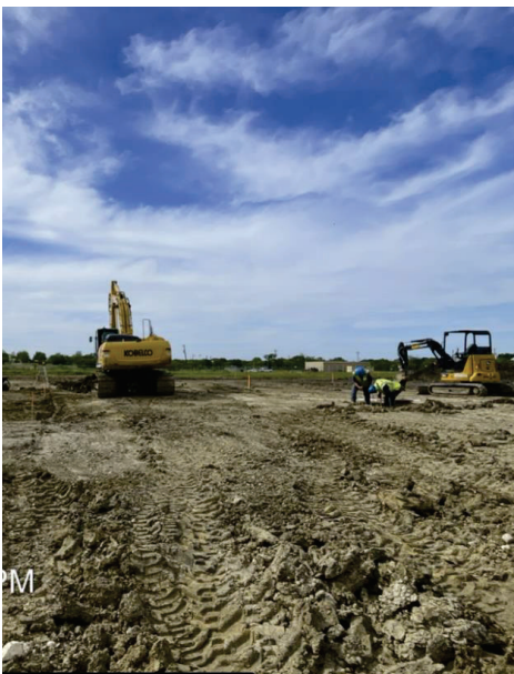
BPS – Subgrade Work for Concrete Paving
