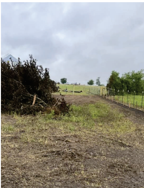
Seg E – Clearing Grubbing of Brush & Trees
