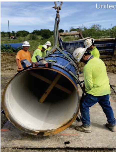
Seg B – Installing Pipe Spacers on Pipe
