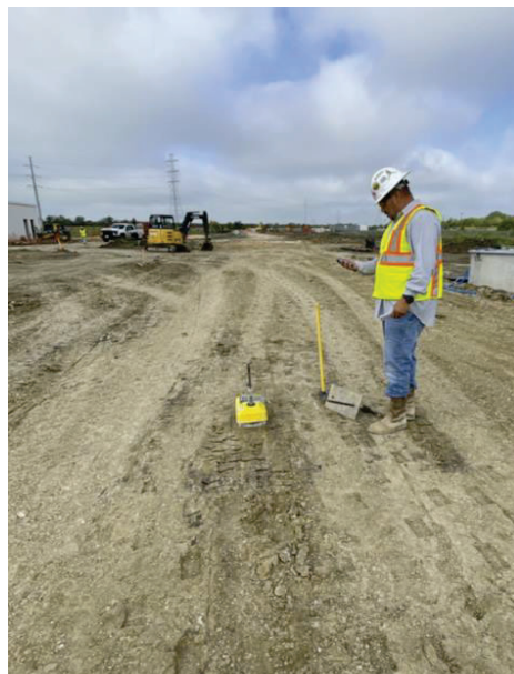
BPS – Testing Density on Paving Subgrade
