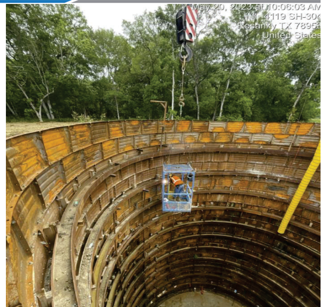
Seg A – Melcar Welds Supports to Ring Beams
