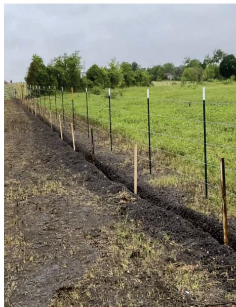
Seg E – Installing Stakes for Silt Fence
