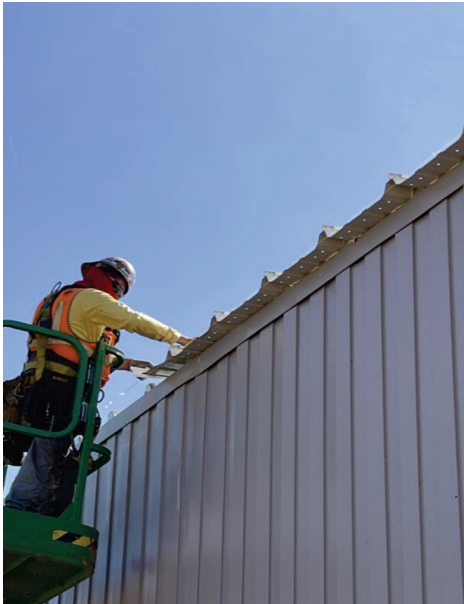
WTP – Electrical Building Roof Sheetting
