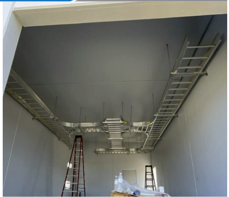
BPS – Cable Tray Install Inside Electrical Building
