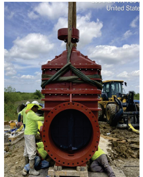
Seg B – Bolting Gate Valve to Pipe
