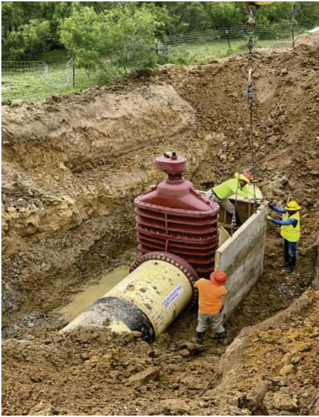
Seg A – Garney Builds Forms at STA. 477+48.82
