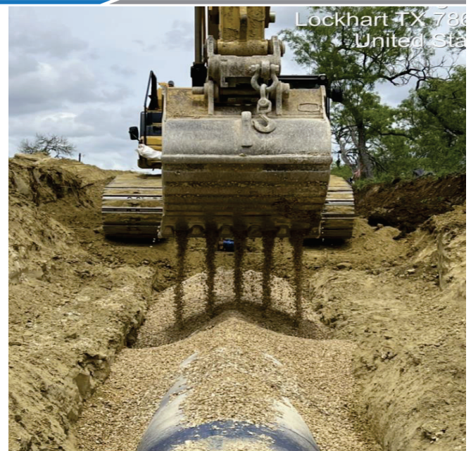
Seg D – Embedment Backfill
