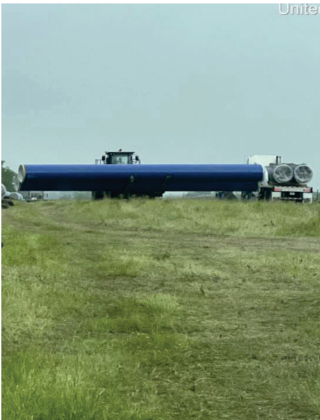
Seg D – Pipe Deliveries
