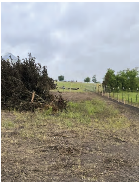
Seg E – Clearing Grubbing of Brush & Trees
