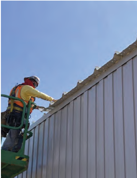
WTP – Electrical Building Roof Sheetting
