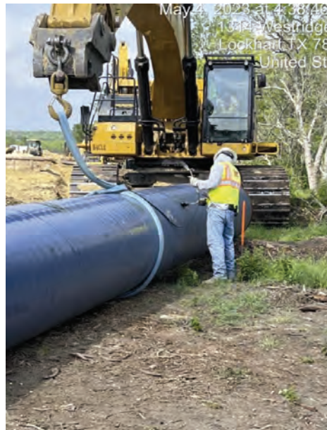
Seg D – Pipe Coating Repair
