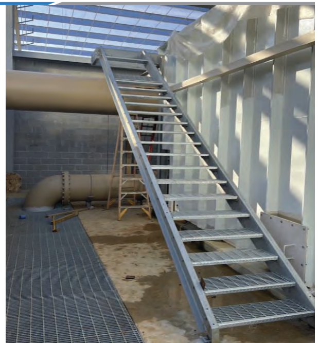
WTP – Stairs installed at Filter Complex
