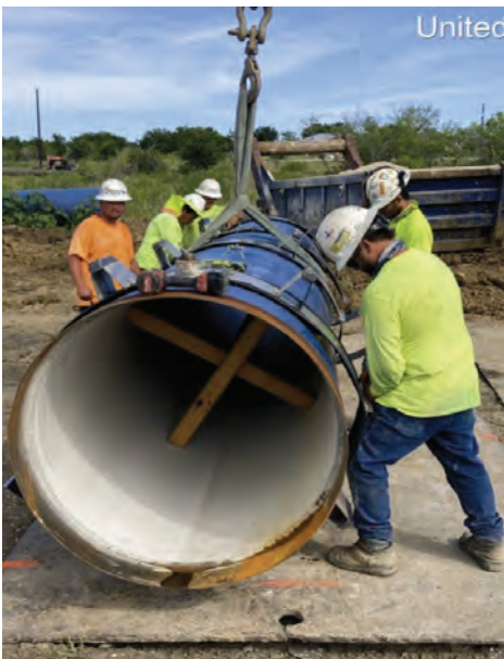
Seg B – Installing Pipe Spacers on Pipe
