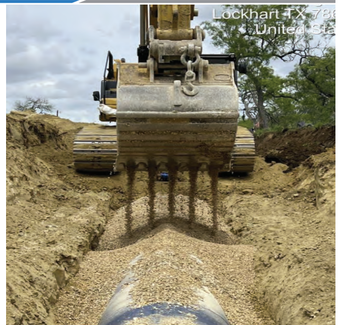
Seg D – Embedment Backfill
