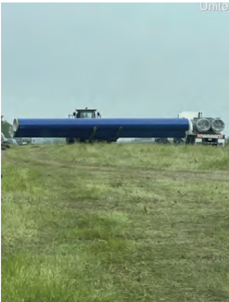
Seg D – Pipe Deliveries
