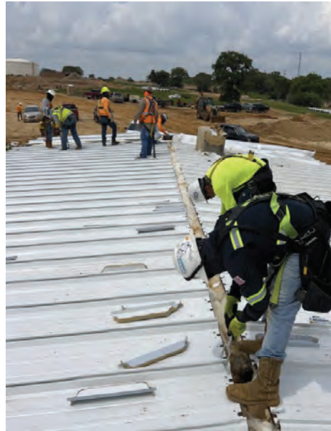
WTP – Electrical Building Installing Roof Sheetting
