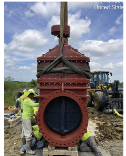
Seg B – Bolting Gate Valve to Pipe
