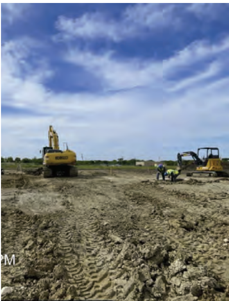
BPS – Subgrade Work for Concrete Paving
