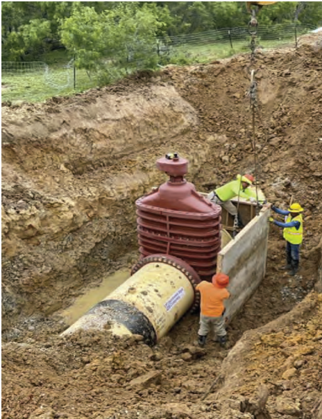
Seg A – Garney Builds Forms at STA. 477+48.82
