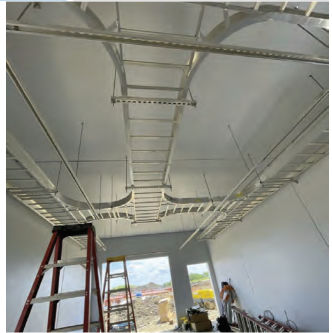
BPS – Hangers & Supports for Electrical Building
