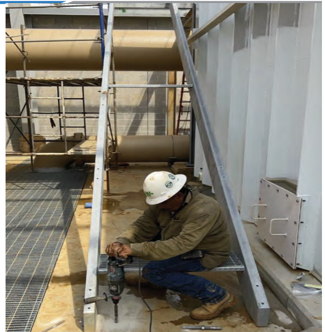
WTP – Installing Stairs at Filter Complex for Elevated Walkway
