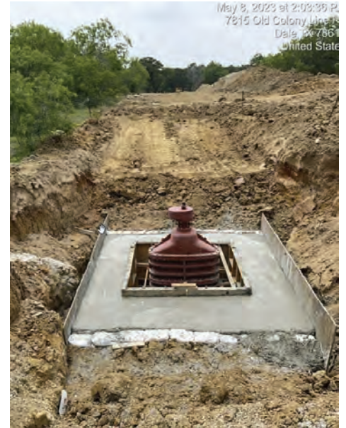
Seg A - Concrete around Valve for Manway
