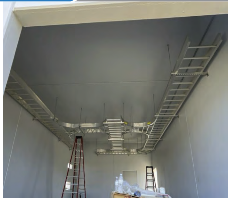
BPS – Cable Tray Install Inside Electrical Building
