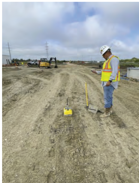
BPS – Testing Density on Paving Subgrade
