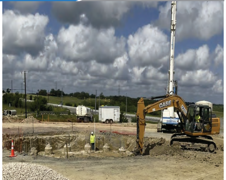
EST - Excavating Piers for Cap Placement
