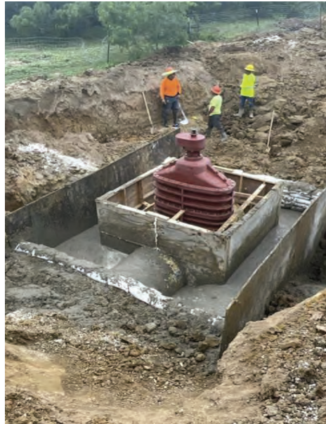
Seg A – Place Flow Fill for Valve Vault at STA. 477+48.82
