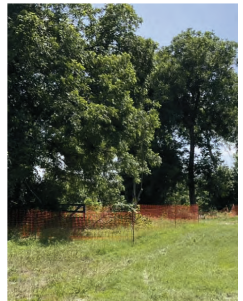
Seg E – Installed Tree Protection
