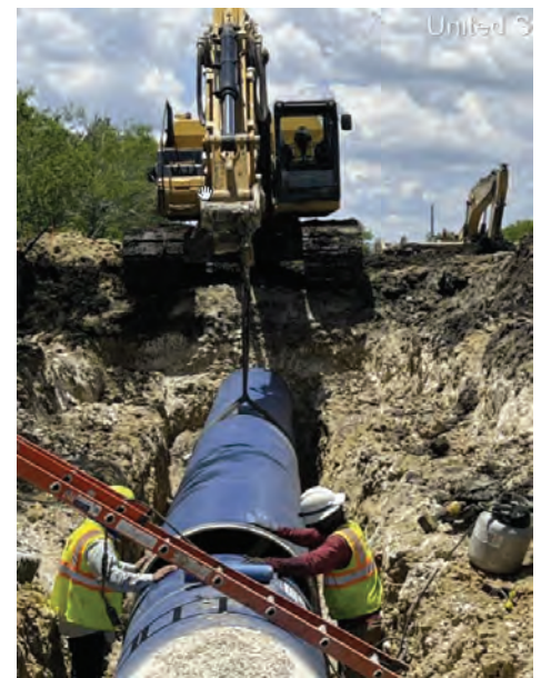
Seg D – Pipe Placement
