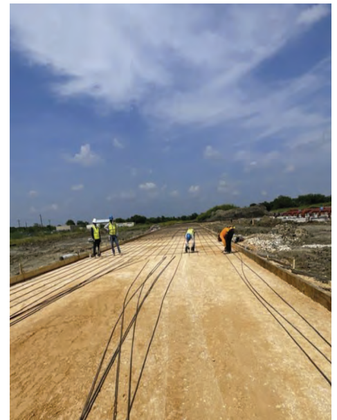
BPS – Road Paving Steel Reinforcement
