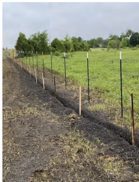
Seg E – Installing Stakes for Silt Fence
