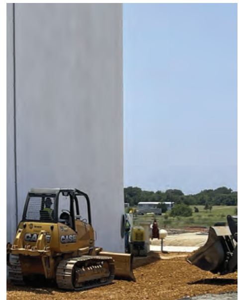
BPS – Base Material Placement Around GST
