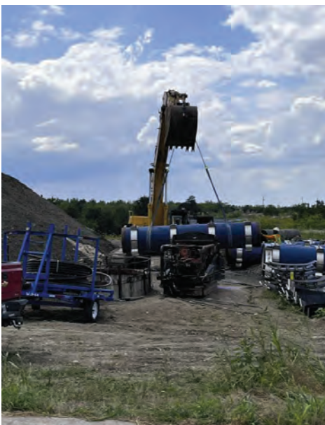
Seg B – Garney Preparing to set Pipe at SH130
