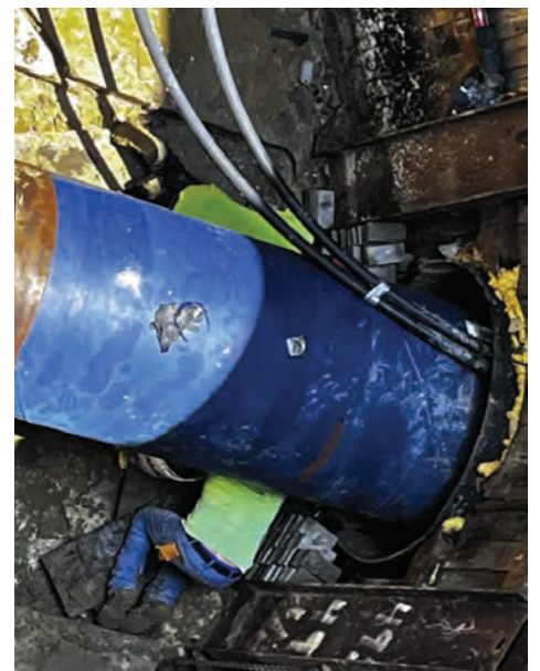
Seg B – Garney Constructing Bulkhead at SH130
