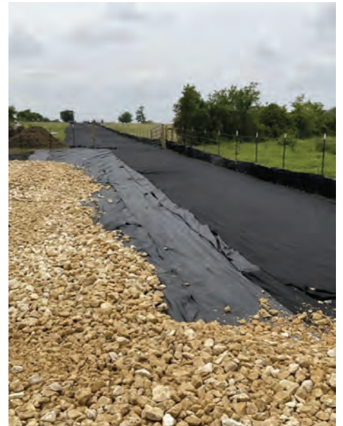
Seg E – Installing Gravel with Barrier
