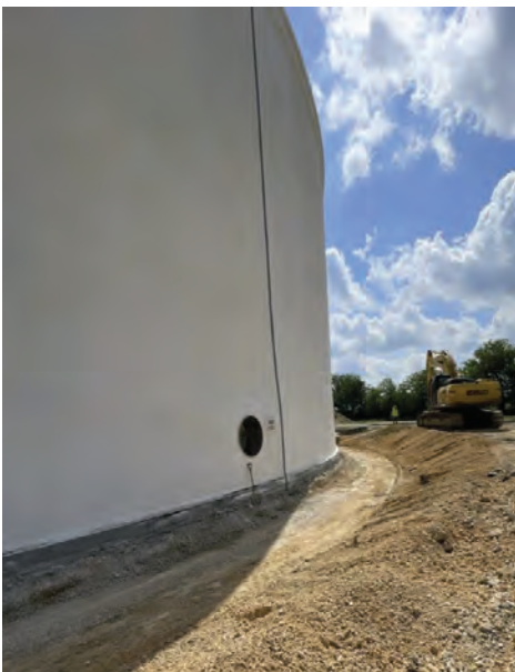
BPS – Excavation Around GST
