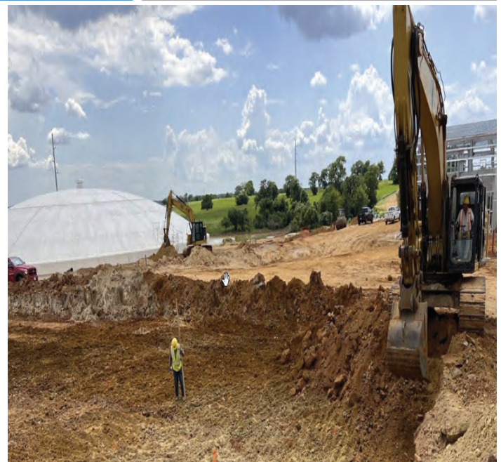
WTP – Grading Subgrade for Drying Beds
