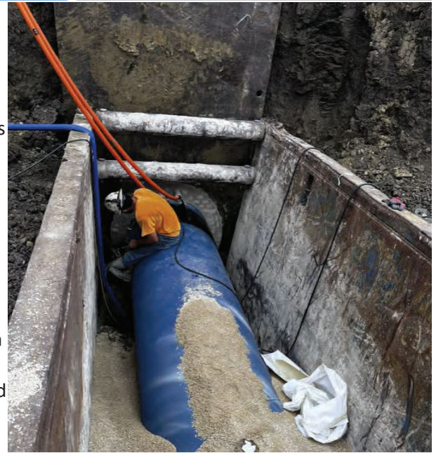
Segment B – Garney applying Canusa on pipe.
