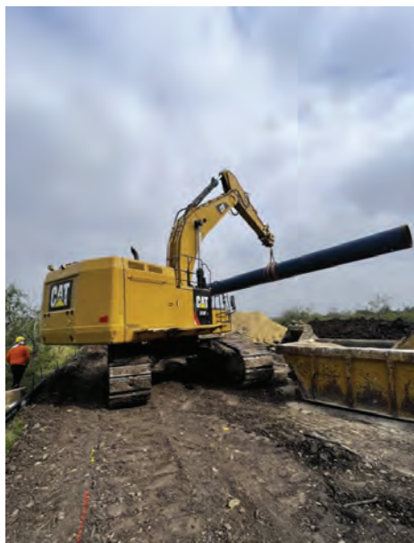
Seg B – Garney Crew placing Pipe at SH130
