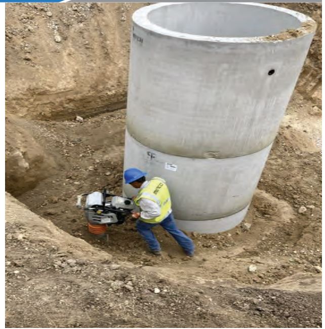
BPS – Backfill efforts around BOV manhole at STA 7+76
