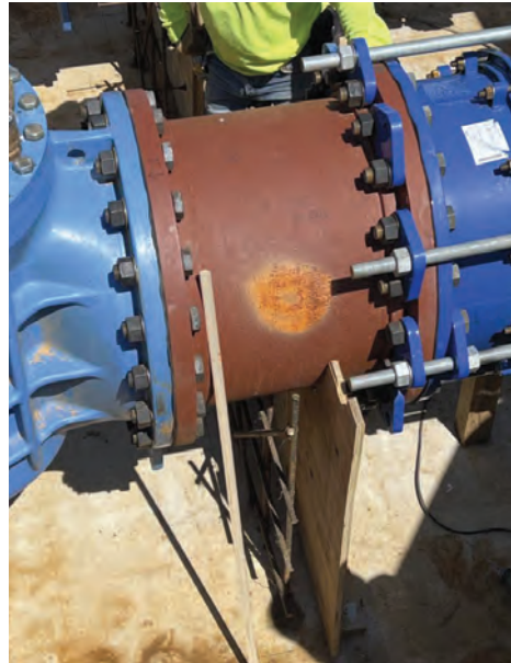
WTP – Rapid Mix Forming Concrete Saddle on 24” GW Pipe
