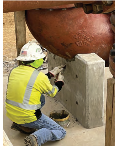
WTP – Rapid Mix Grout 24” GW Concrete Saddle Support 5
