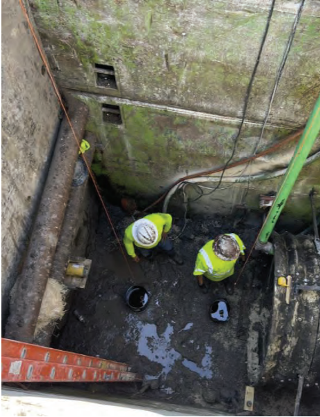
Seg D – Morrison Creek Tunnel
