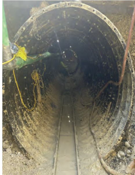
Seg D – Tunneling at FM 1339
