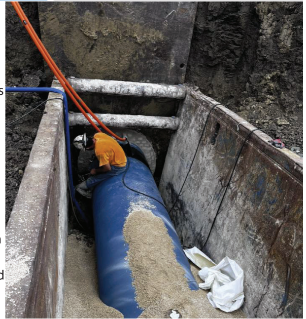
Segment B – Garney applying Canusa on pipe.
