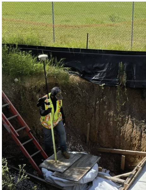
Seg E – Surveying for Elevation Connection at Plant
