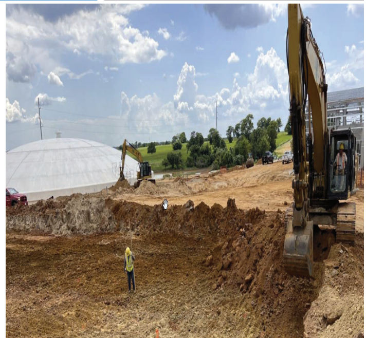
WTP – Grading Subgrade for Drying Beds
