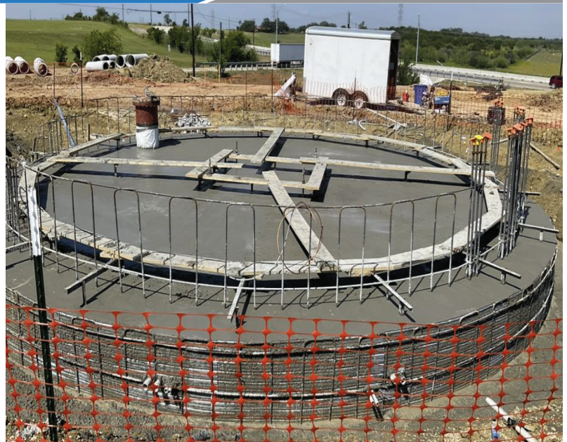
EST – Completed Cap Base
