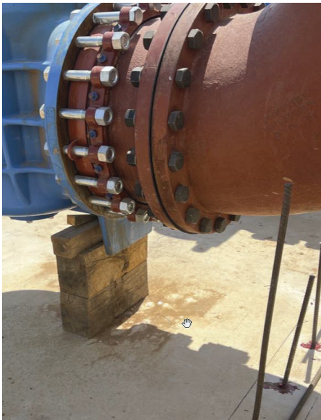
WTP – Rapid Mix Setting Dowels for 24” GW Concrete Pipe Supports
