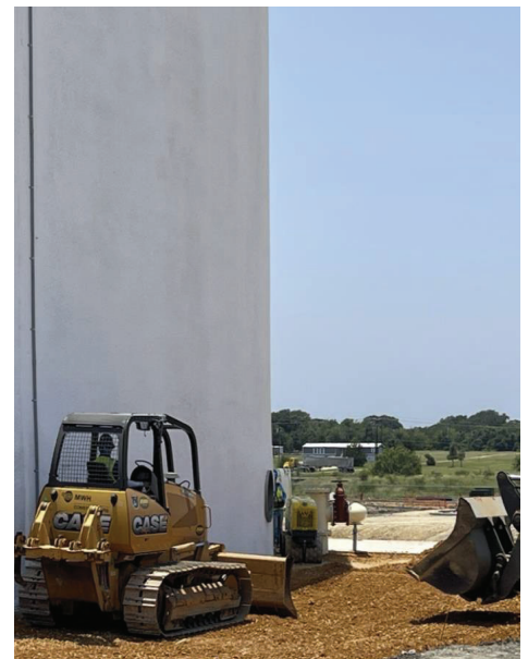
BPS – Base Material Placement Around GST
