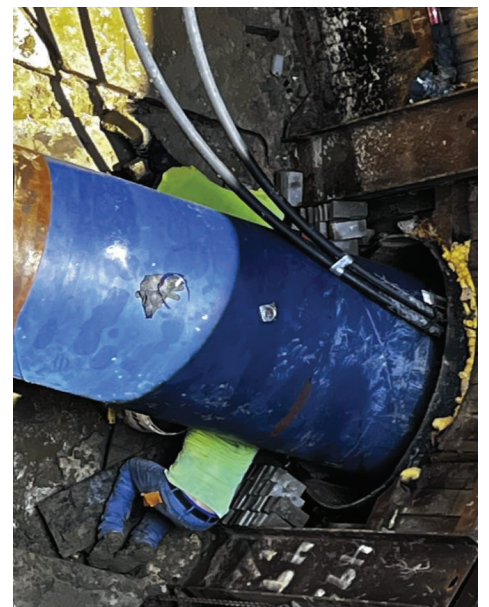
Seg B – Garney Constructing Bulkhead at SH130
