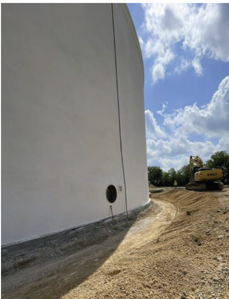
BPS – Excavation Around GST
