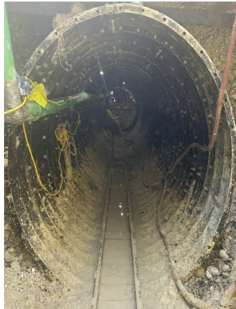
Seg D – Tunneling at FM 1339
