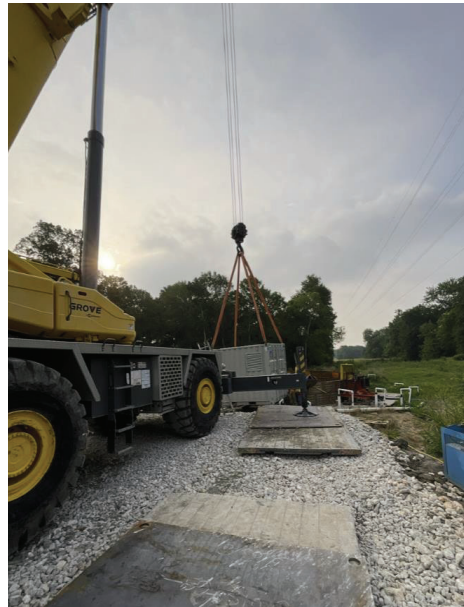
Seg A – Melcar Places Electric Panel Next to Bore Pit
