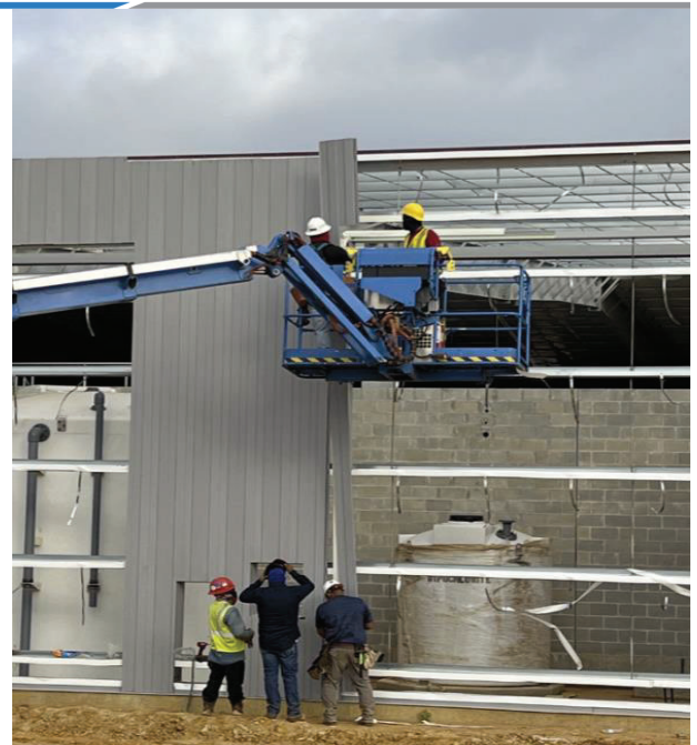
WTP – Filter Complex Wall Sheeting East Side
