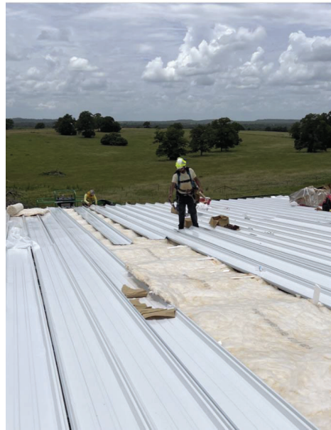
WTP – Filter Complex Roof Sheetting
