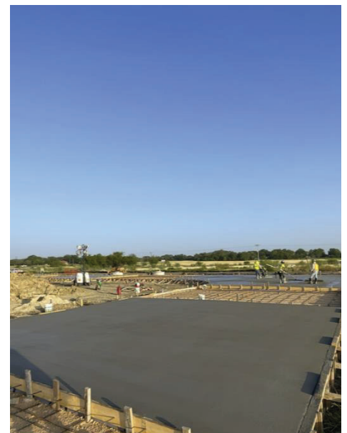
BPS – Access Road Concrete Placement
