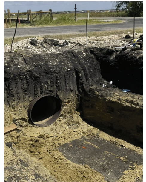
Seg E – Finished Installing Casing
