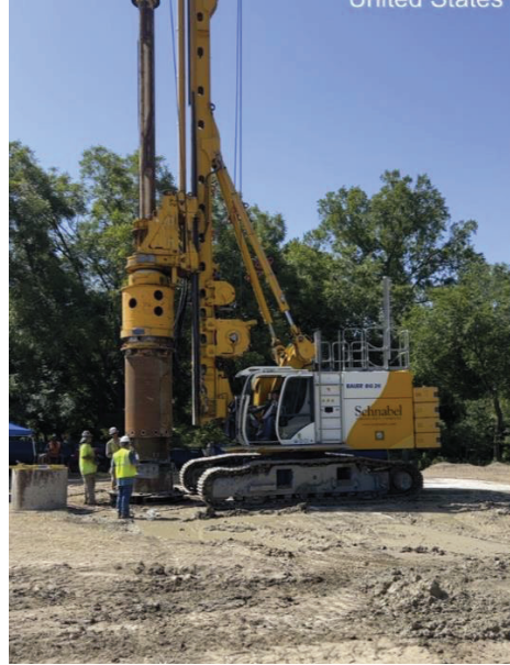
Seg D – Shaft #1 Casing
