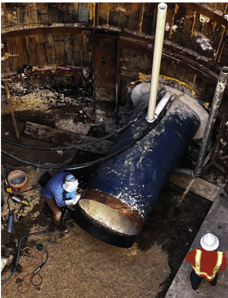
Seg B – Welder Attaching Butt Strap to Pipe at SH130
