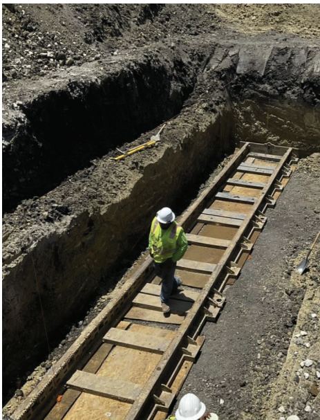
Seg E – Installing Base Track for Boring Machine
