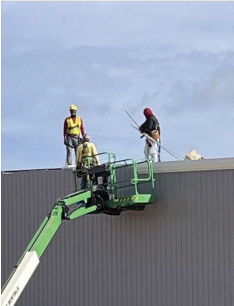
WTP – Filter Complex Installing Rake Trim
