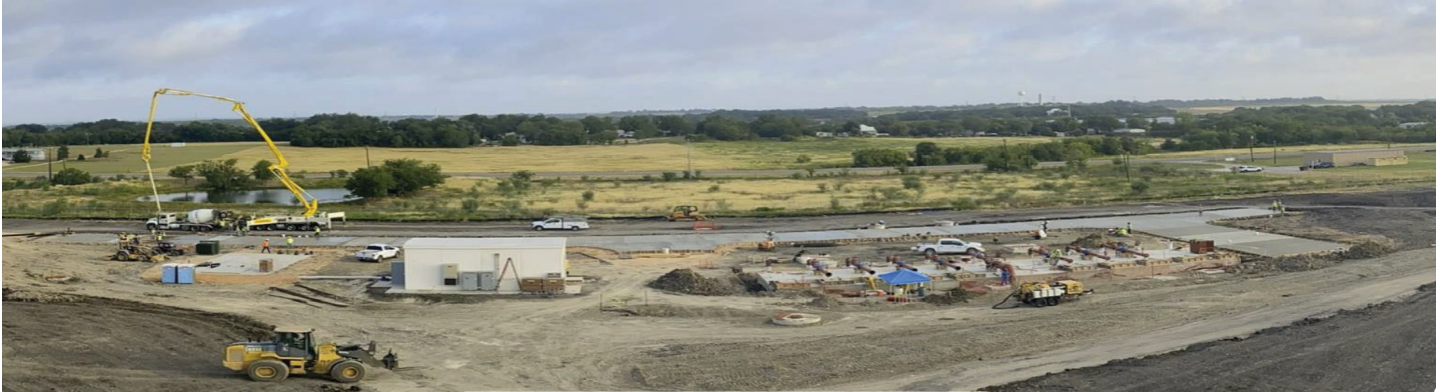
BPS – Placed Road Paving
