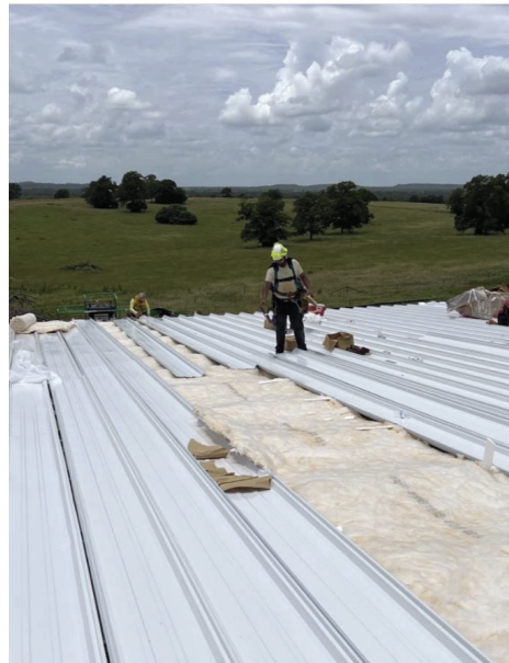
WTP – Filter Complex Roof Sheetting
