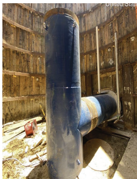
Seg B – Welded Butt Strap Complete at SH130
