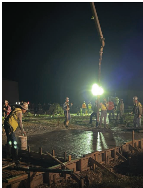
BPS – Access Road Concrete Placement
