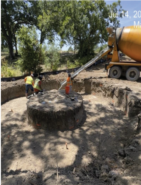
Seg D – Receiving Shaft Temp Pad Pour
