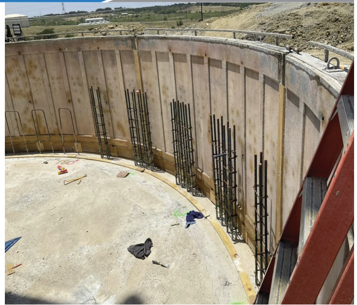
EST – Inside of First Lift of Upright
