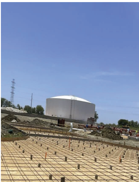
BPS – Access Road Expansion - Joints and Rebar
