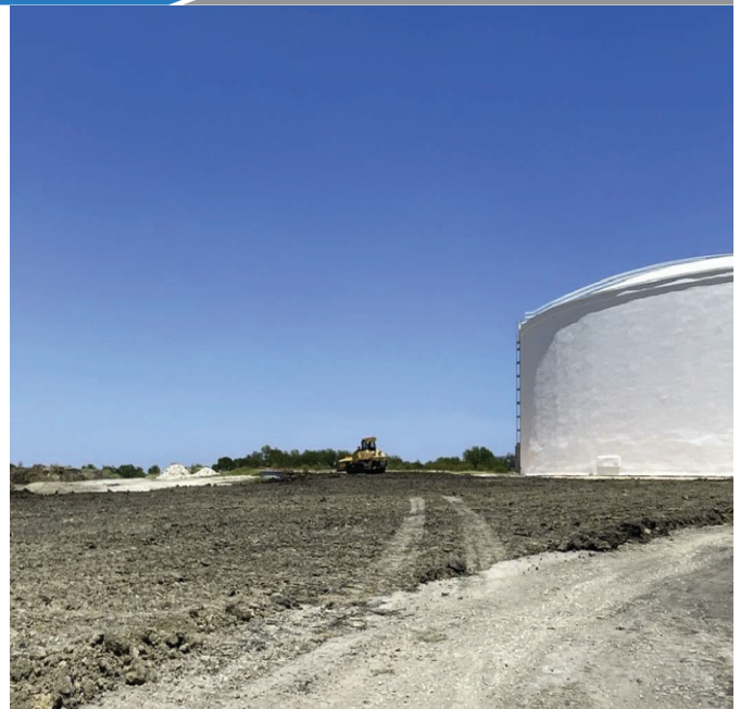
BPS – Grading West of Ground Storage Tank
