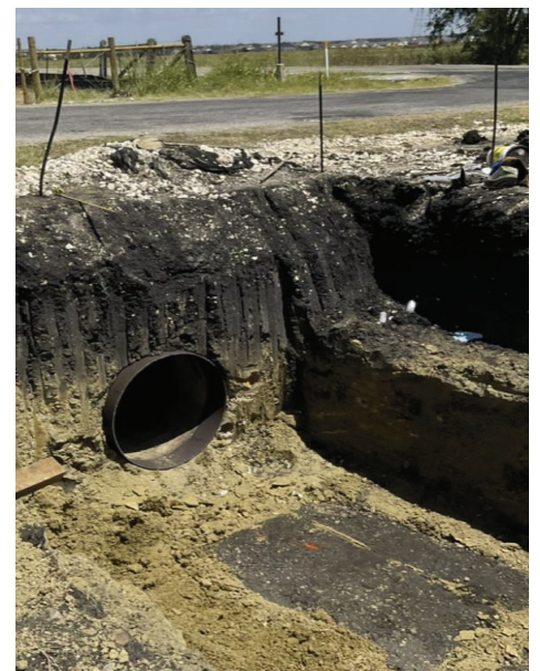
Seg E – Finished Installing Casing
