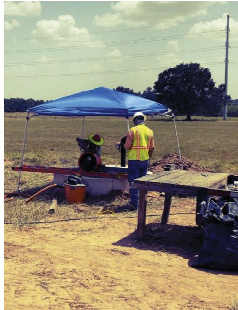
Seg A – Garney Installing an Air Relief Valve
