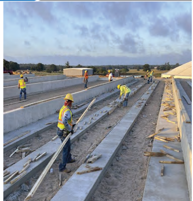
WTP – Drying Beds Removing Forms on Concrete Runners
