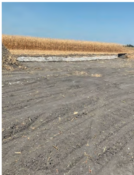
Seg E – Rock Berm and Silt Fence Installation
