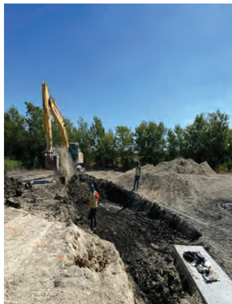
BPS –Detention Pond Spillway Excavation
