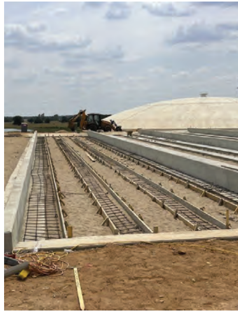
WTP – Drying Beds Setting Rebar for Concrete runners
