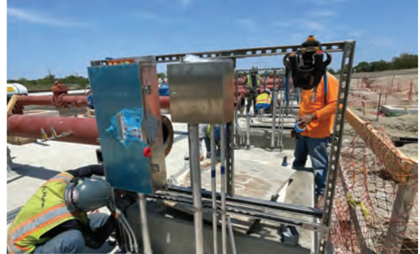
BPS – Electrical Rack for Pumps
