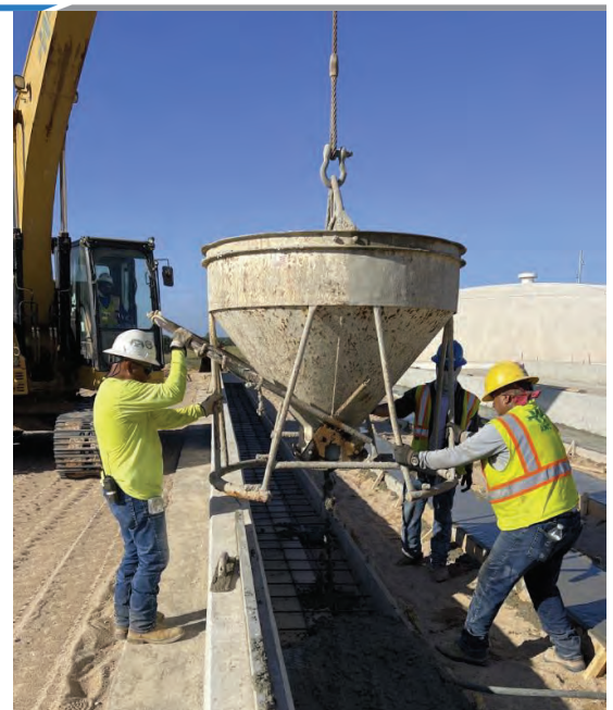
WTP – Drying Beds Placing Concrete on Runners
