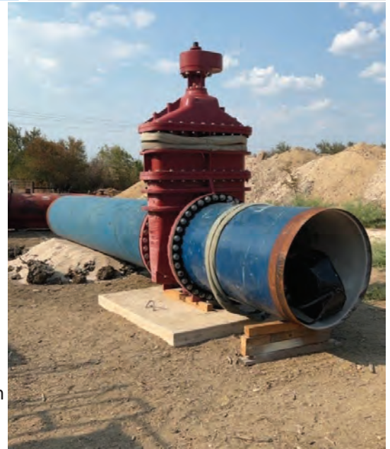
Segment B – Assembled Gate Valve
