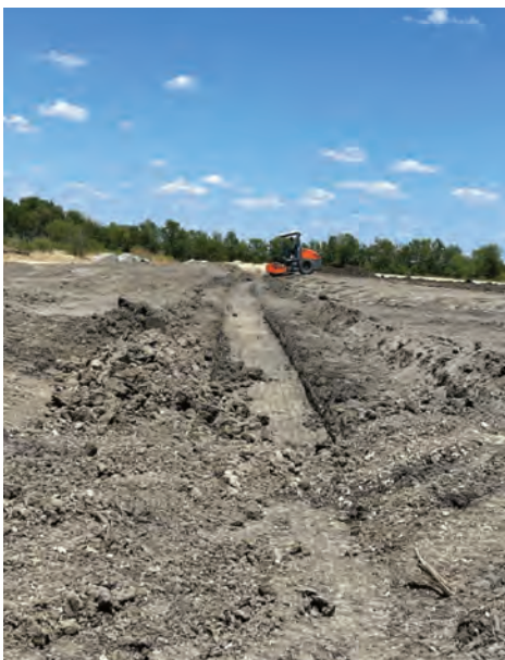
BPS – Swale 1 Grading Toward Detention Pond
