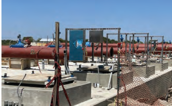
BPS – Electrical Rack for Pumps
