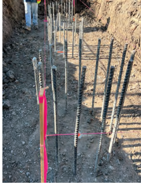
Seg D – Morrison Creek Pier Prep
