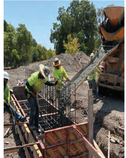
Seg D – Morrison Creek Bridge Abutment Pour
