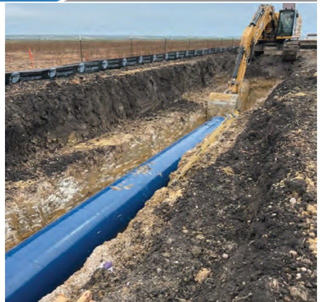
Seg D – Pipe Installation
