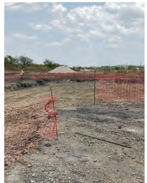
Seg E – Backfilling Vista Ridge Water Line Bore
