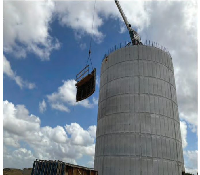
EST – Removing Internal Concrete Forms of 8th Lift
