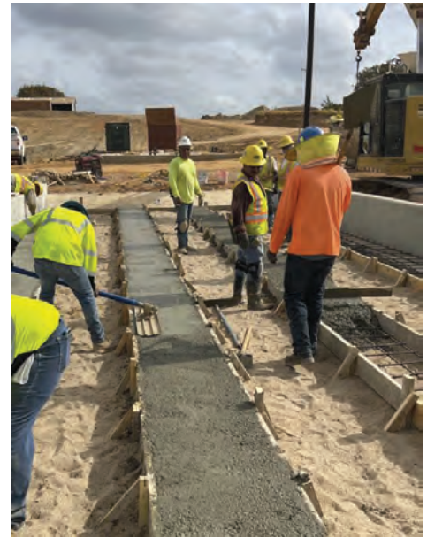
WTP – Drying Beds Concrete Placemen for Concrete Runners 5
