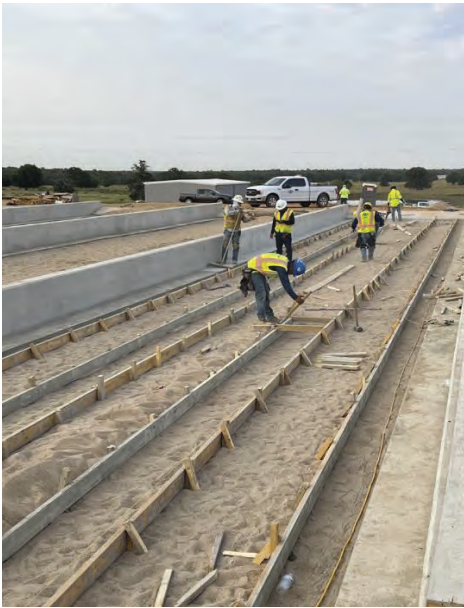
WTP – Drying Beds setting Forms for Concrete Runners
