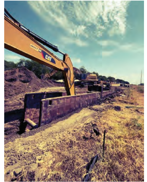
Seg A – Garney Placing Pipe East of Plum Creek
