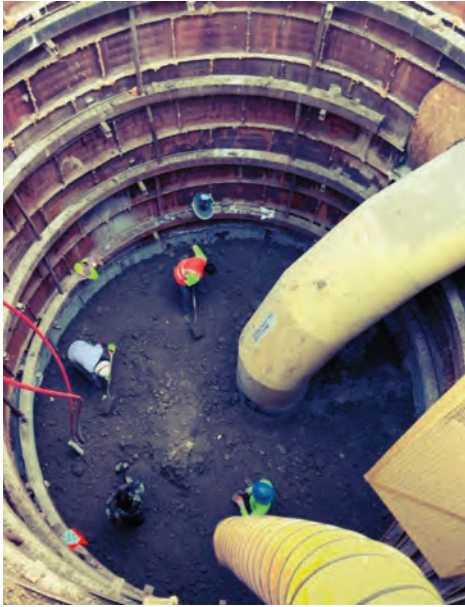
Seg A – Melcar Place Backfill in Receiving Pit
