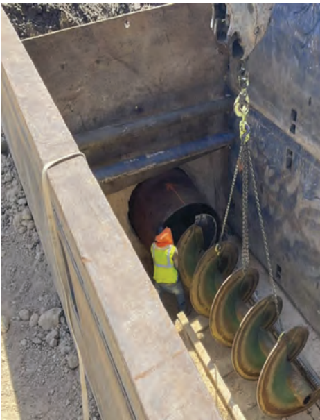
Seg E – Lowering Section of Drill Bit
