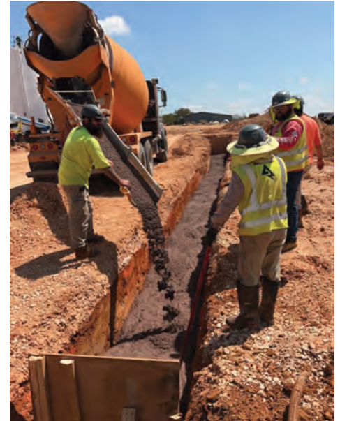
WTP – Lighting Duct Bank South of Lime System Concrete Placement 5
