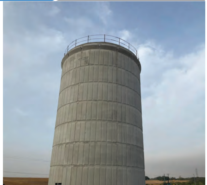
EST – Finished Top Portion of EST
