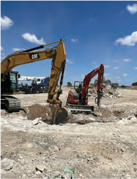
Seg D – Launch Shaft Excavation
