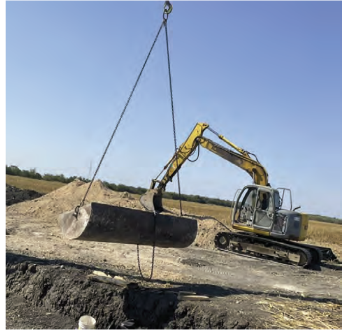
Seg E – Dumping Spoils from Bore 21
