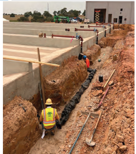
WTP – Drying Beds Installing 4’ Sludge Pipe
