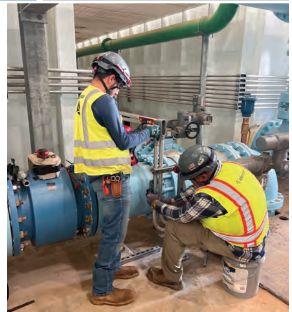
WTP – Filter Complex Rough-in Conduits
