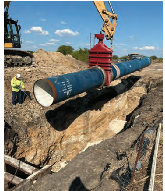
Segment B – Installing Gate Valve
