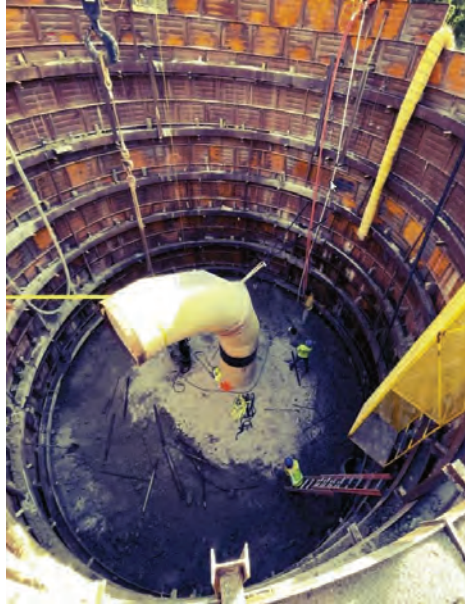
Seg A – Backfill at Plum Creek Receiving Pit
