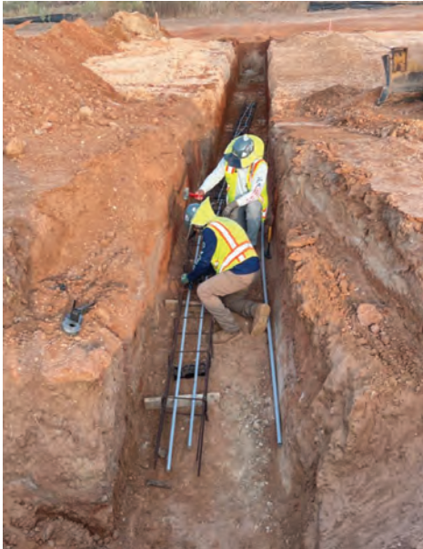
WTP – Installing Conduits for Lighting Duct Bank South Side of Lime System
