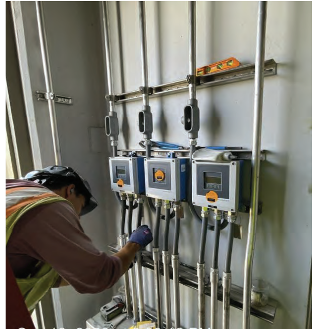
BPS – Seal Tight Install Inside Electrical Building
