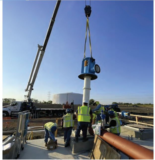
BPS – Pump Installation
