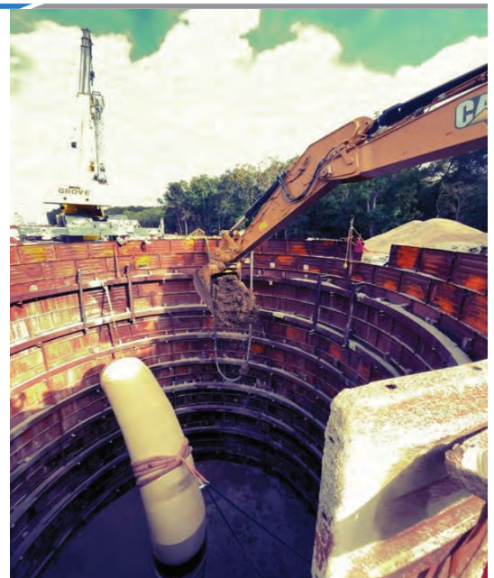
Seg A - Garney Places Backfill into Bore Pit
