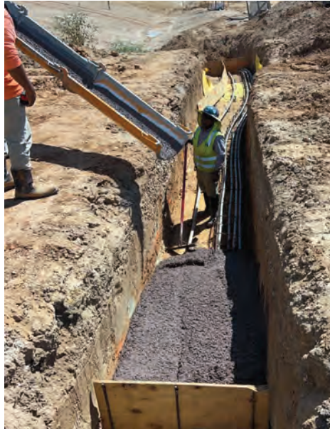
WTP – Duct Bank P3 Concrete Placement
