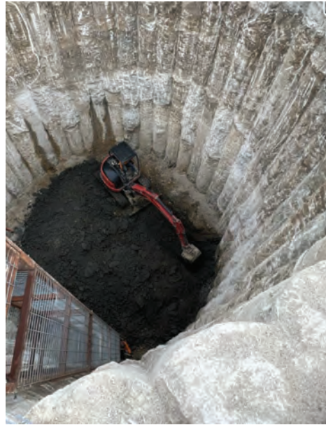
Seg D – Launch Shaft Excavation
