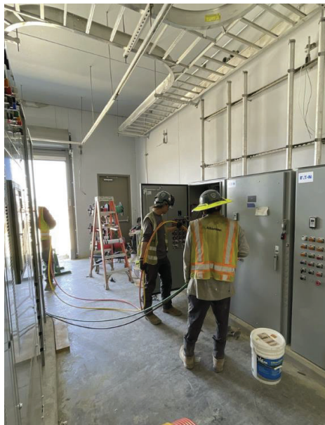
BPS - Wire Pull for Pump Soft Starts
