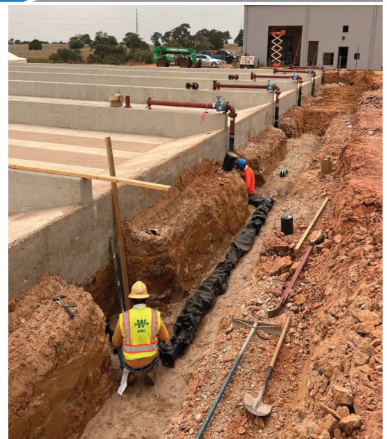
WTP – Drying Beds Installing 4' Sludge Pipe
