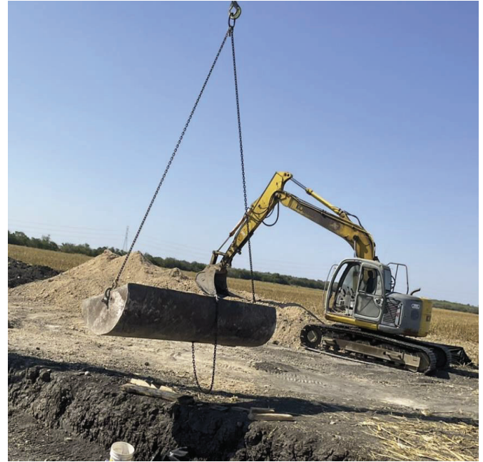
Seg E – Dumping Spoils from Bore 21
