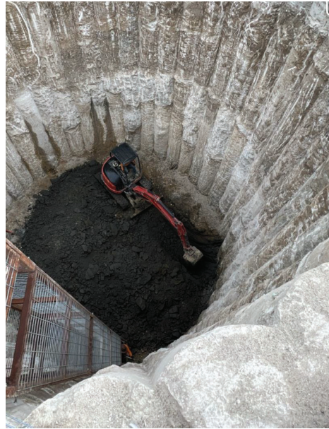
Seg D – Launch Shaft Excavation
