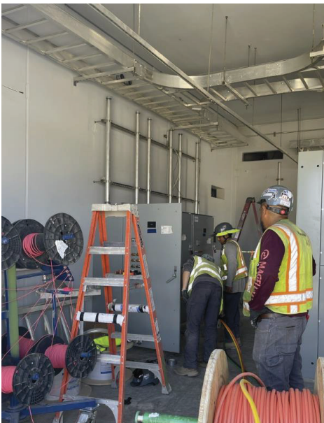
BPS – Wire Pull for Pump Soft Starts
