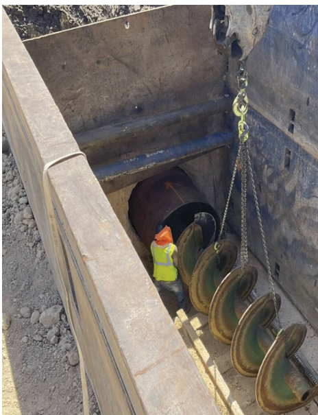
Seg E – Lowering Section of Drill Bit
