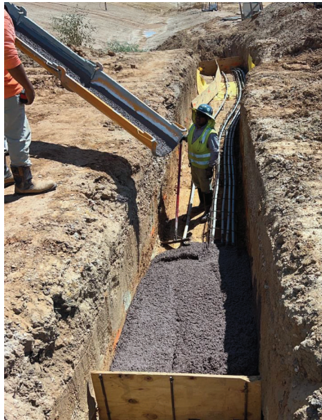
WTP – Duct Bank P3 Concrete Placement
