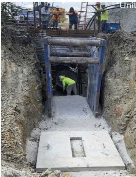
Seg B – Installed Base for Gate Valve
