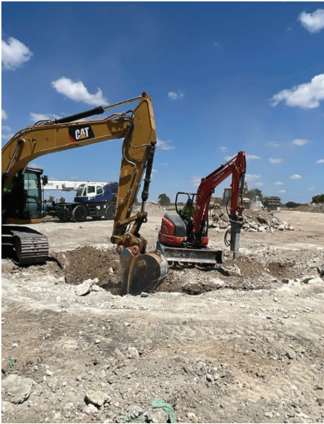
Seg D – Launch Shaft Excavation
