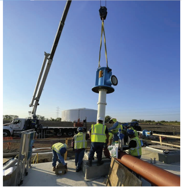
BPS – Pump Installation
