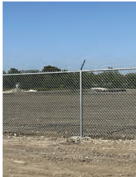
BPS – Barbed Wire Installed on Security Fence
