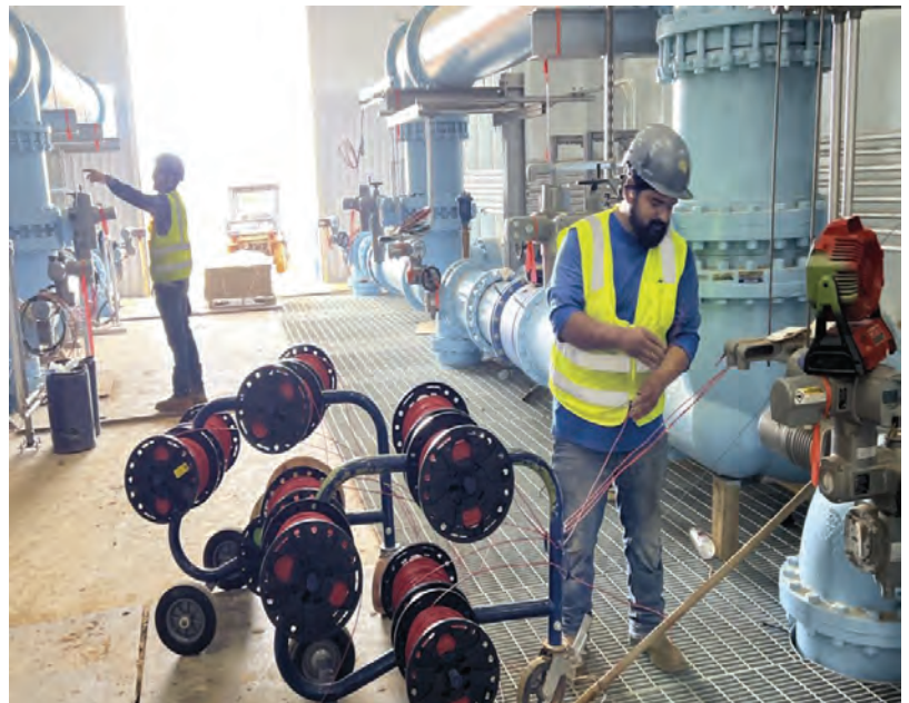
WTP – Wire Pulling at Filter Complex
