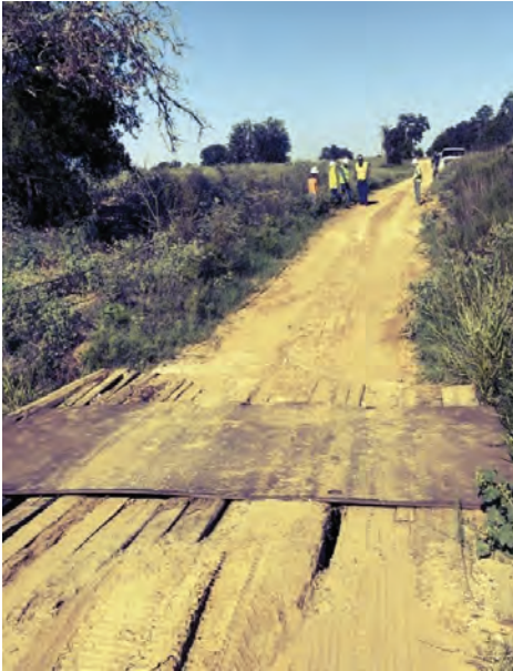
Seg A – Work Begins on Low Water Crossing at Rifle Road
