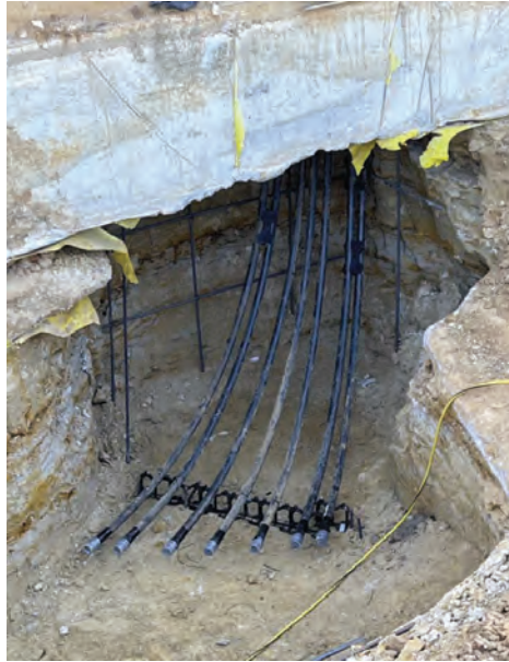
WTP – Filter Complex Rough-in Conduit Risers Under Slab in Electrical Room
