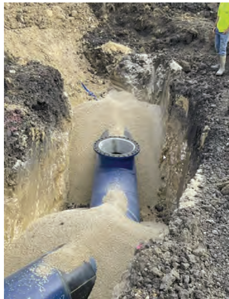
Seg E – Installing Gravel to Hold Concrete
