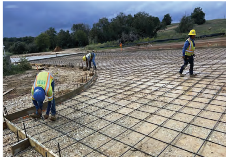
WTP – Installing Rebar for Driveway
