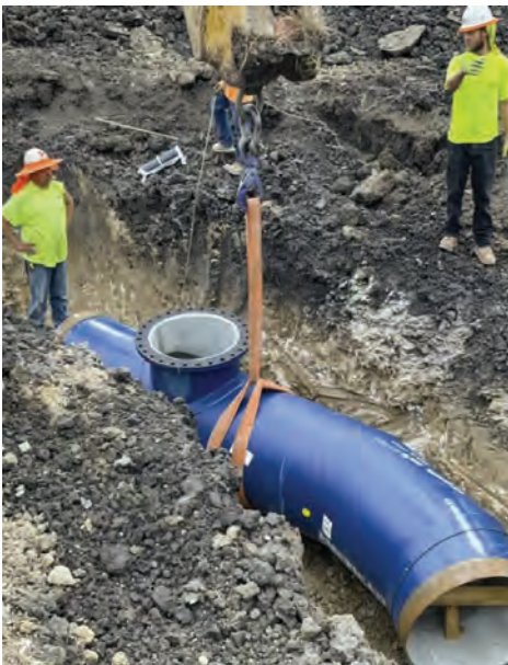
Seg E – Laid 45 Degree Manway Pipe
