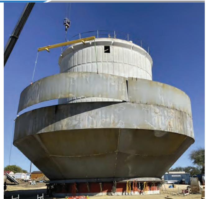
EST – Adding 4 th Sheet to Shell
