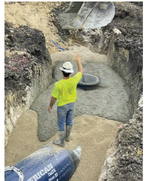
Seg E – Pouring Concrete Around Manway
