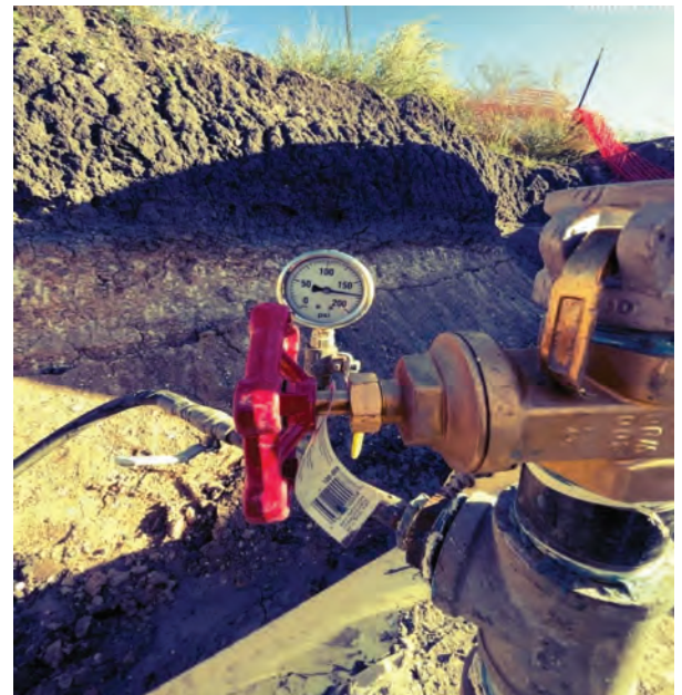
Seg A - Garney Test of 42" Line Passes
