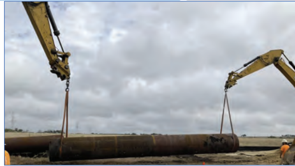
Seg E – Moving and Lowering First Casing
