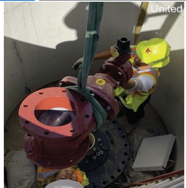
Seg D – Placing of Air Check Valve
