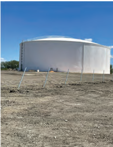
BPS – Security Fence Posts Installed
