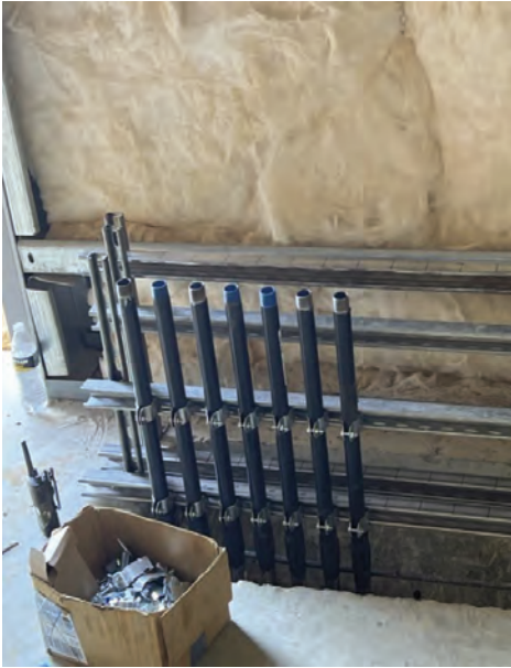
WTP – Filter Complex Rough-In Conduit Risers Under Slab
