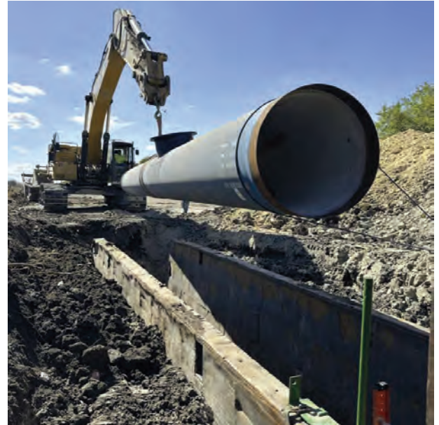
Segment B – Installing Pipe MK#1081
