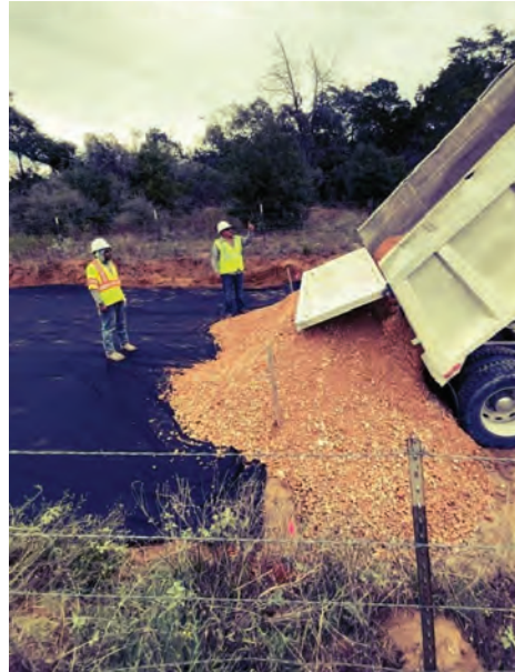
Seg A – J7 Works on Low Water Crossing at Rifle Road
