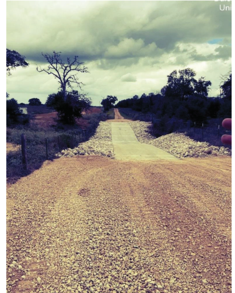
Seg A – Rifle Road Low Water Crossing Complete
