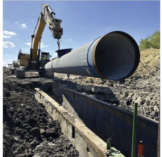
Segment B – Installing Pipe MK#1081
