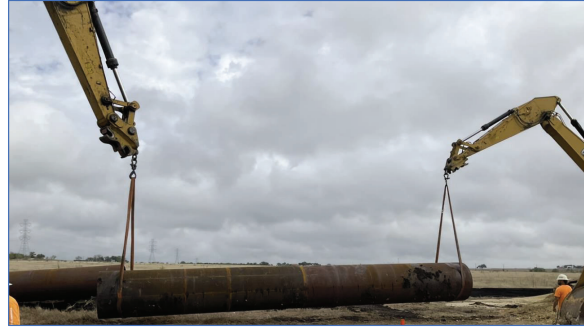
Seg E – Moving and Lowering First Casing
