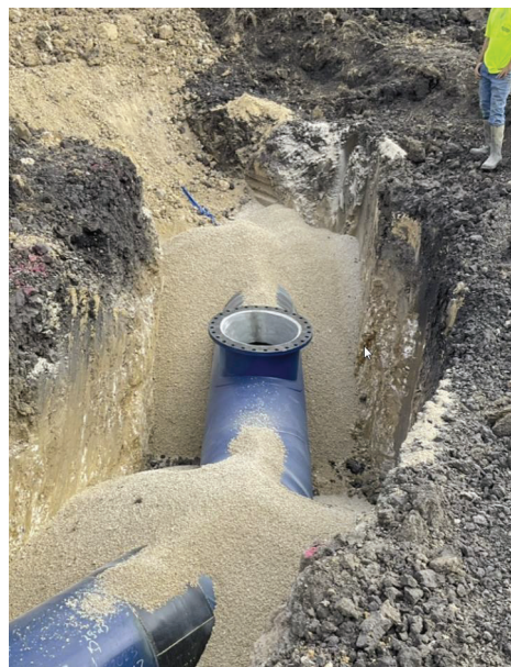
Seg E – Installing Gravel to Hold Concrete
