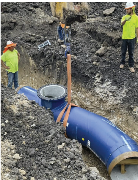
Seg E – Laid 45 Degree Manway Pipe
