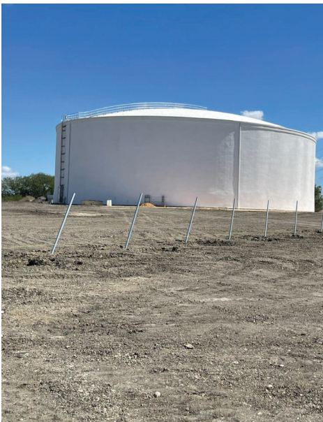
BPS – Security Fence Posts Installed
