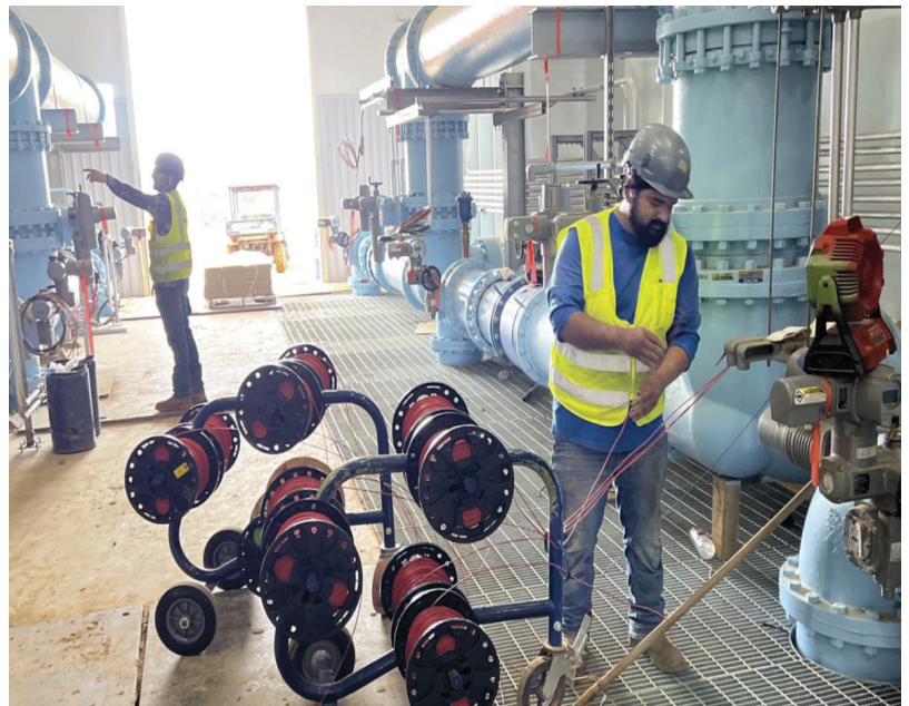
WTP – Wire Pulling at Filter Complex
