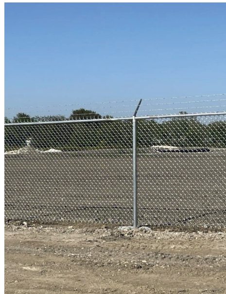
BPS – Barbed Wire Installed on Security Fence
