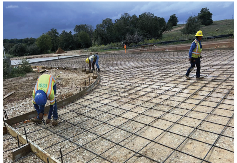
WTP – Installing Rebar for Driveway
