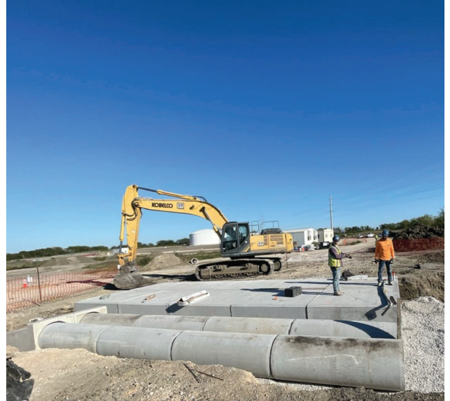
BPS – Drainage Work for Booster Site Access Road
