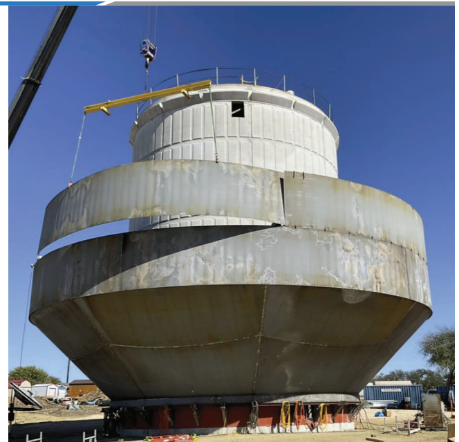
EST – Adding 4 th Sheet to Shell
