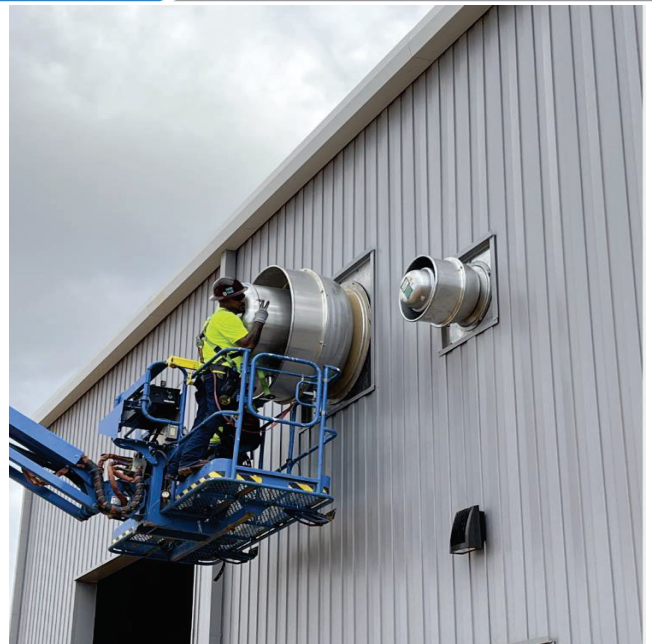
WTP – Installation of Exhaust Fan at Filter Complex
