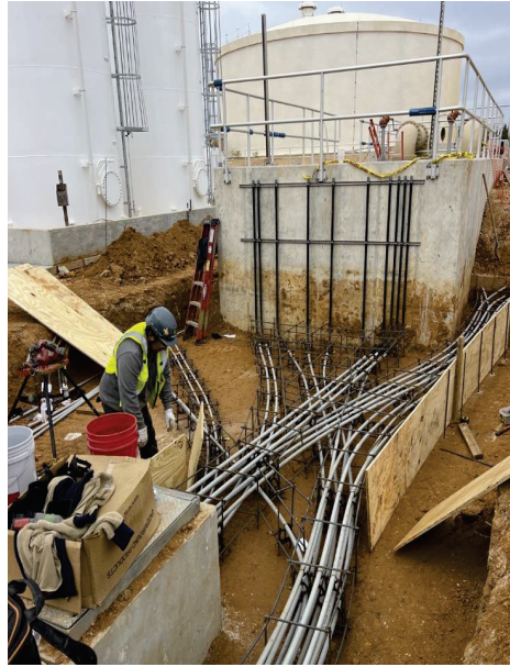
WTP – Setting Conduits in Trench for Duct Bank T-T
