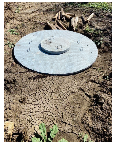
Seg B – Permanent Lid Placed at STA 359+94
