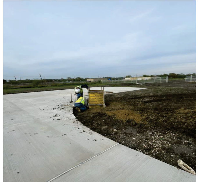
BPS – Sonotube for Light Pole Pier
