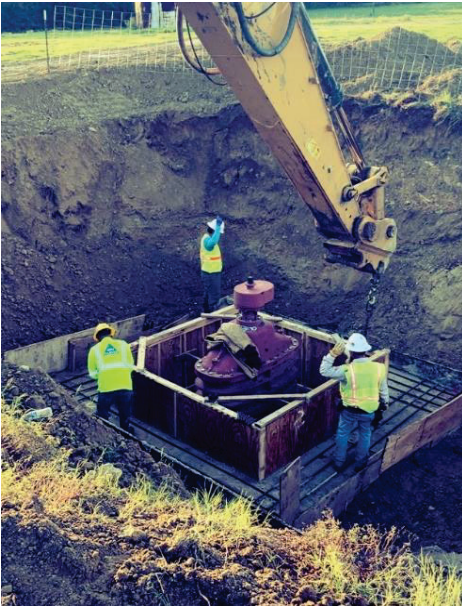
Seg A – Rebar Install for Vault Box Pad
