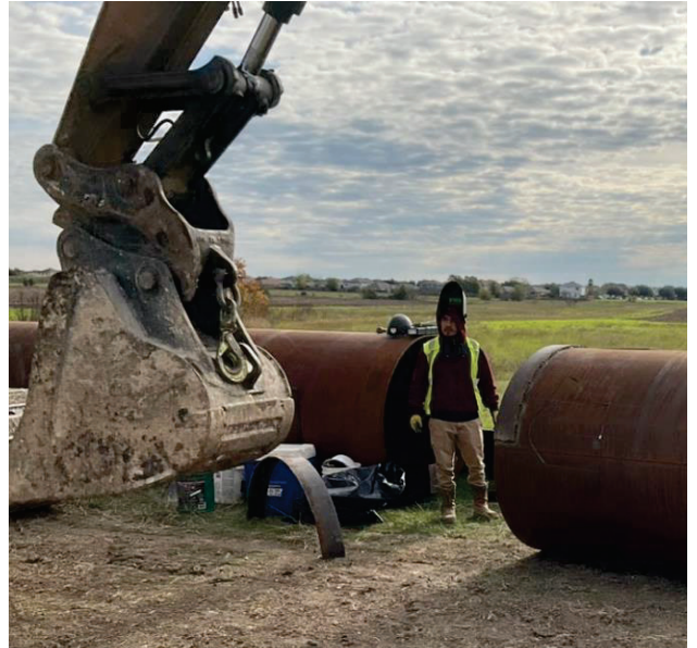
Seg E – Preparing Casing for Bore
