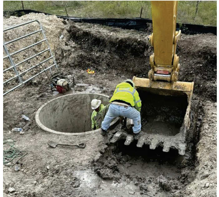
Segment B – Removing Mud from Pipe
