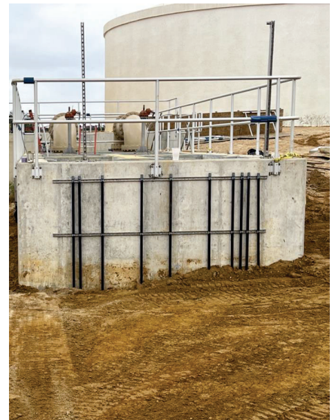
WTP – Trench Backfill at Duct Bank T-T
