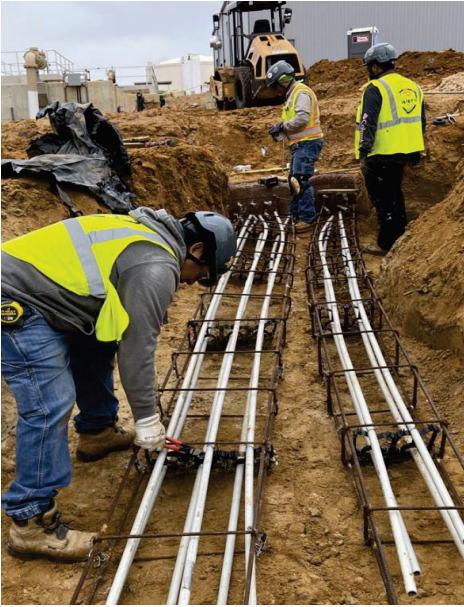
WTP – Setting Conduits in Trench for Duct Bank ZZ & YY
