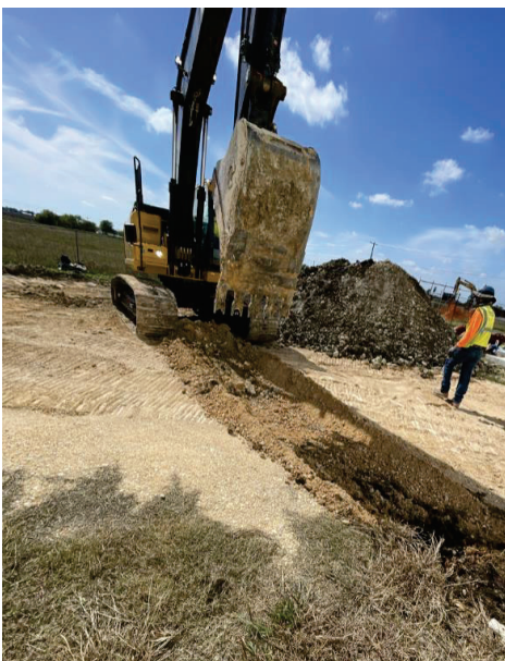
BPS – Excavation for Yard Pipe Install
