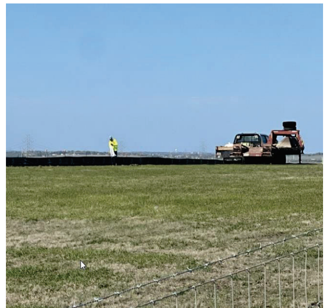
Seg D – Silt Fence Placement
