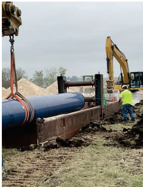
Seg E – Lowering Pipe Into Ditch
