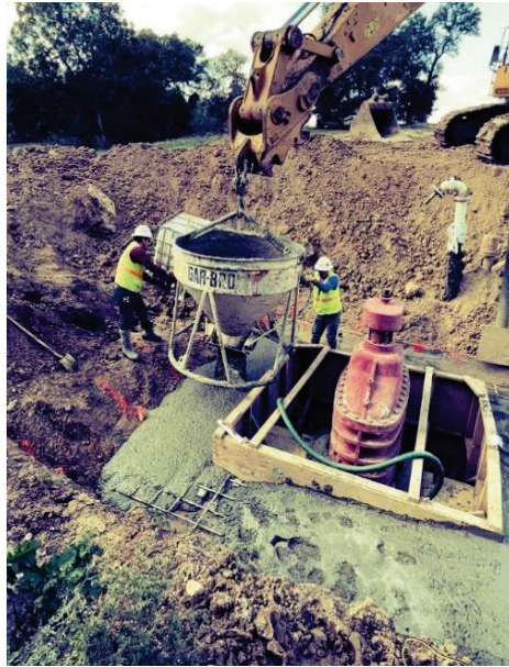
Seg A – Concrete Placement for Vault Box
