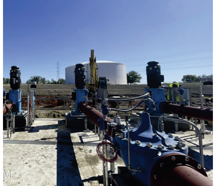
BPS – Installing Pump Station Motors
