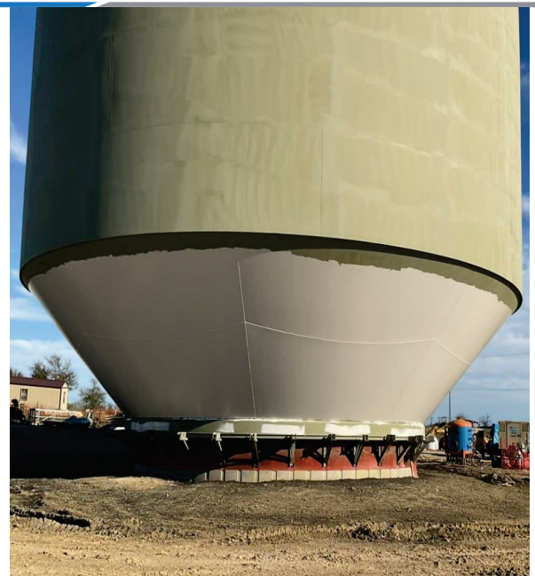
EST – First Coat of Paint
