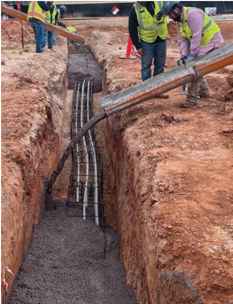
WTP – Duct Bank K-K Concrete Placement
