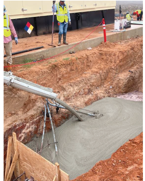
WTP – Duct Bank M-M Flow Fill in Trench
