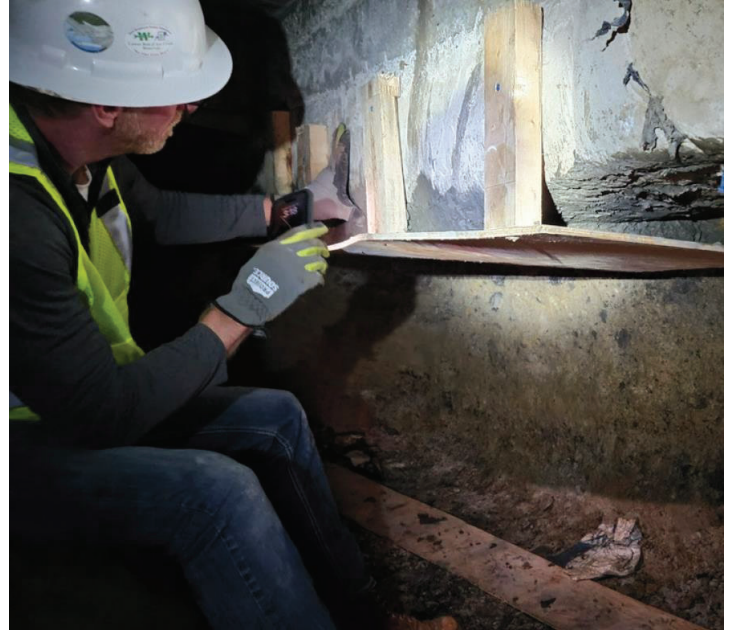
BPS – Under slab Beam Repair
