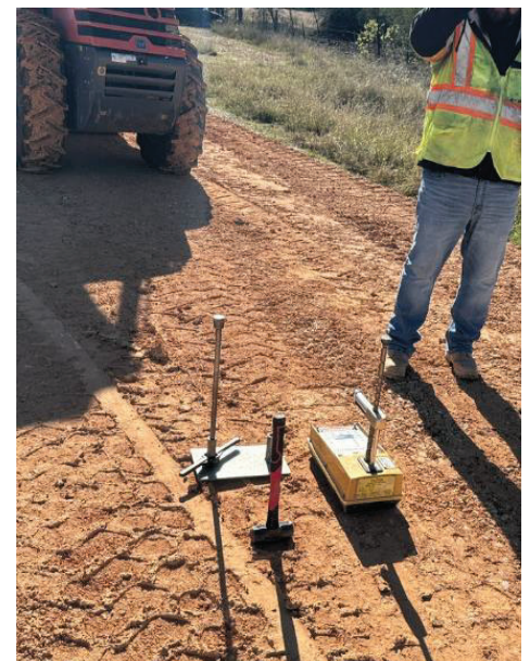
BPS – Density Test for Base Road
