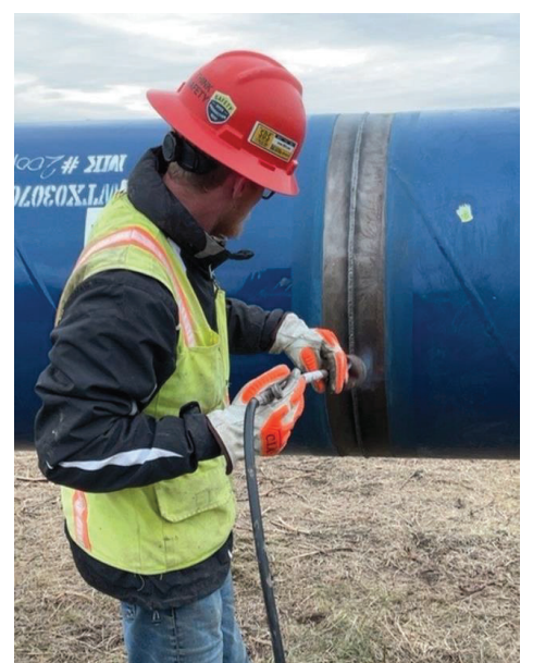
Seg E – Preparing Pipe for Epoxy
