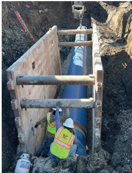
Seg D – Pipe Placement
