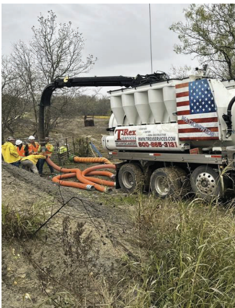
Seg B – Vacuuming Debris from SH-130 Tunnel
