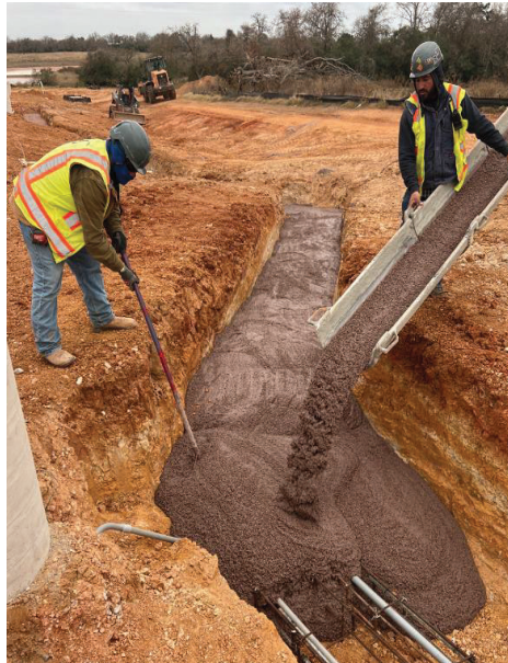
WTP – Duct Bank Concrete Placement
