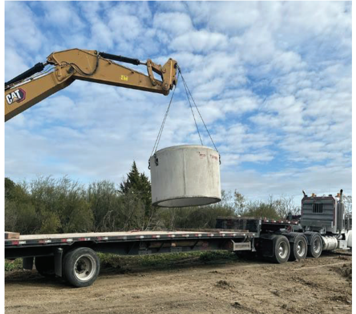
Segment B – Offloading Precast Off of Railroad Street
