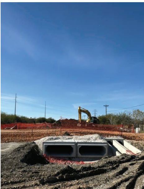
BPS – Installing Base Material for Access Road
