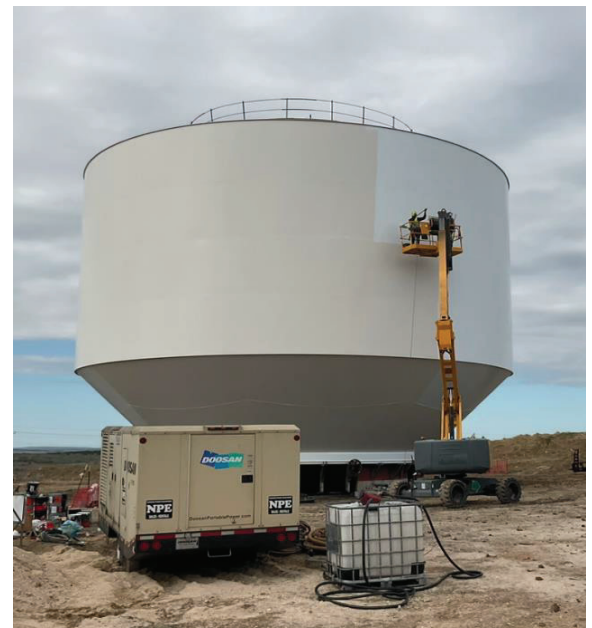
EST – Rolling on Final Coat of Paint
