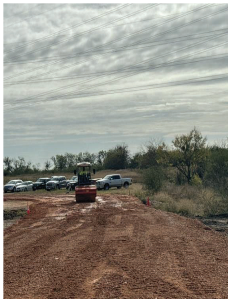
BPS – Road Base Install for Access Road
