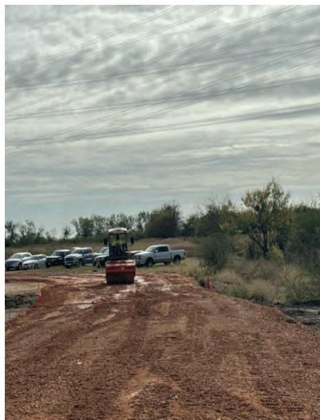
BPS – Road Base Install for Access Road
