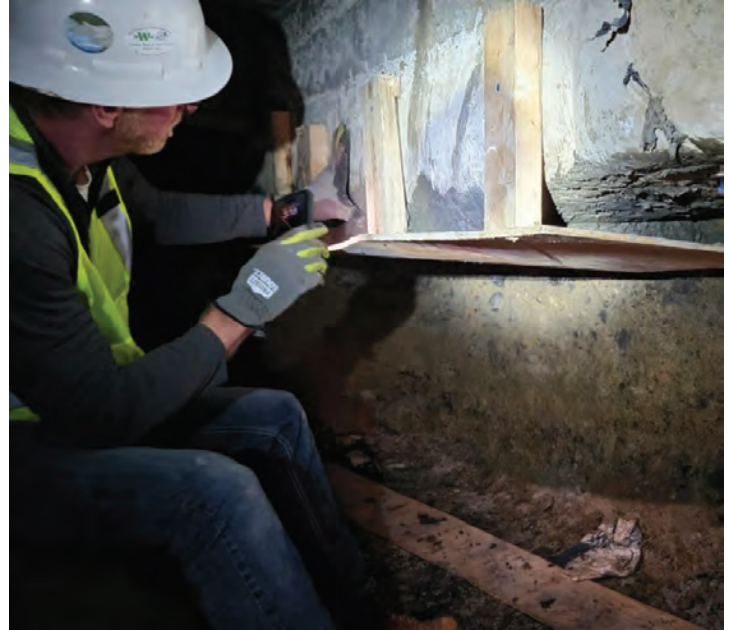
BPS – Under slab Beam Repair
