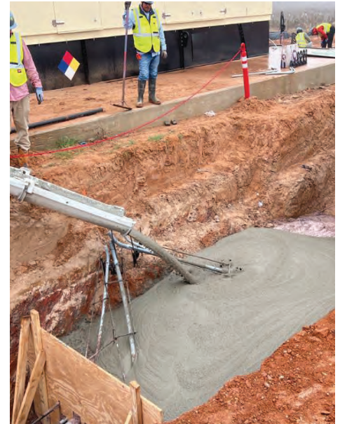
WTP – Duct Bank M-M Flow Fill in Trench
