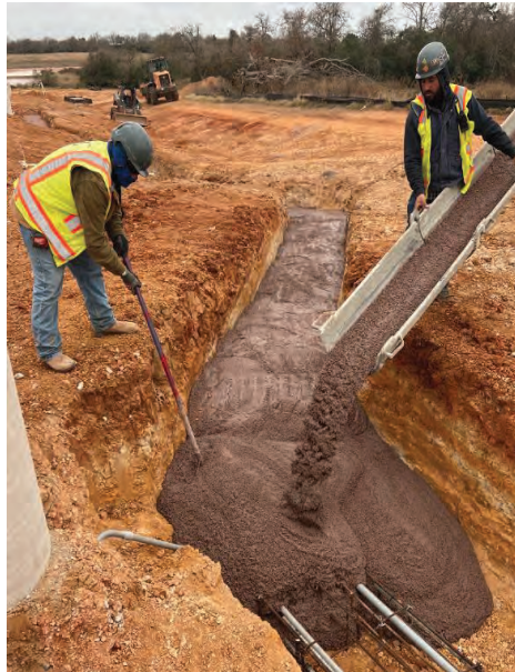
WTP – Duct Bank Concrete Placement
