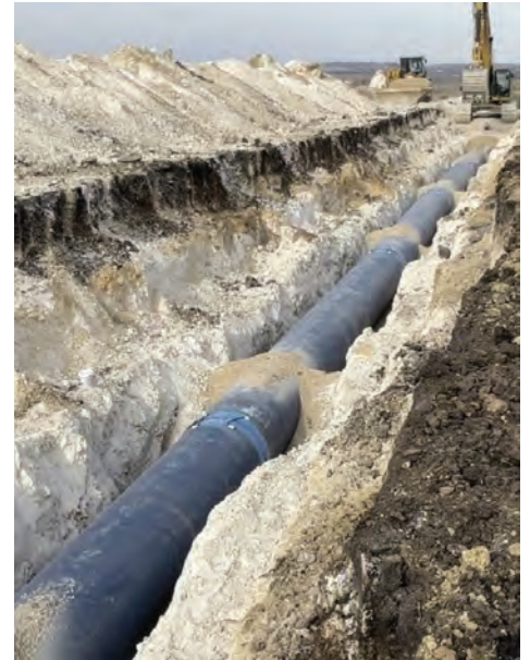
Seg D – Pipe Installation
