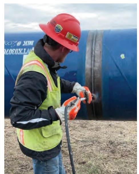
Seg E – Preparing Pipe for Epoxy
