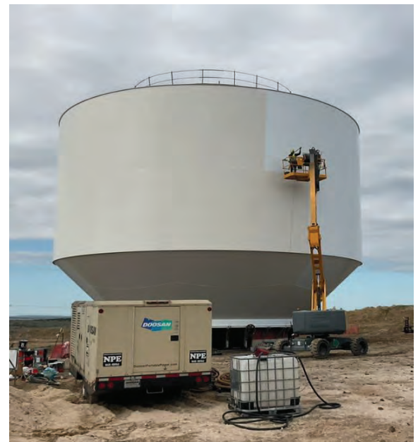
EST – Rolling on Final Coat of Paint
